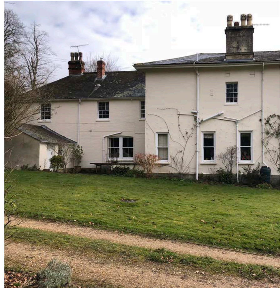
West side of dwelling the oil tank proposed on the extreme left side of the photograph.
