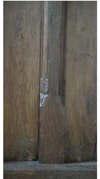
Detail of chamfered stops on screen panelling in the Great Hall.
