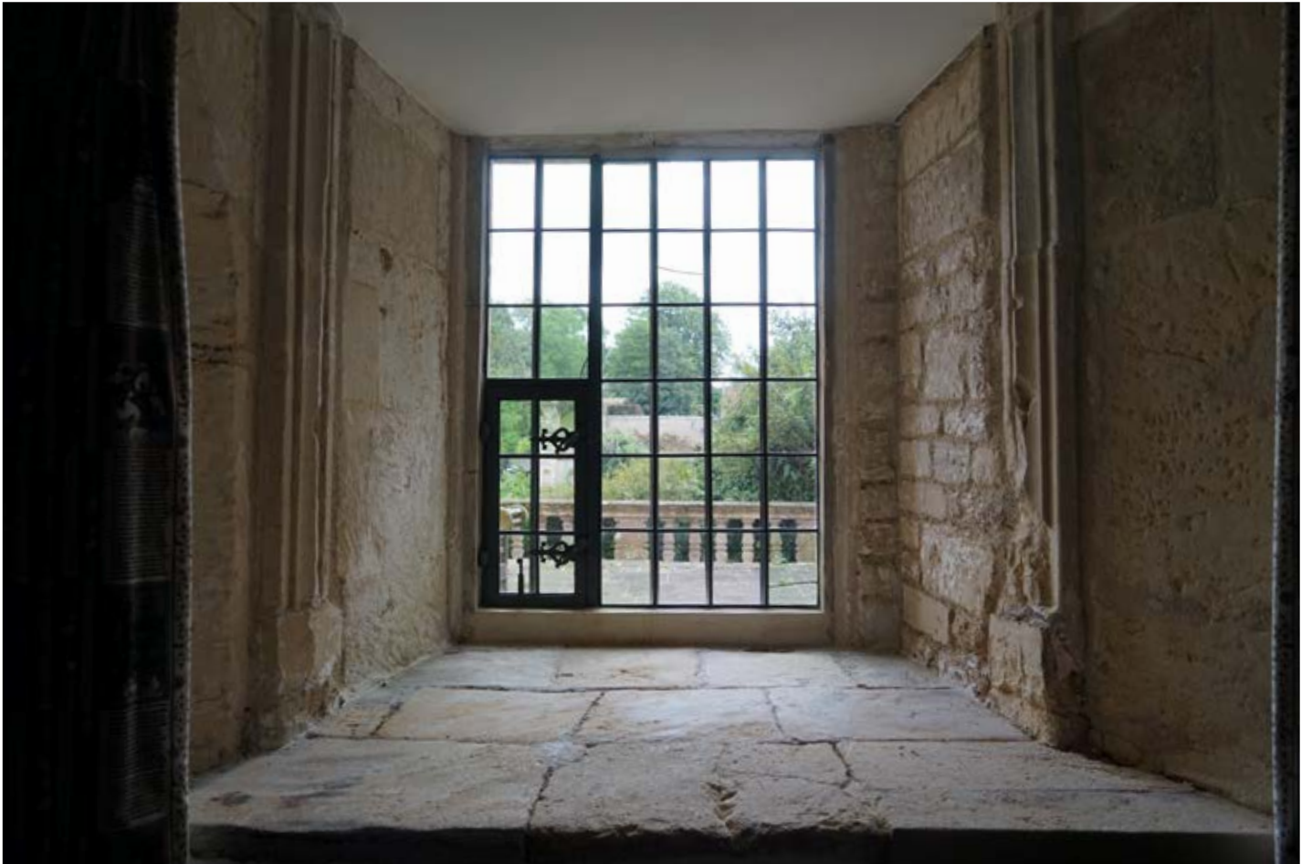
Detail of Library window, looking out over front terrace (west elevation).
