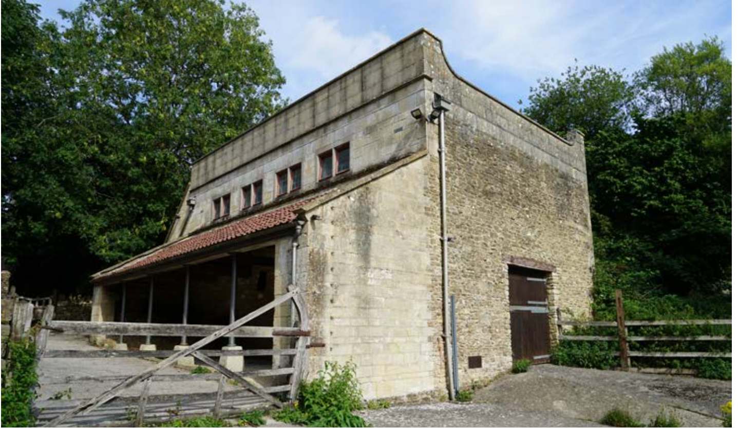
Squash court with open cart shed side extension to the north.
