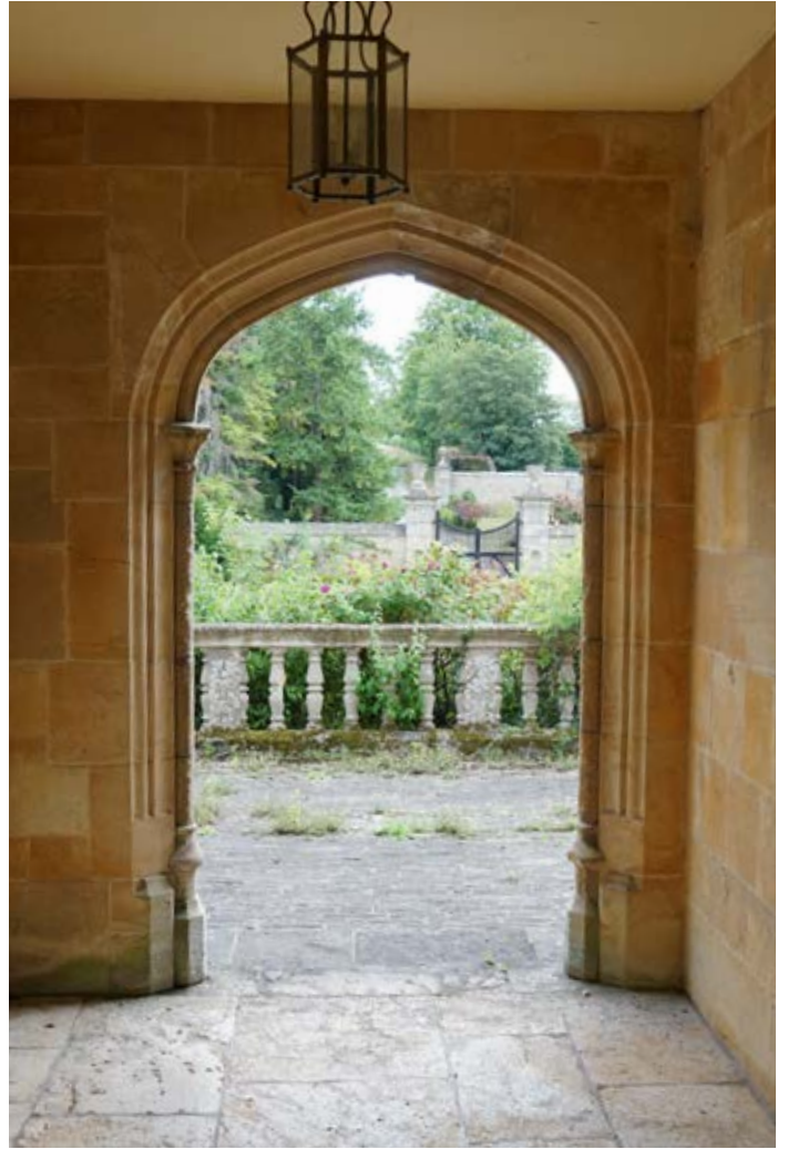
View out into Entrance Porch. Four-centred arch with engaged pilasters open to the outside.
