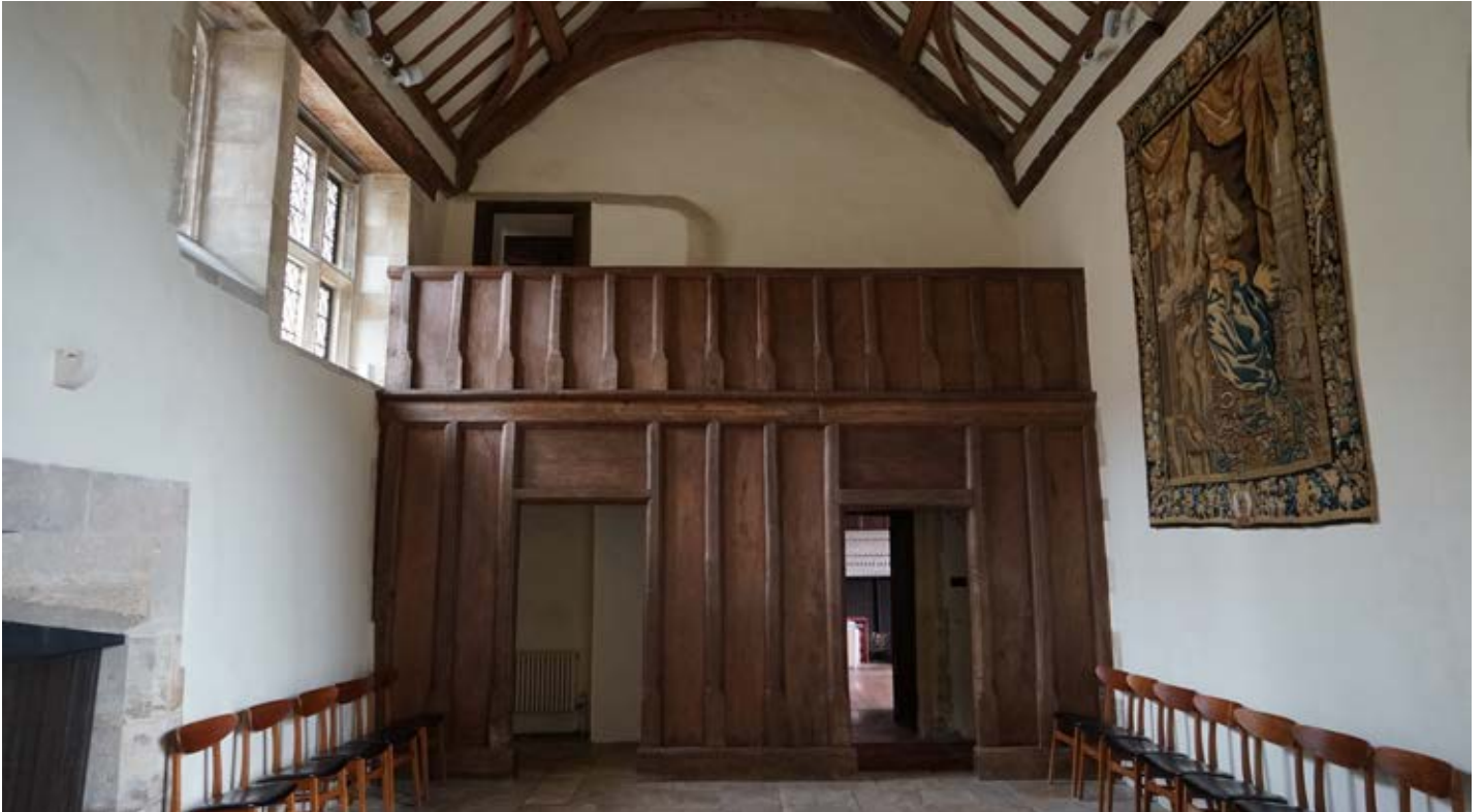
The Great Hall looking towards Screens Passage with Gallery over. Timber screen salvaged from a building in Barnstaple
