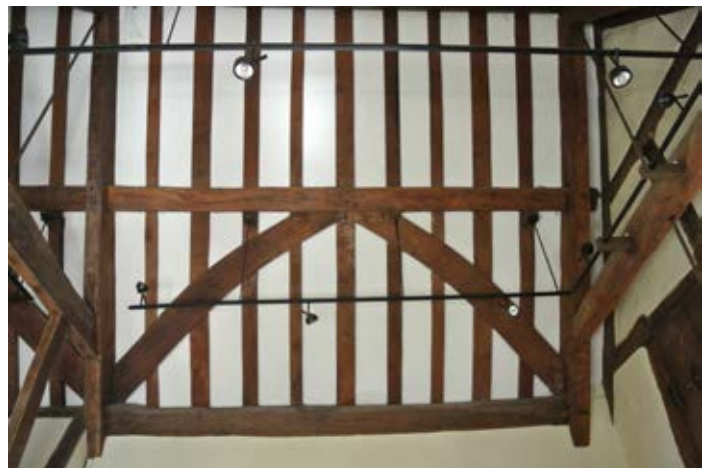
Detail of timber framing to landing area.
