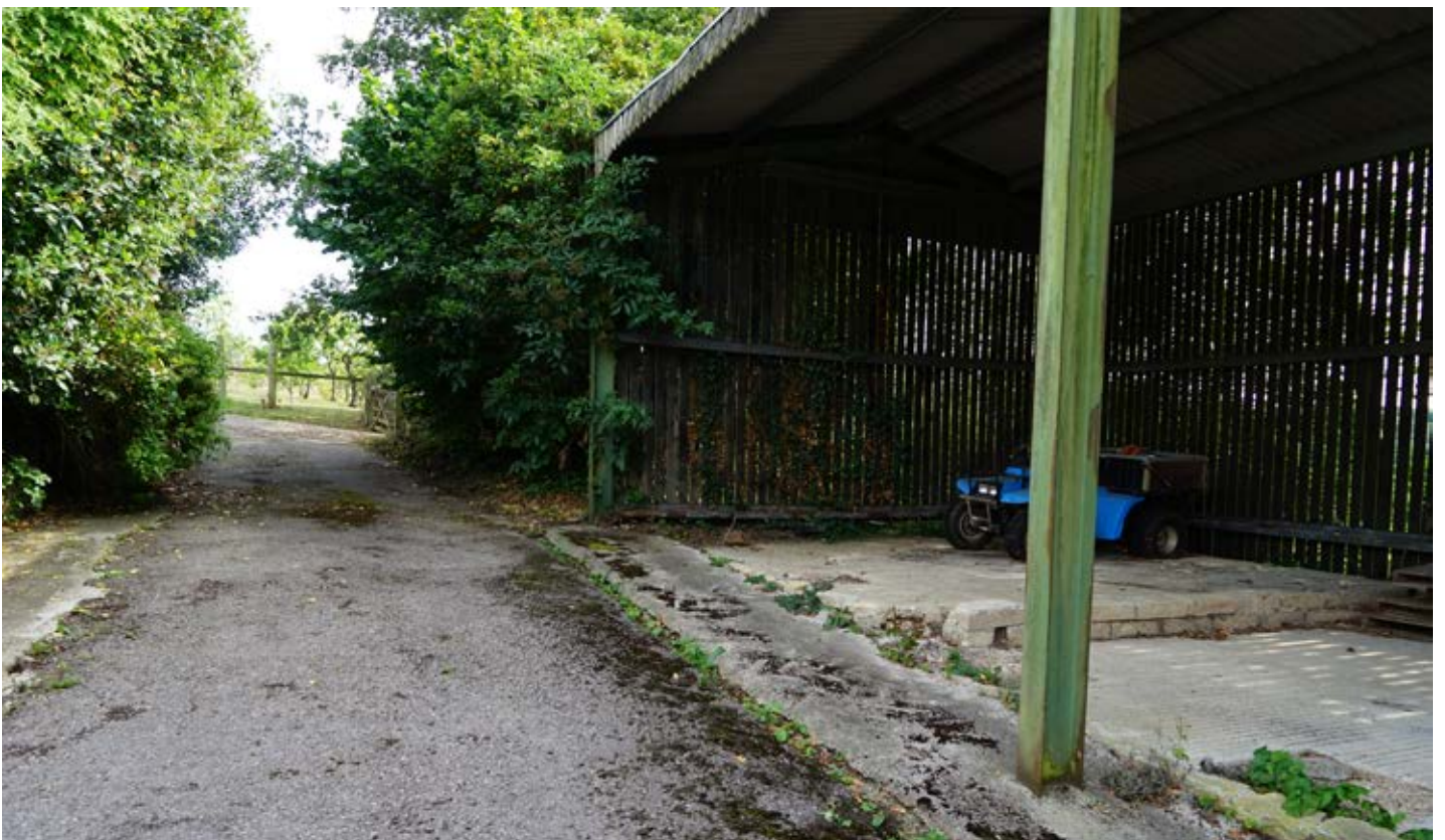
Dutch Barn / Parking - timber clad with steel structure.
