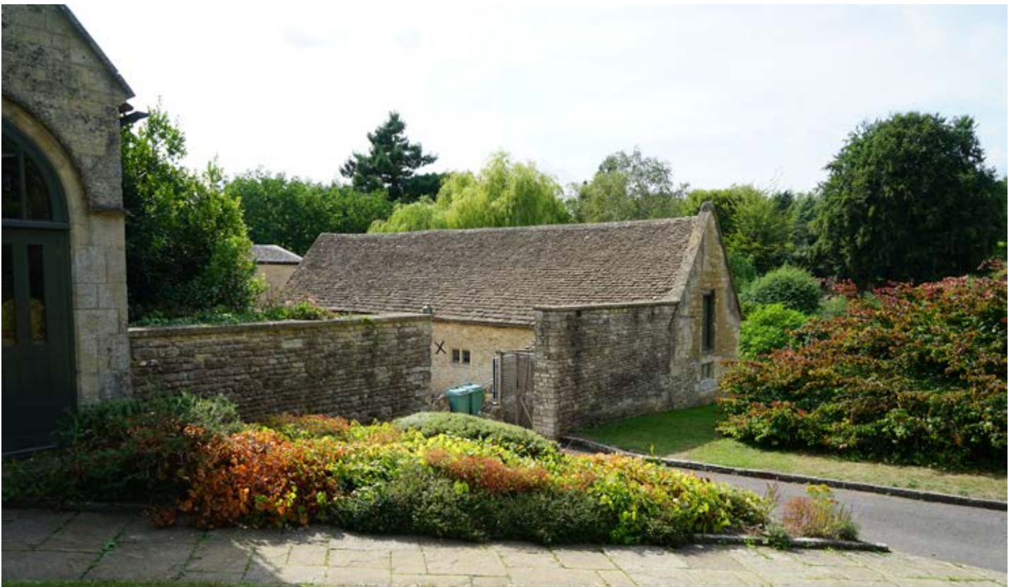
Stone wall linking coach house (left) and stable (right), enclosing courtyard.
