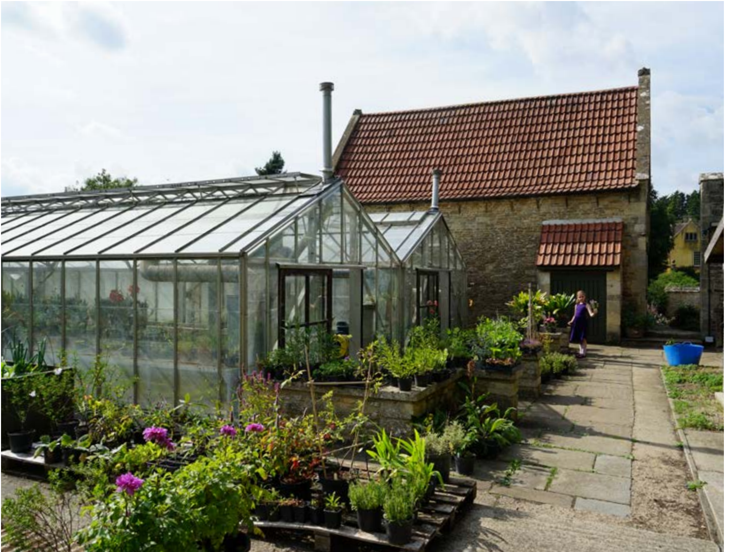
Modern greenhouses with coach house behind
