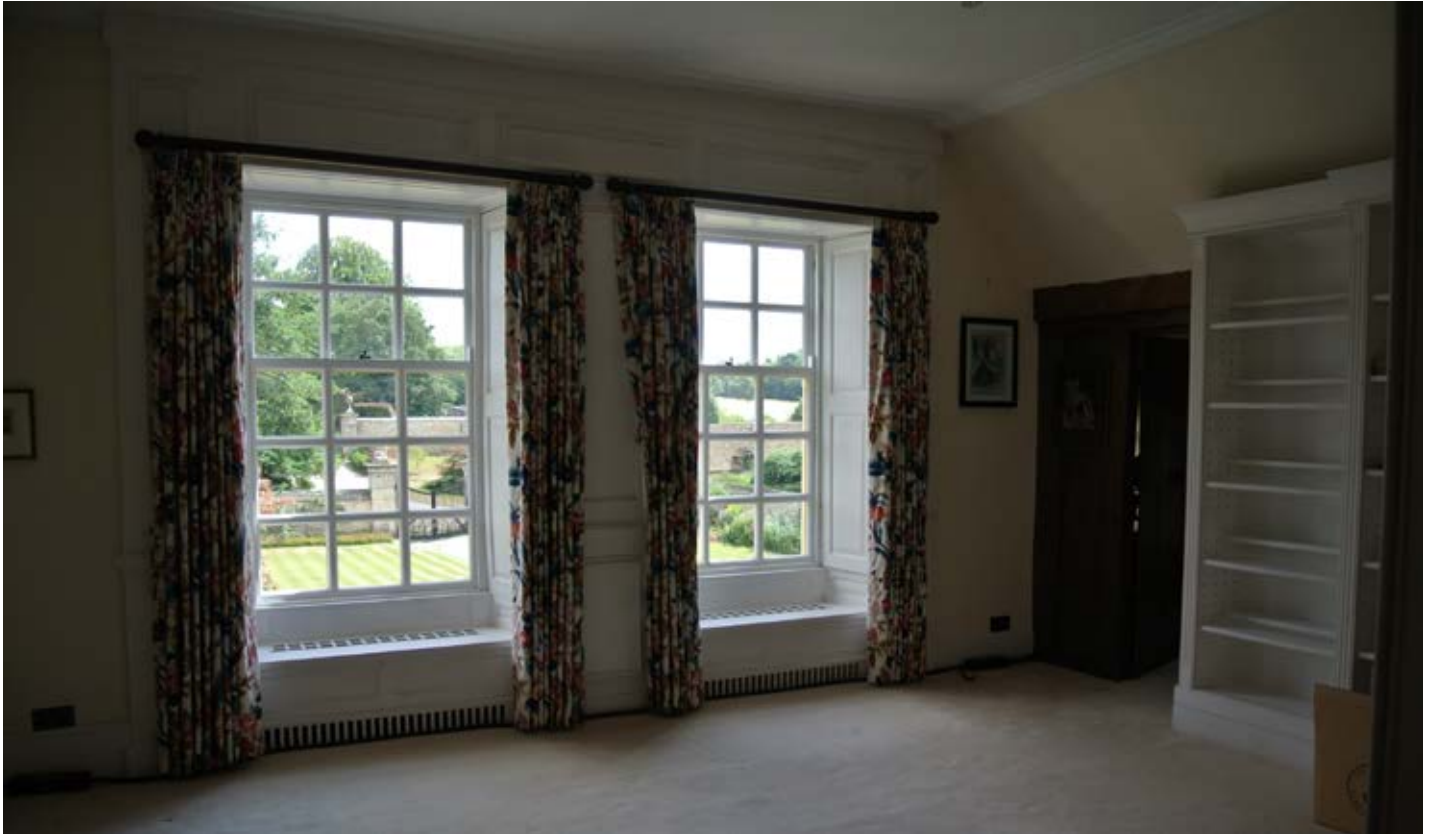
Bedroom with six-over-nine sash windows (modern replacements set in original frames with shutters).
