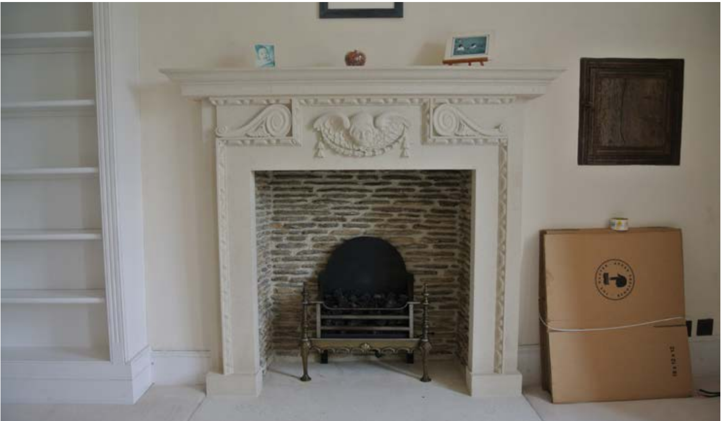
Fireplace in bedroom, a mix of reproduction classical surround, with brick slip fireback.
