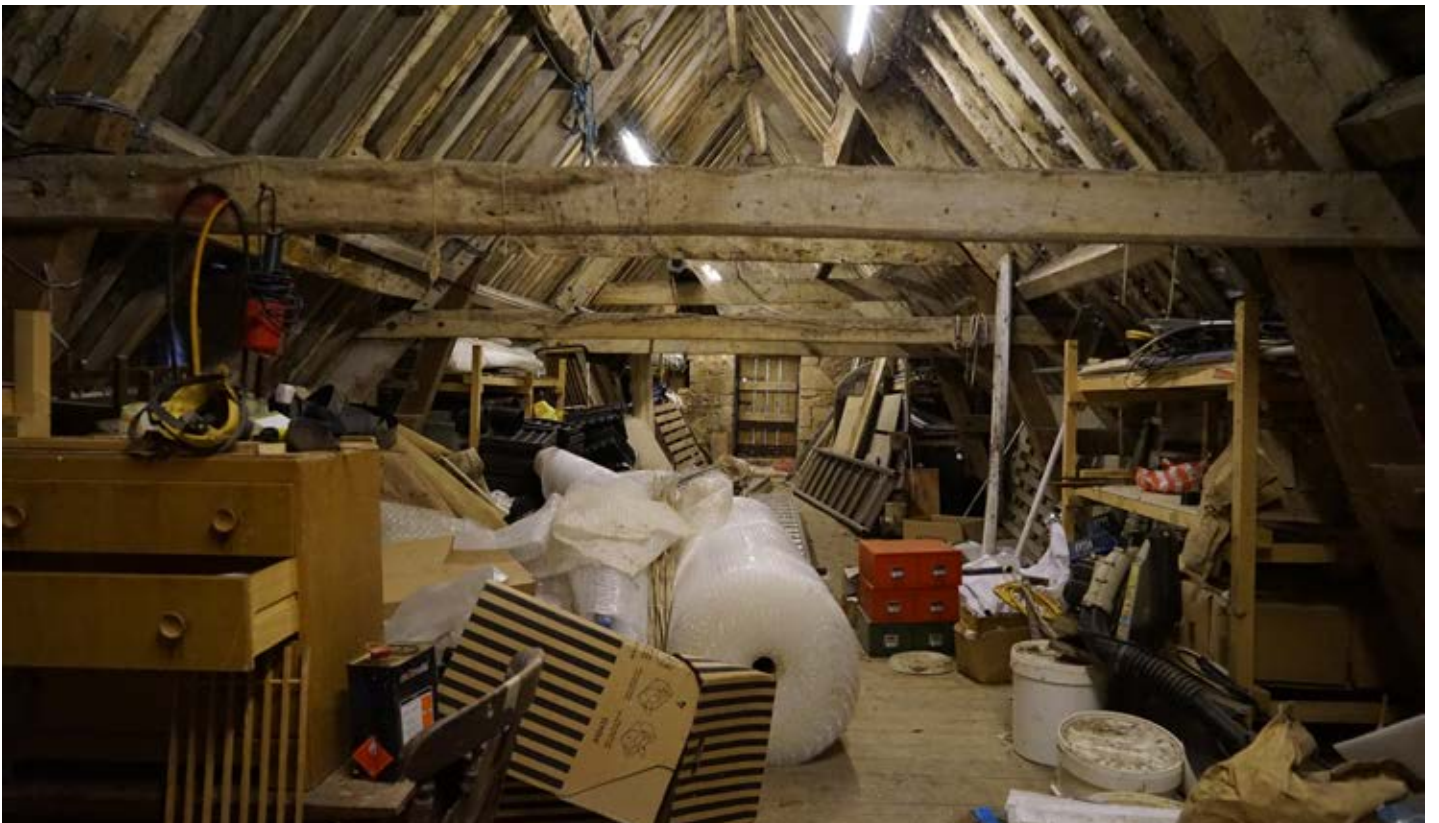
Interior view of hay loft above stable block.
