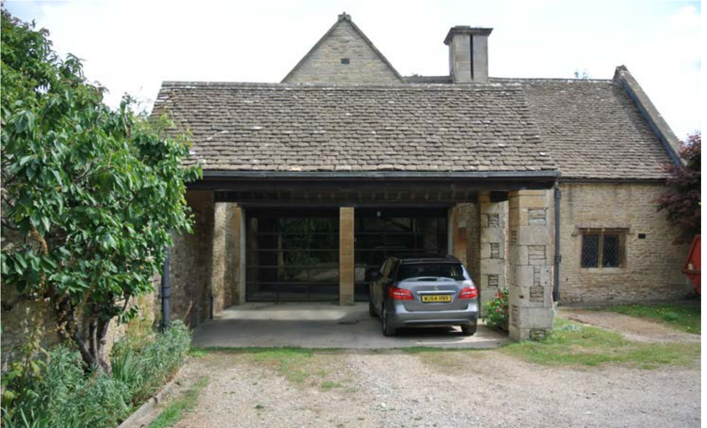
View from the North, including more recent carport extension.
