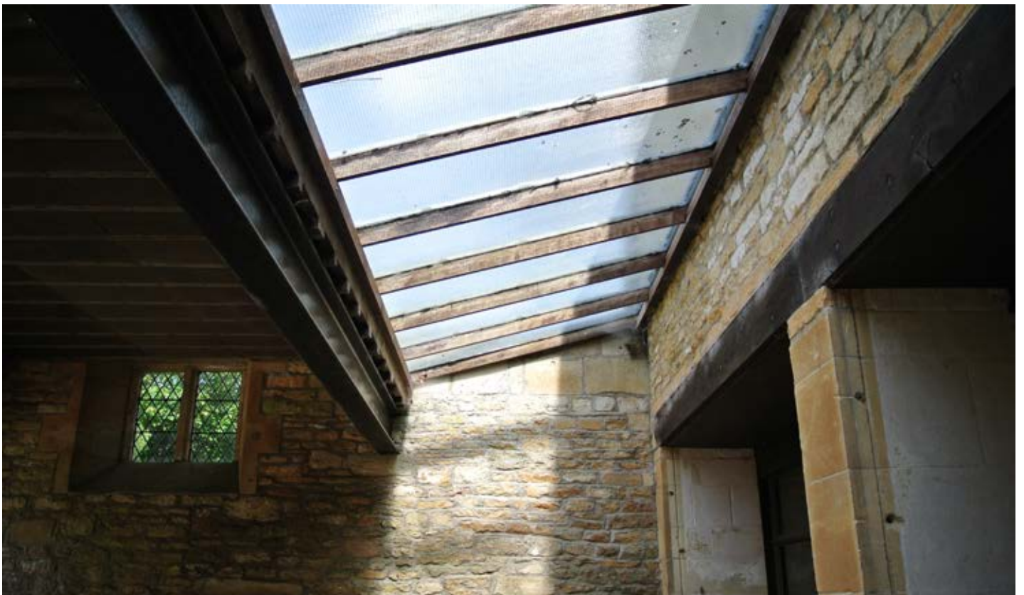
Glazed link between granary building and carport. Note lead light window into garden serving carport.
