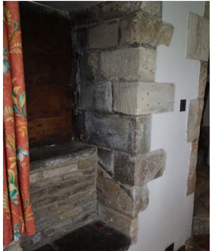
View of upper level space in room. Note small opening to the outside, suggesting delivery chute of some sort?? Brakspear plan has this room identified as 'heating chamber' so this could have been to deliver coal for heating boilers.
