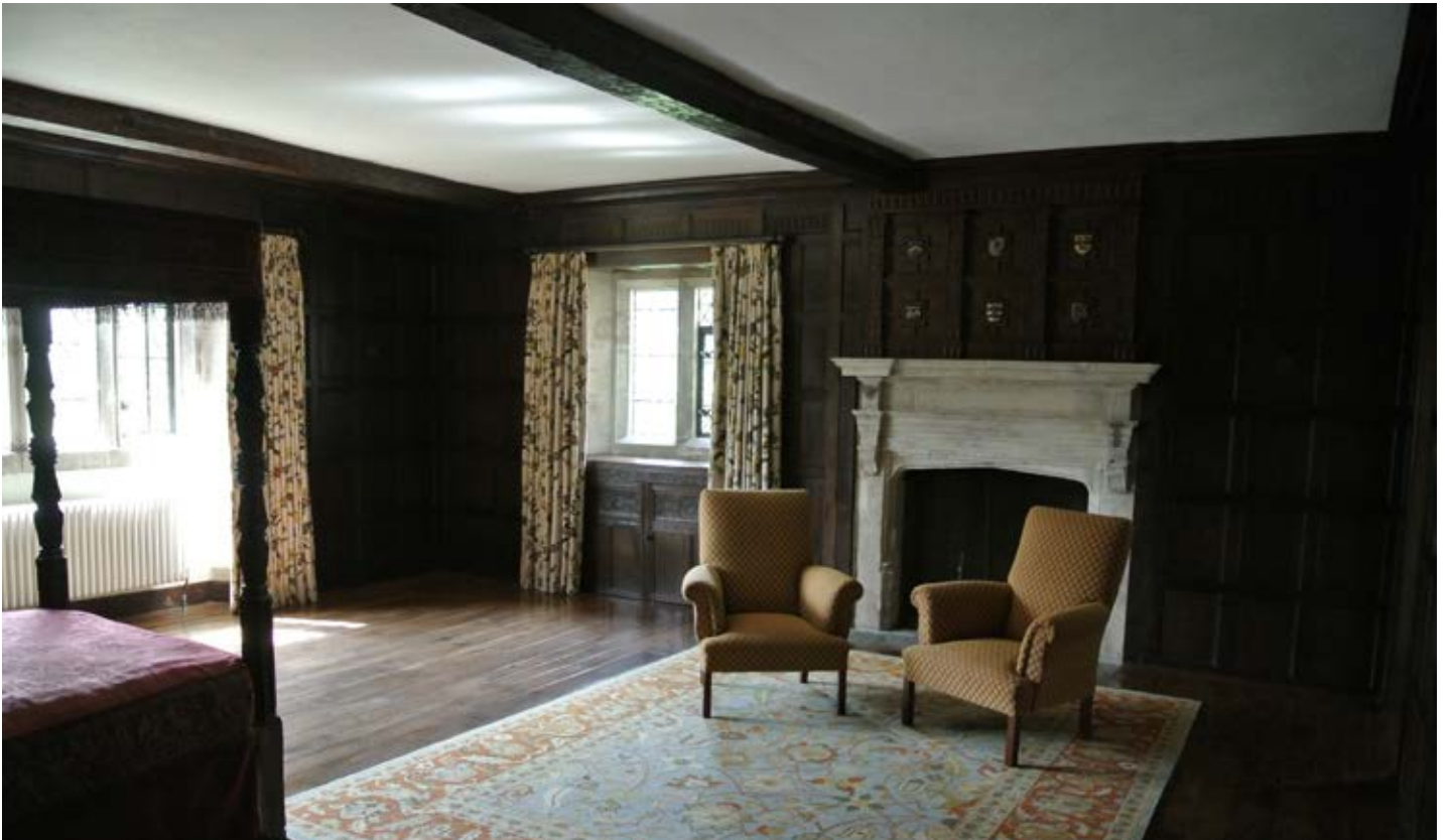
Fully panelled bedroom with stone fireplace and decorative panelling above. Stone mullion and transom, leaded light casement windows.
