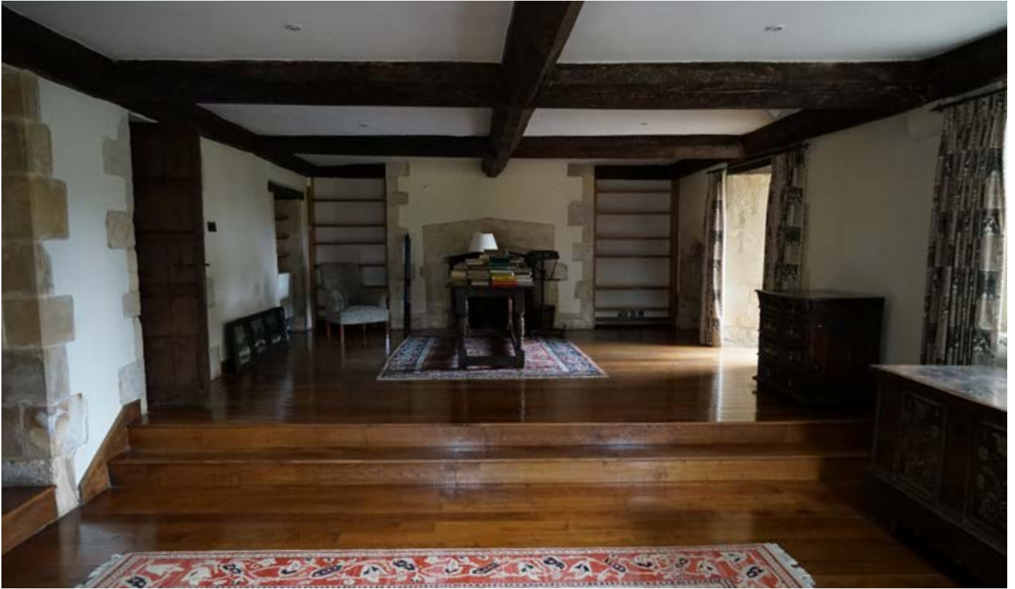
Library, looking towards fireplace. Chamfered beams to ceiling (16th century) and stone quoins to openings around the room.
