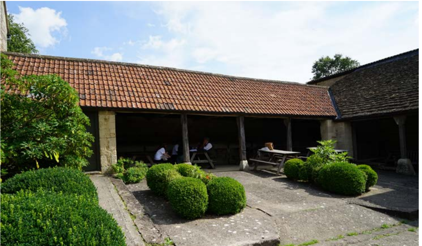
Single storey coach house range to courtyard
