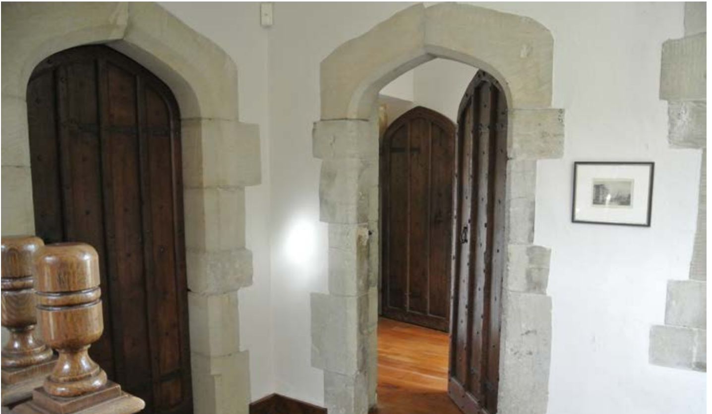
Hallway landing with four-centred arch stone doorways leading to rooms beyond.
