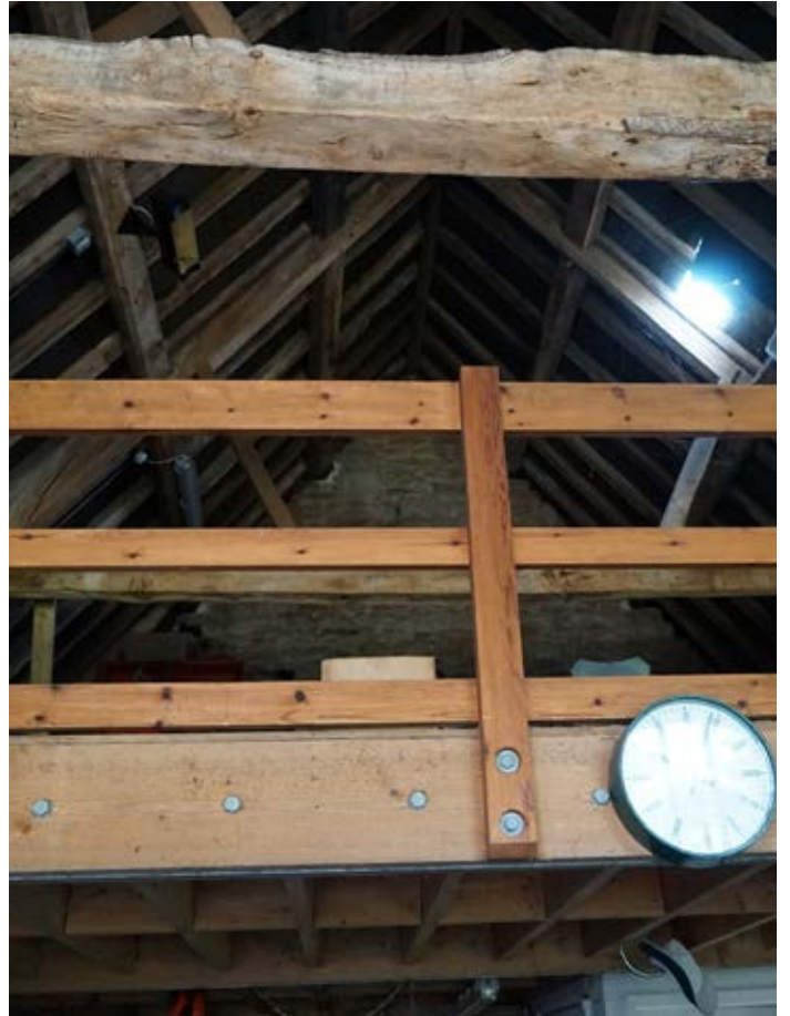
Interior of double height coach house with modern inserted mezzanine.
