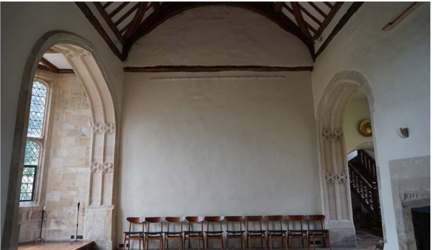
The Great Hall looking towards the High End, with canted bay to the front elevation (left in photo), added by Brakspear to original 16th century design.
