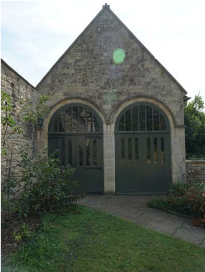
Gable end elevation of coach house (east)
