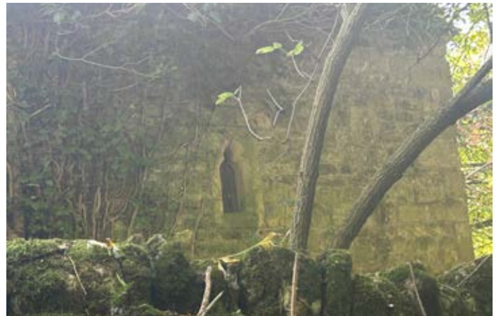
L1 - Detail of small window in end wall.
