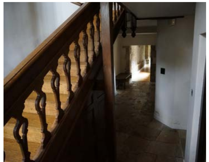
Details of north west staircase, with splat balusters and newel post finials - assumed to be Brakspear design.
