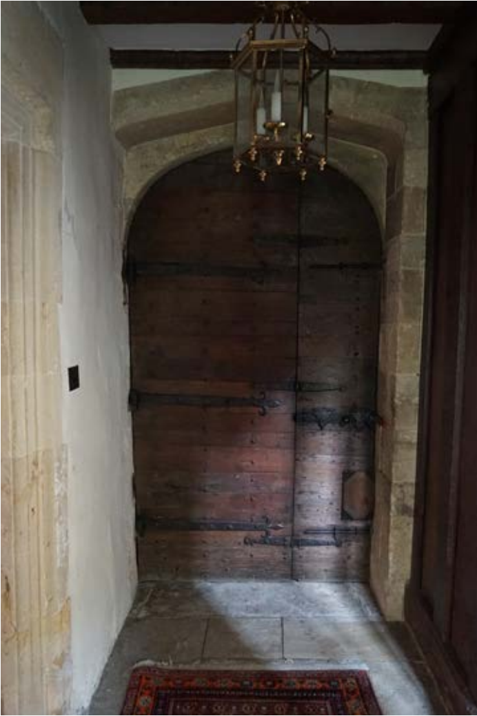
Main front door into Entrance Porch, off Screens Passage.
