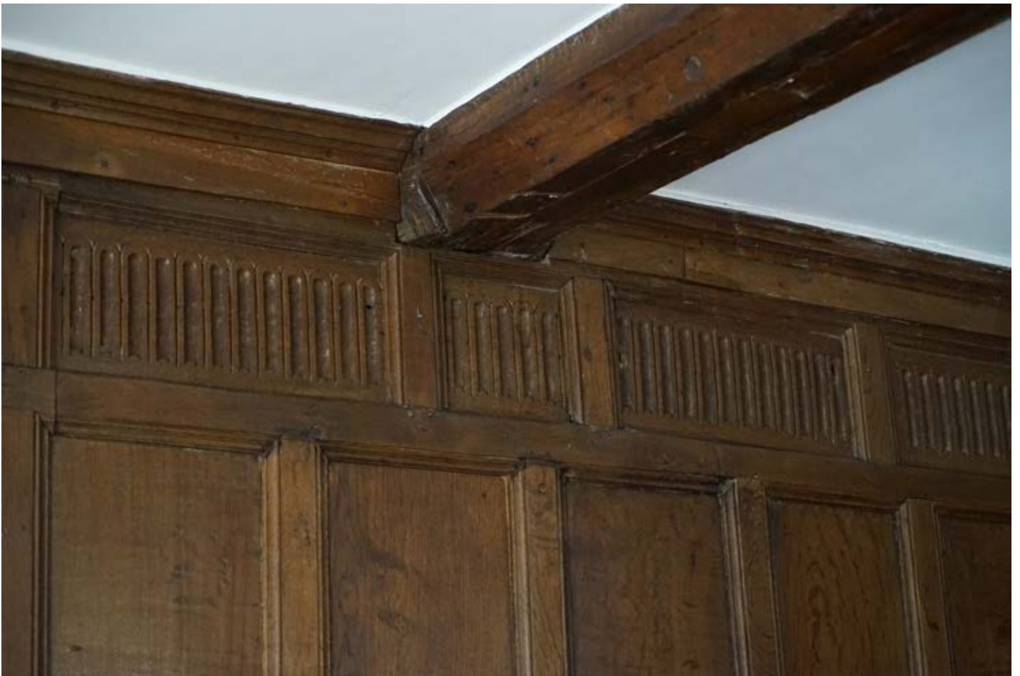
Details of timber panelling to dining room, with stopped and chamfered beam to centre of the room.
