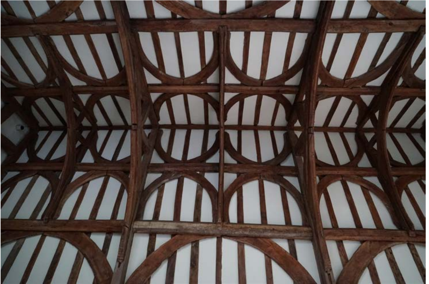
Roof timbers to The Great Hall dating back to c.1500, with its impressive roof structure of six bay double-purlin windbraced hall roof with arch-braced collar trusses.
