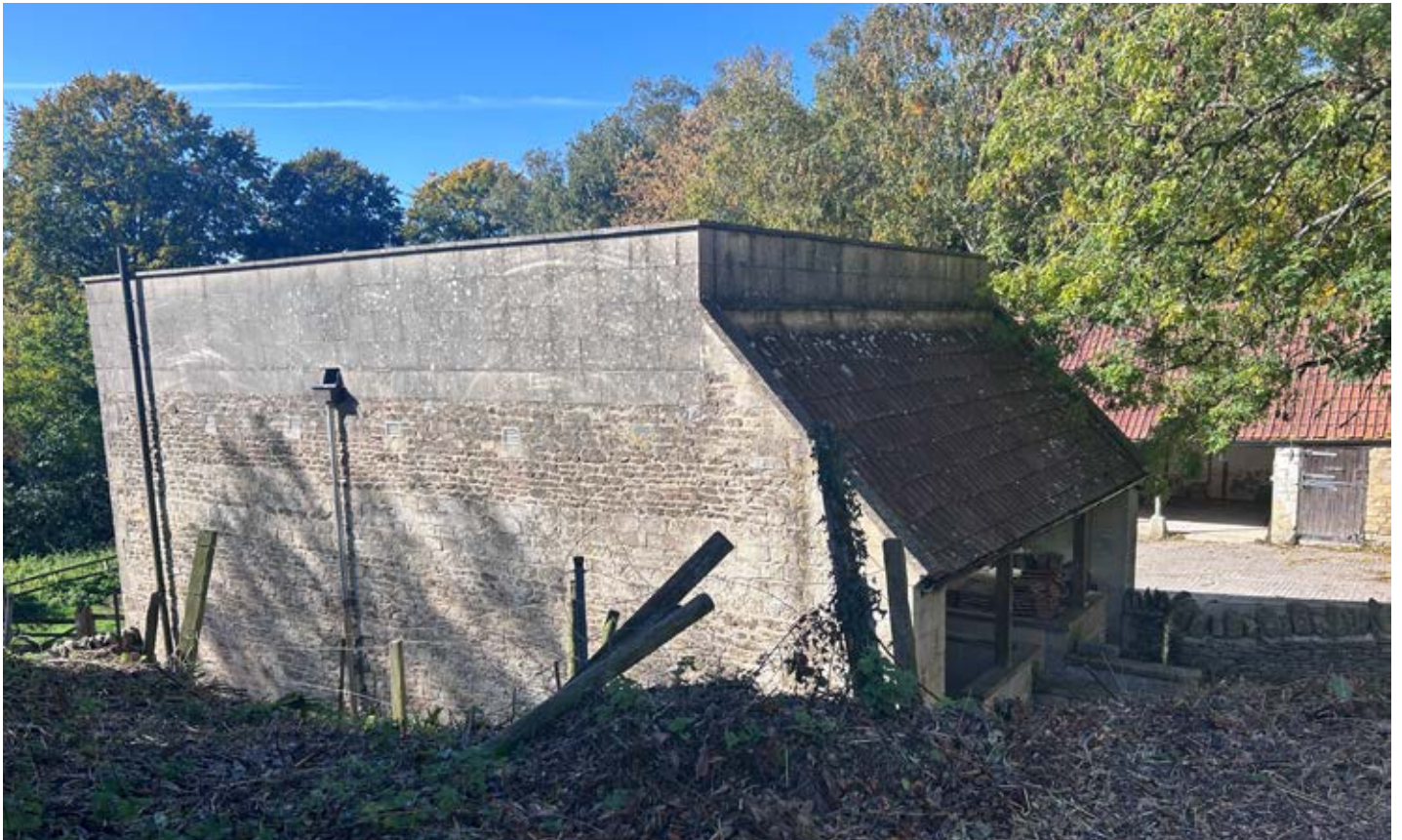
View of south elevation wall of squash court building - note modern square top over older stonework.
