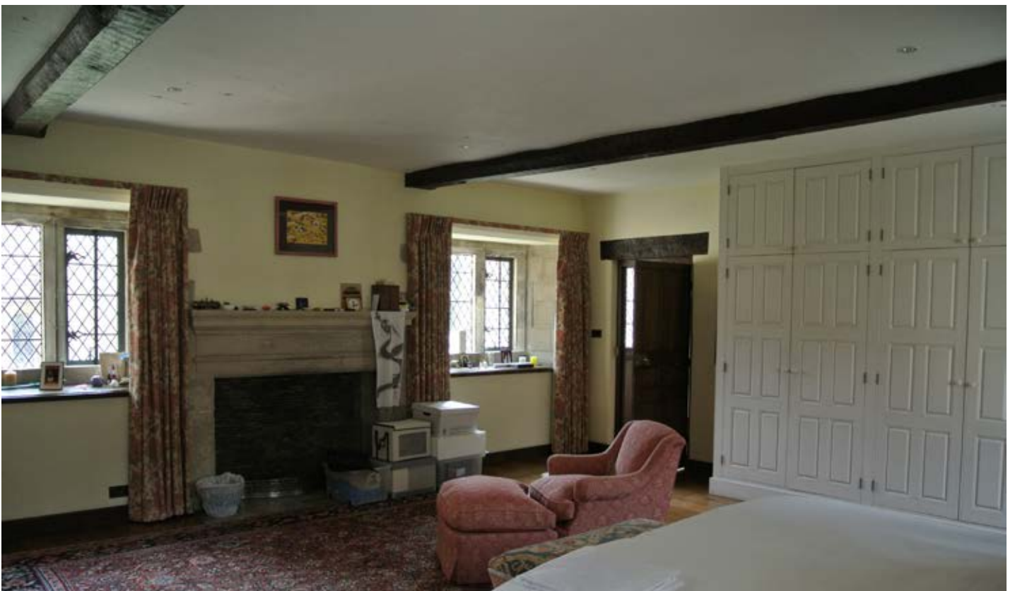
Lead-light stone mullion casement windows look out onto inner courtyard. Stone fireplace surround.
