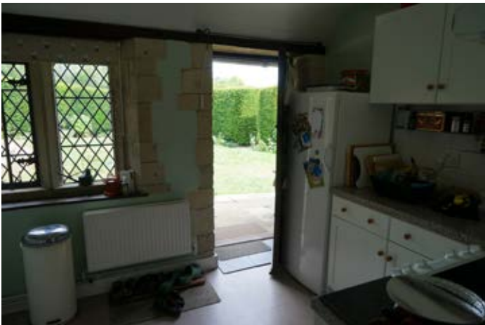
Stone mullioned, lead-light casement window to the kitchen.
