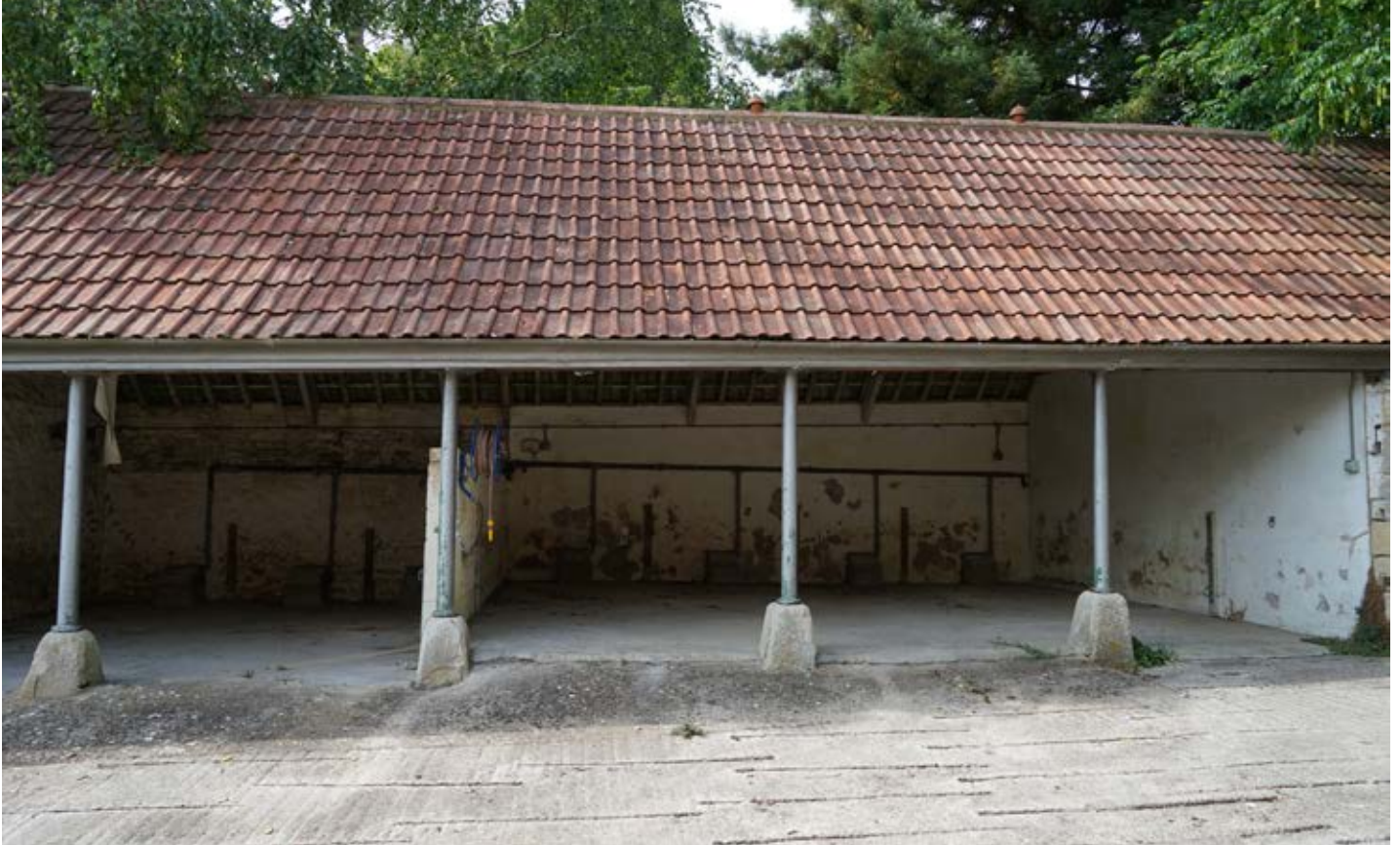
Open fronted cart shed with steel posts on concrete blocks.
