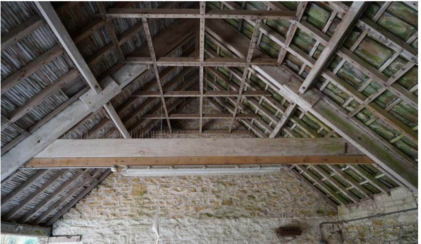
Interior roof structure of open cart shed.
