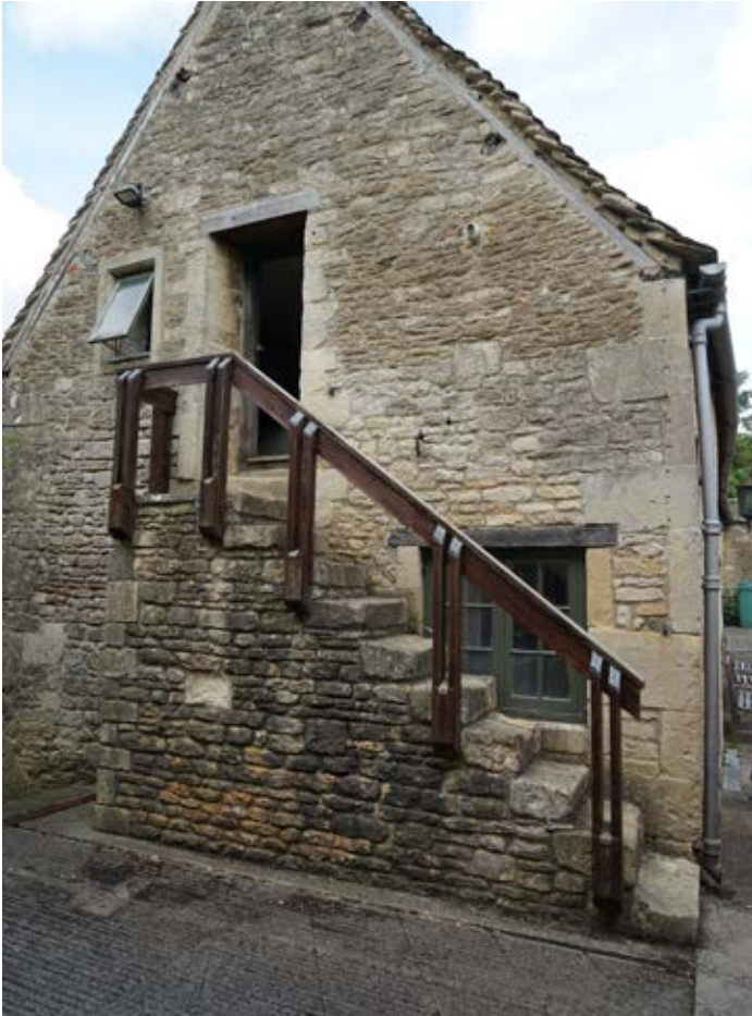
Stable block gable end elevation (west)
