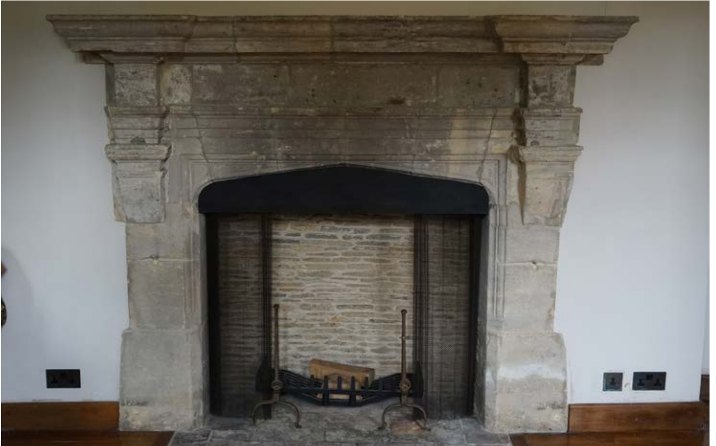
Detail of stone fireplace with four-centred arched opening; console brackets supporting pedimented mantle shelf.
