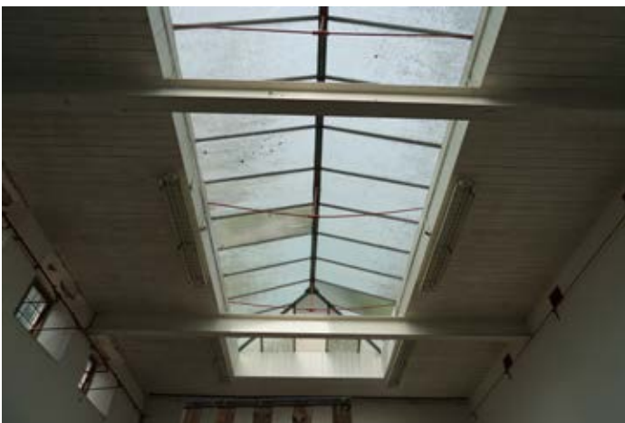
Rooflight to interior of Squash court.
