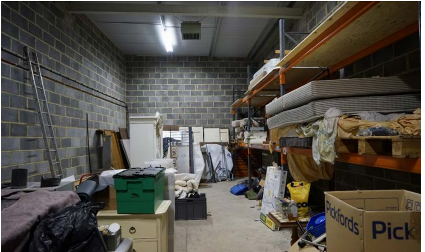
Interior of barn with modern breeze block wall lining.
