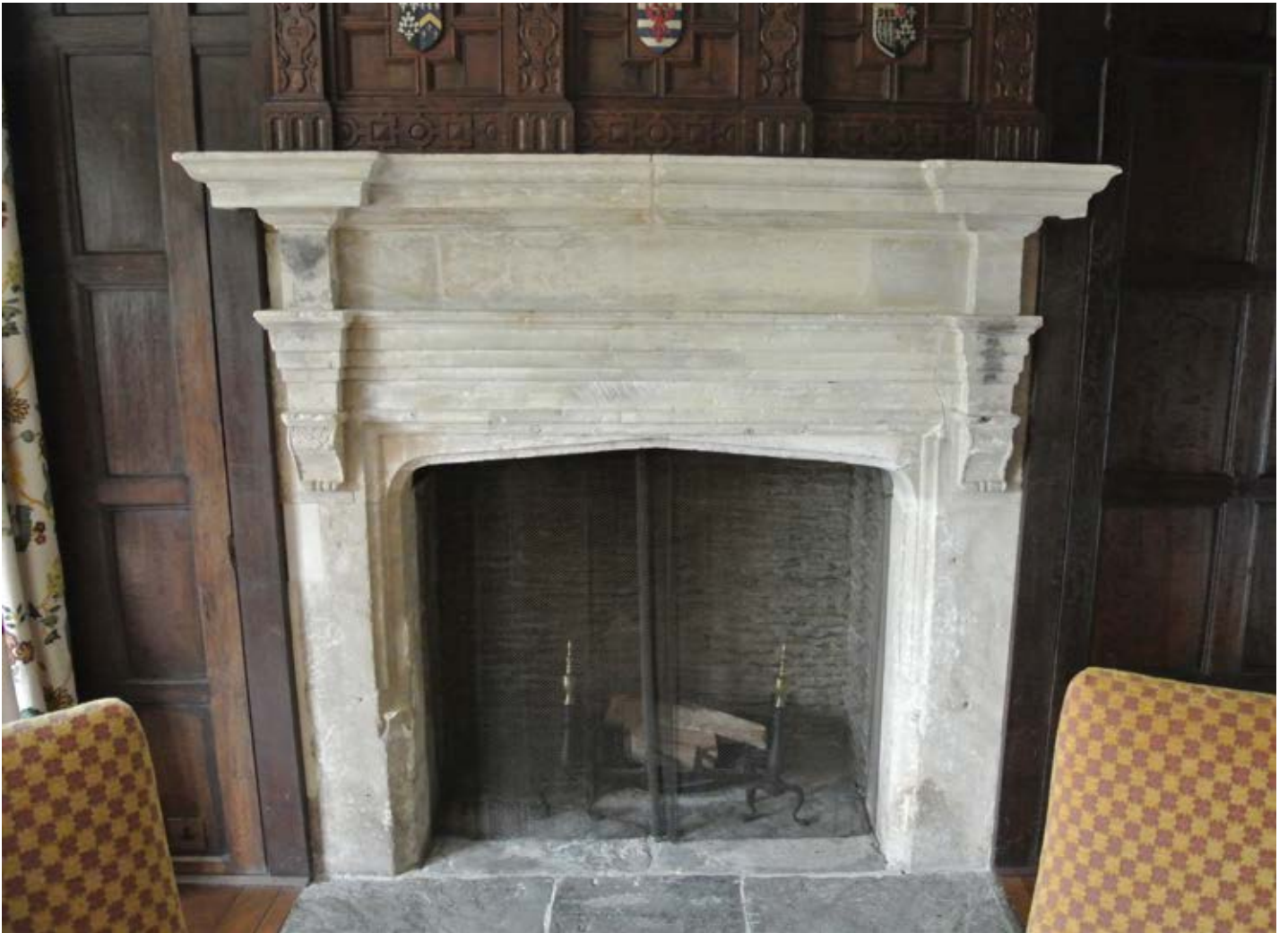
Stone fireplace to panelled bedroom, with corbelled support heavy mantleshaft.
