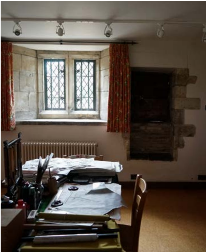
View of upper level space in room. Note small opening to the outside, suggesting delivery chute of some sort?? Brakspear plan has this room identified as 'heating chamber' so this could have been to deliver coal for heating boilers.
