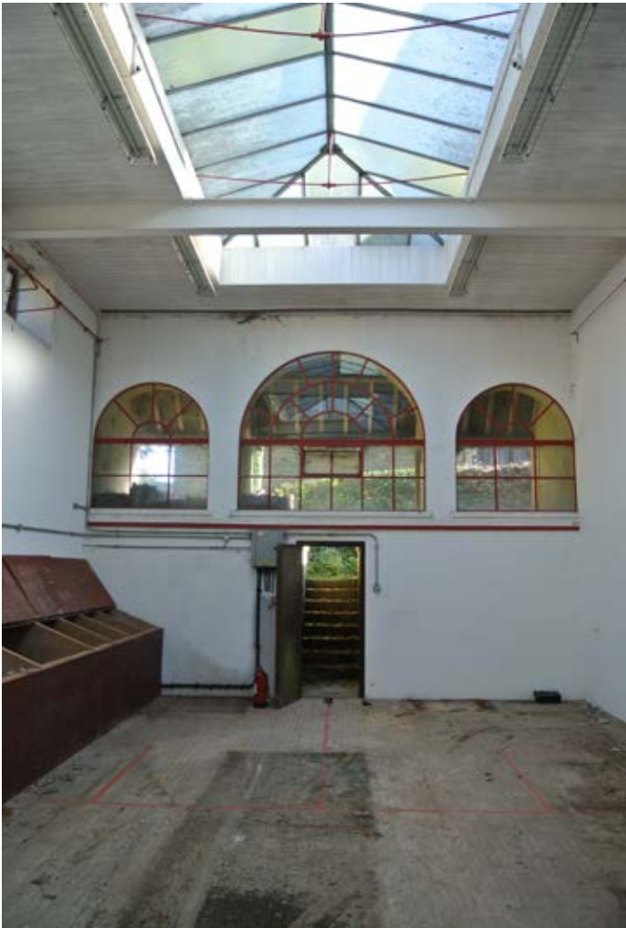
Squash court interior - entrance wall with viewing windows.
