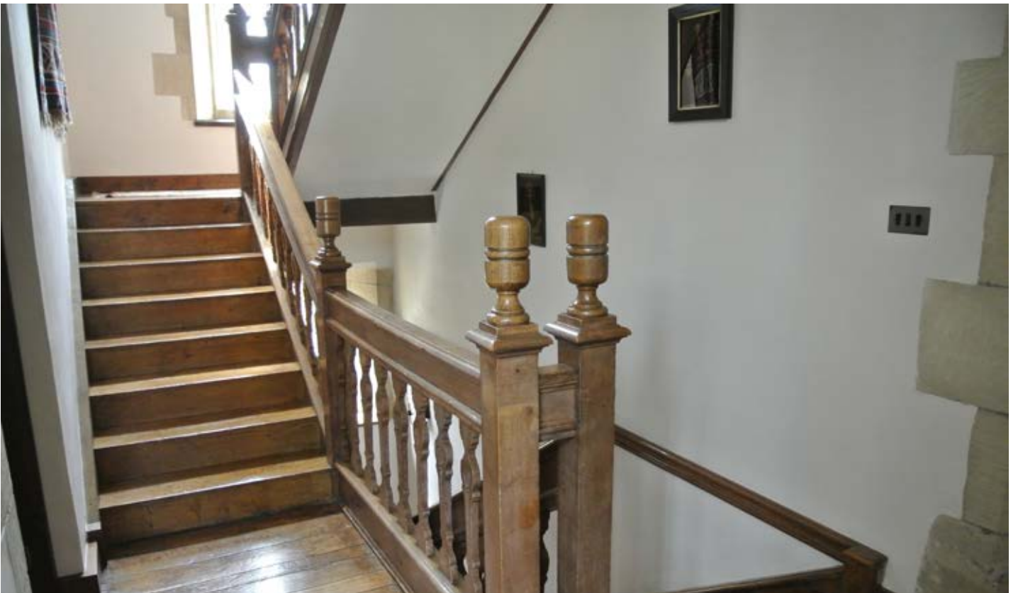
North west staircase serves ground to second floors. Splat balusters emulate those found on main staircase (20th century).
