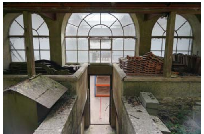
Arched glazing to entrance of Squash court with steps down.
