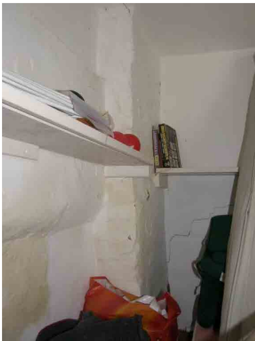
Fig. 25 Former flue to boiler
