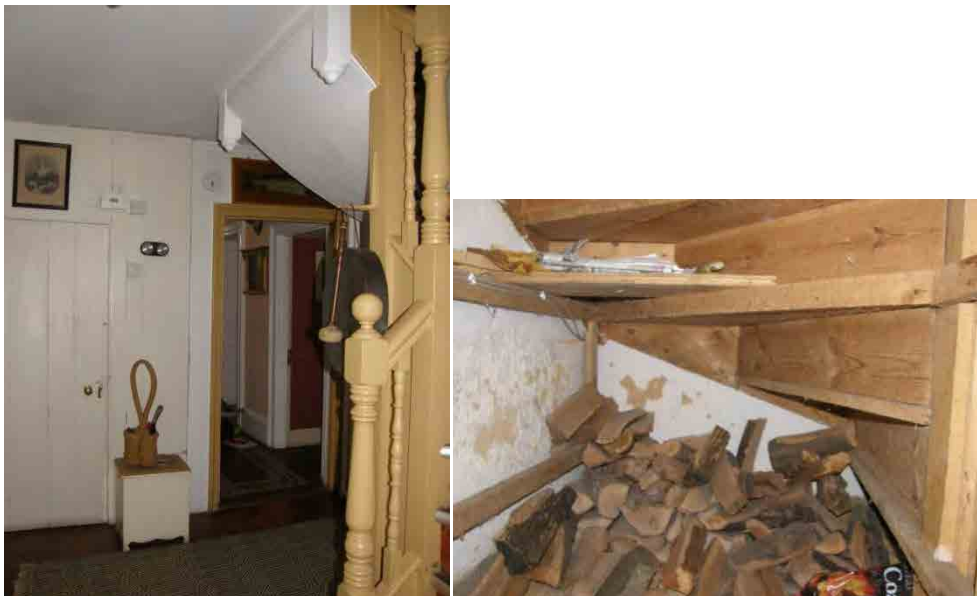
Fig. 13 Rear of hall with entrance to cellar on left Fig. 14 Construction of service stair
