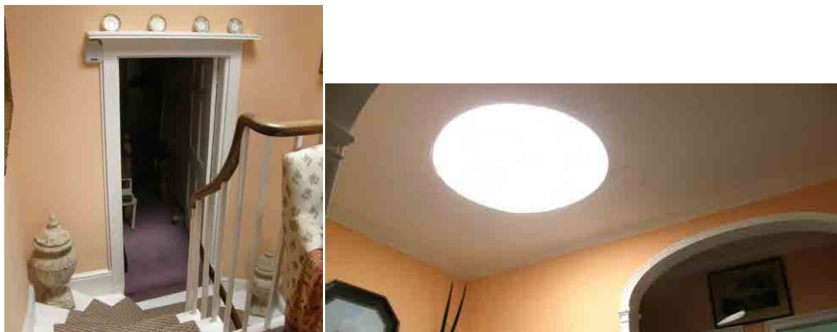
Fig. 28 Doorway connecting landing to rear extension
