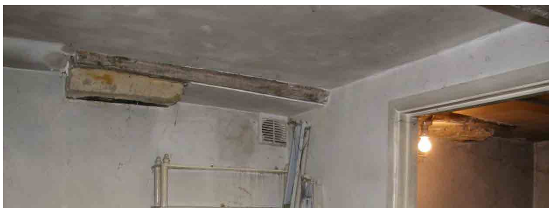
Fig. 67 Stone corbels once supporting the kitchen hearth above
