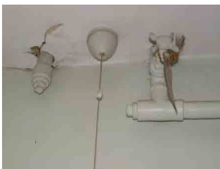
Fig. 44 Remains of older piping
