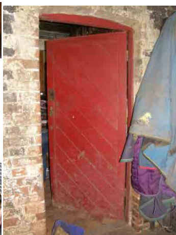
Fig. 72 Fireplace in tack room Fig. 73 Diagonally-boarded door Fig. 74 Stable interior
