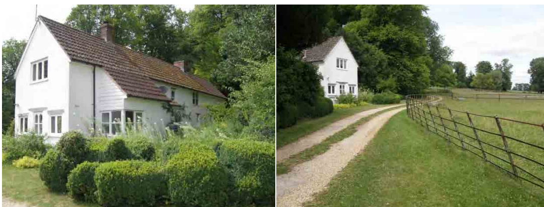
Fig. 75 Former lodge house Garden Cottage
