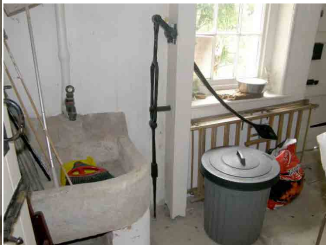
Fig. 26 Hand pump and stone sink
