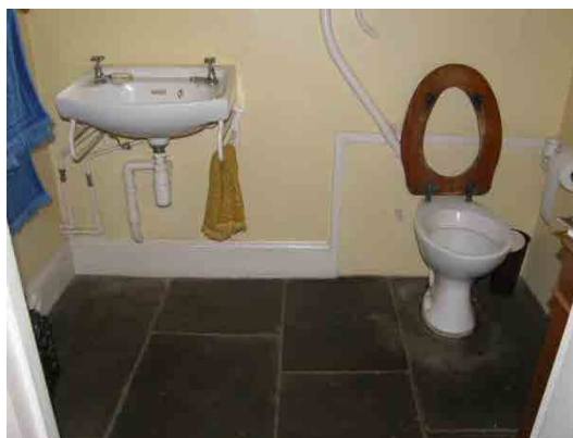
Fig. 16 WC of c1900 with later hand basin
