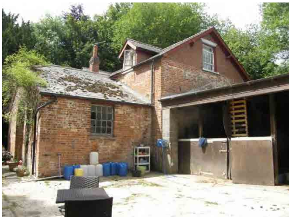
Fig. 70 Stables from east
