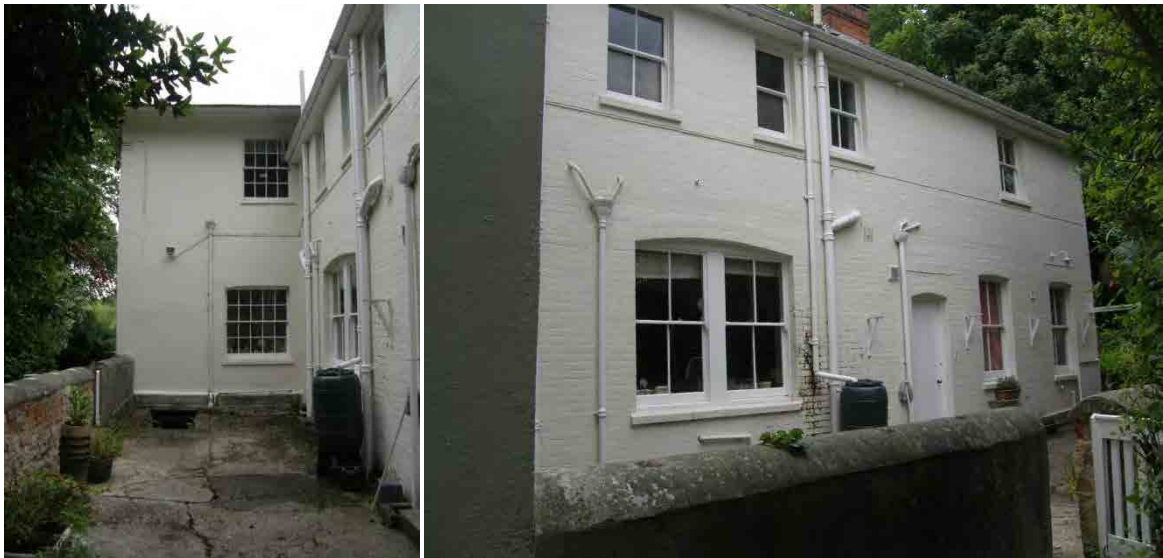
Fig. 5 Rear of main range, east side Fig. 6 East elevation of service wing
