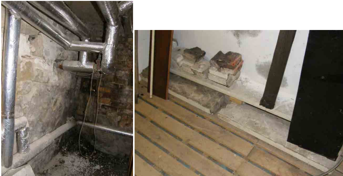
Fig. 68 Section of unplastered wall in area of heating ducts between rooms 5 & 6
