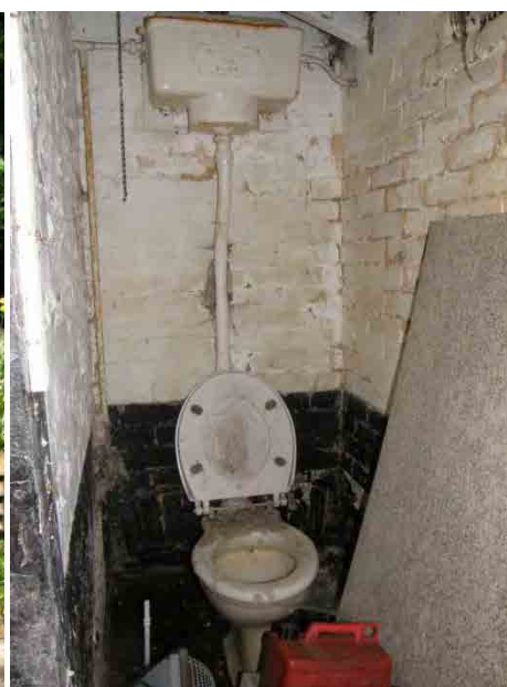
Fig. 78 WC attached on east side
