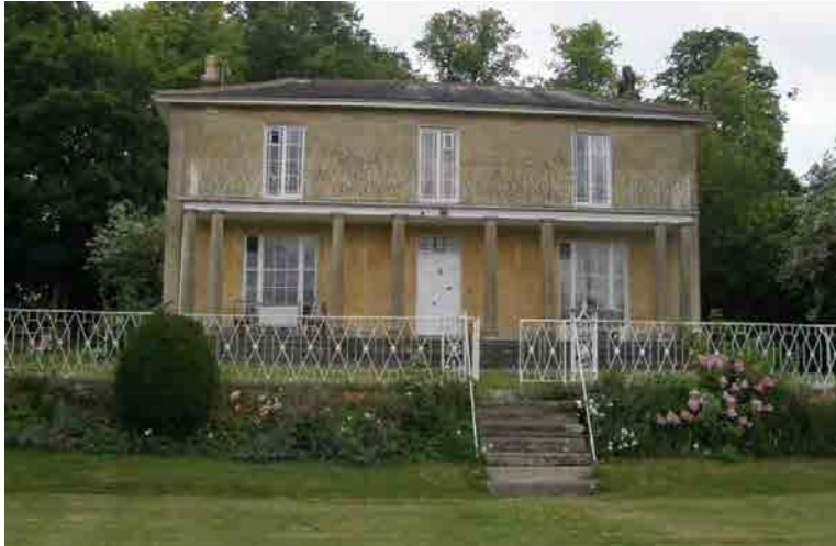
Fig. 1 Main south elevation and ornamental railings to terrace
