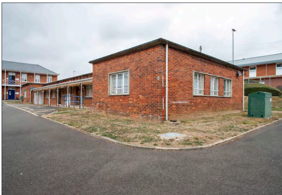
Photograph 7: Building JE 0 060 viewed from the south
