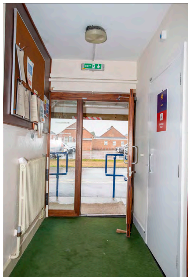
Photograph 18: Building JE 0 060 off-centre entrance lobby in the south-west half of the building
