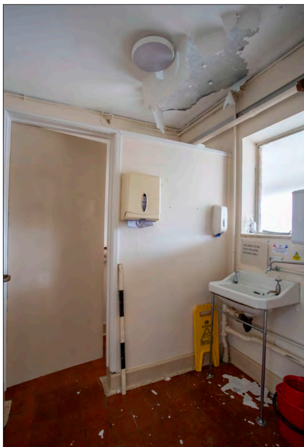
Photograph 17: Building JE 0 060 men's W.C. room G68
