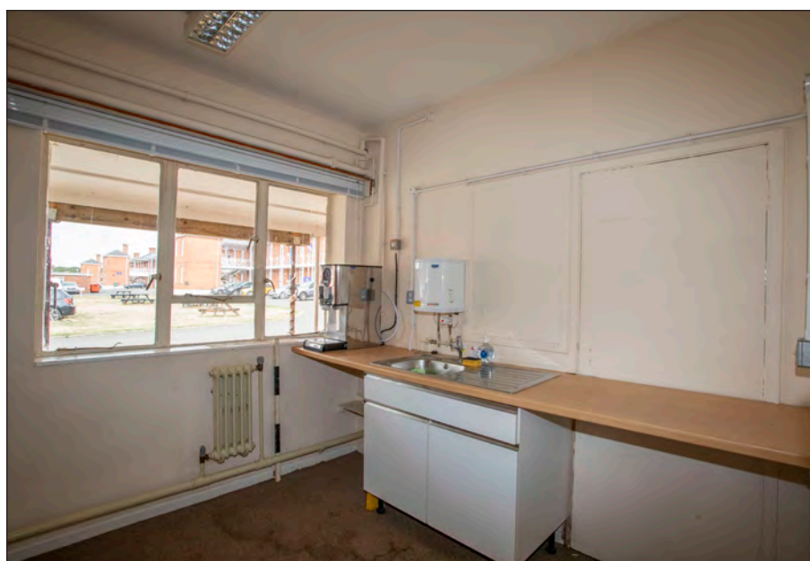
Photograph 34: Building JE 0 060 kitchen G66 with blocked door on the right
