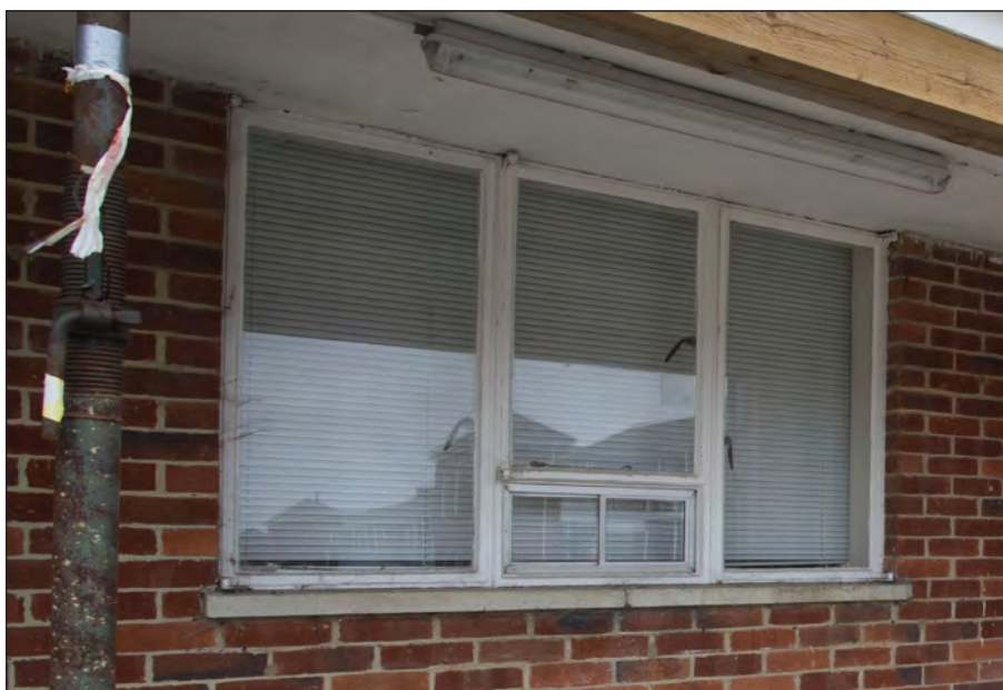
Photograph 14: Building JE 0 060 modified 4-light triple casement window with an inserted hatch (to room G27)
