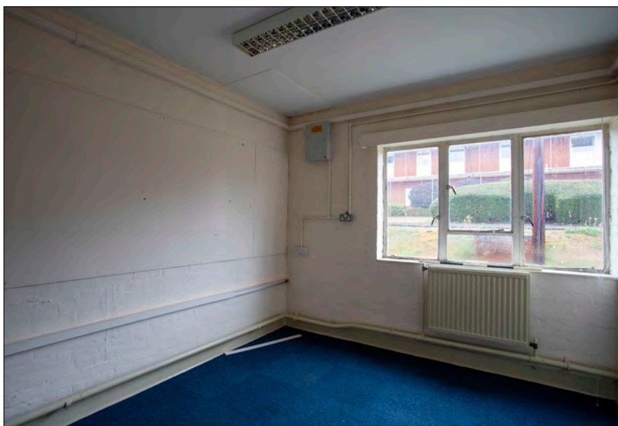
Photograph 40: Building JE 0 060 Officer Commanding (OC) office
