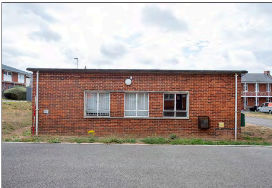
Photograph 3: Building JE 0 060 north-west end elevation
