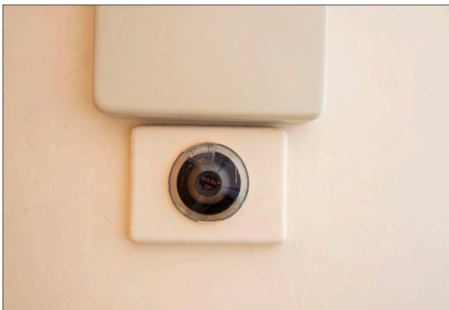
Photograph 36: Building JE 0 060 detail of Chubb Mark IV Manifoil combination lock
