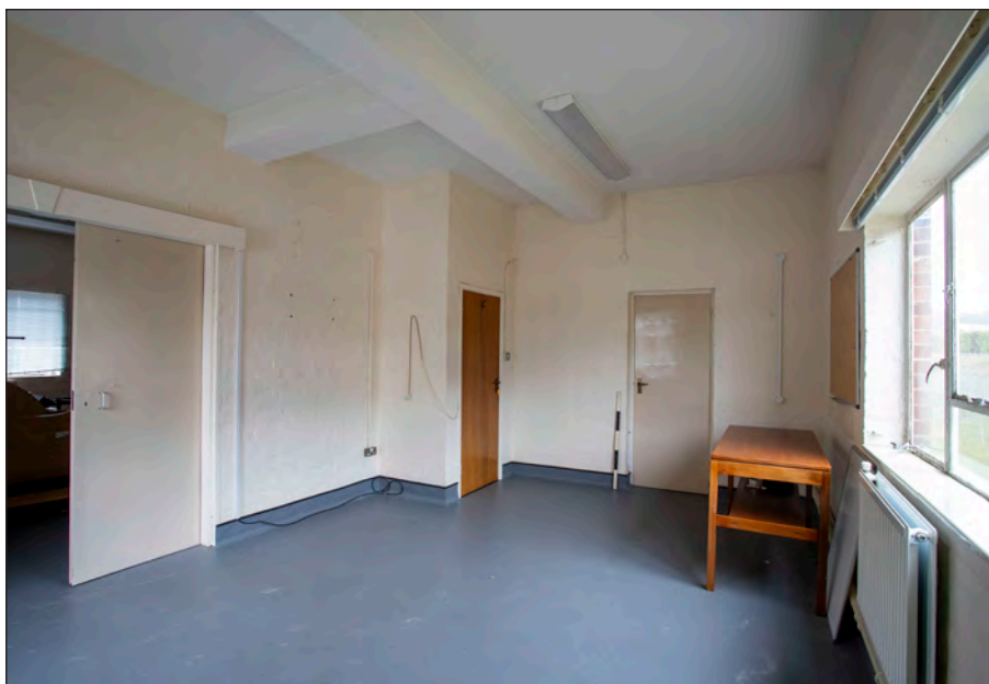
Photograph 41: Building JE 0 060 Commanding Officer (CO) office
