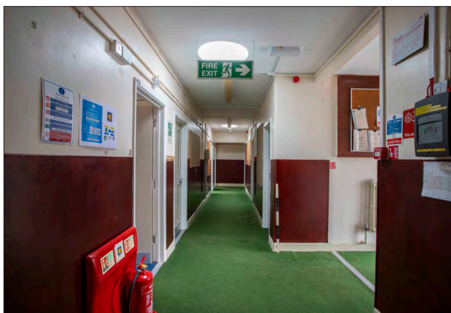
Photograph 22: Building JE 0 060 main corridor G37 in the south-eastern half
