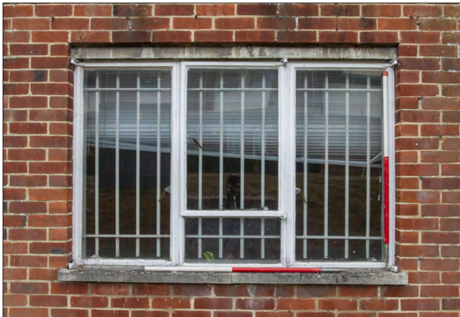
Photograph 13: Building JE 0 060 example of a 4-light triple casement window
