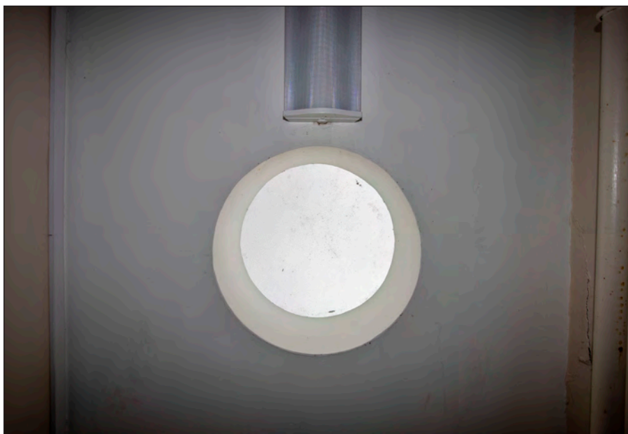
Photograph 23: Building JE 0 060 detail of the rooflights in the main corridor(s)
