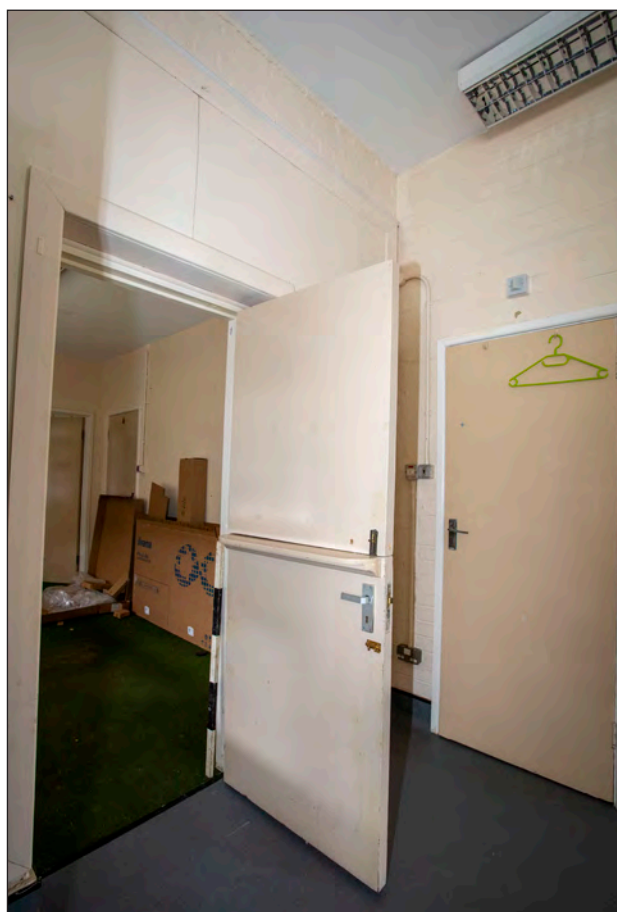
Photograph 44: Building JE 0 060 split door between rooms G26 and G27
