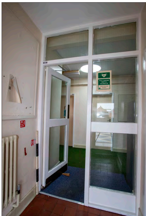
Photograph 15: Building JE 0 060, off-centre entrance lobby in the north-west half of the building
