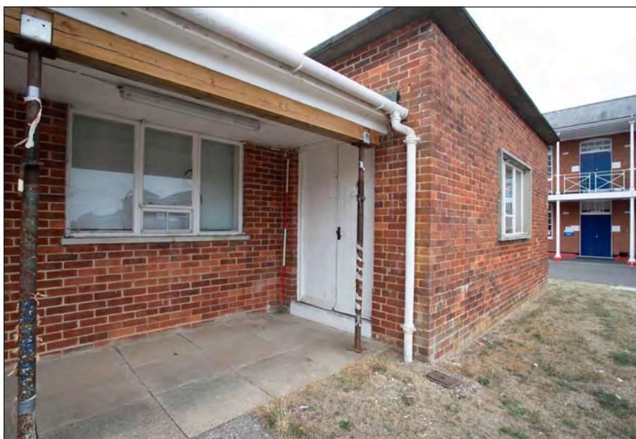
Photograph 10: Building JE 0 060 entrance into the south-east end of the building
