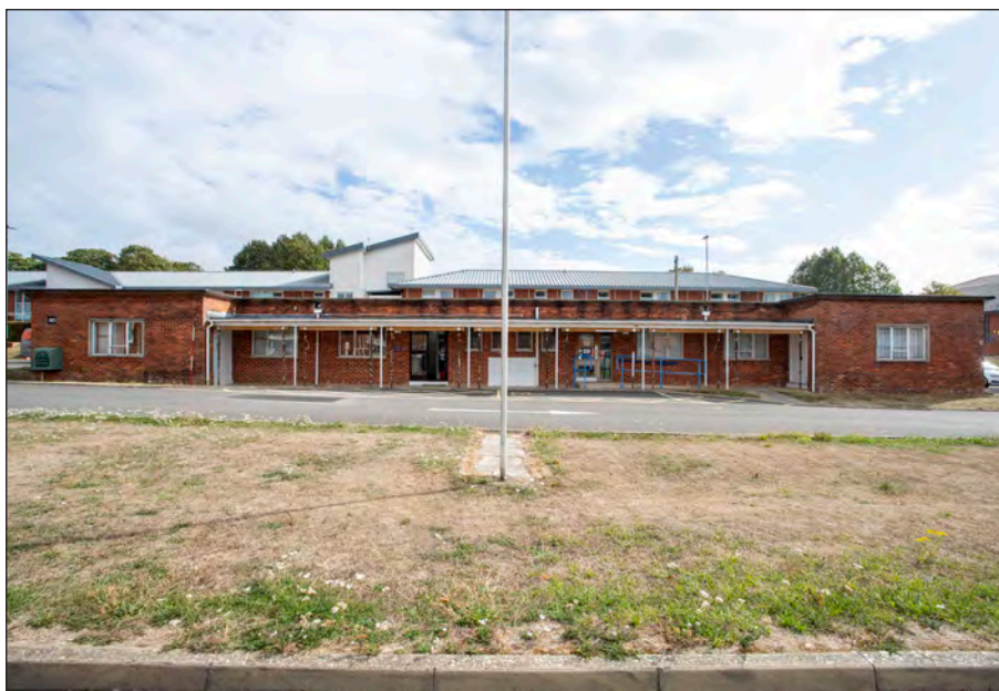
Photograph 1: Building JE 0 060, Jellalabad Barracks, Tidworth Garrison - front (south-west) elevation
