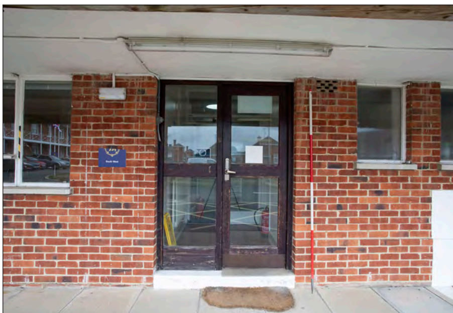
Photograph 8: Building JE 0 060 northern of the two off-centre front entrance
