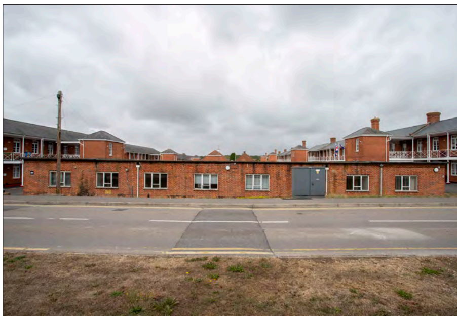
Photograph 5: Building JE 0 060 rear north-east elevation viewed from Kirkee Road
