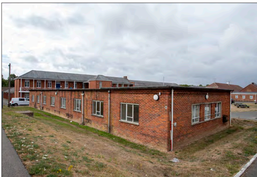
Photograph 4: Building JE 0 060 viewed from the north
