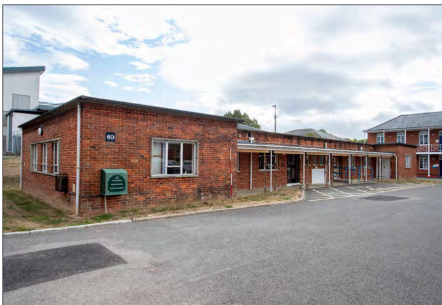
Photograph 2: Building JE 0 060 viewed from the west
