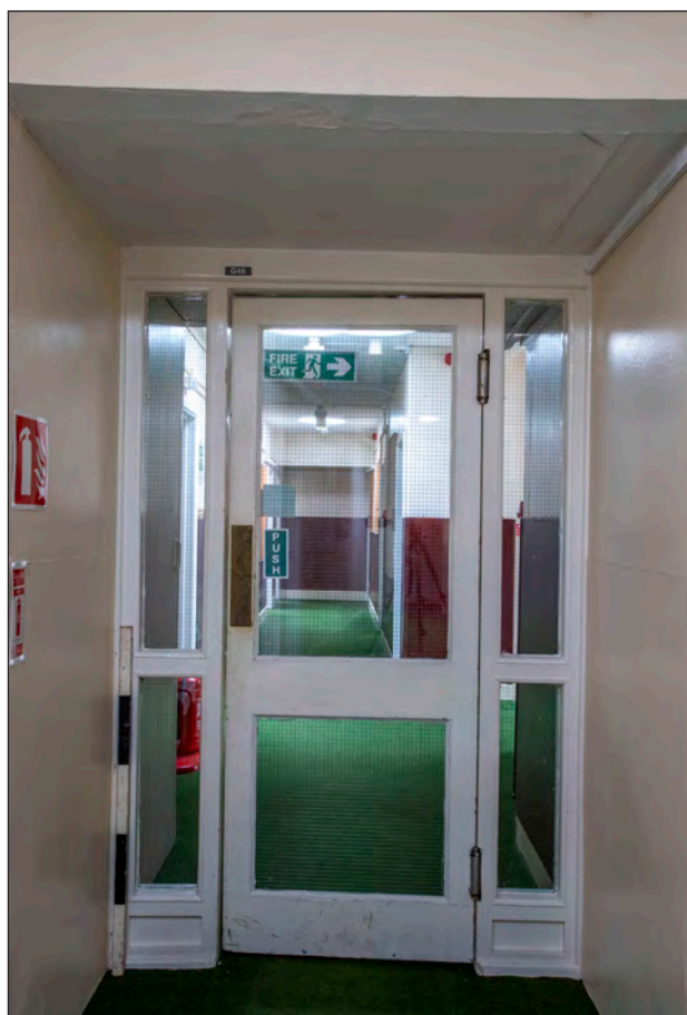
Photograph 21: Building JE 0 060 glazed partition doorway that separates the main corridor into two
