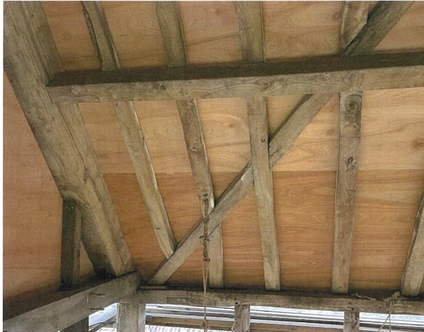
11. Roof Bracing, Purlin & Rafters
