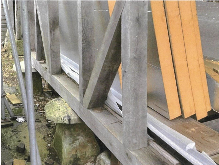
5. Typical Base Frame & Post Connections
