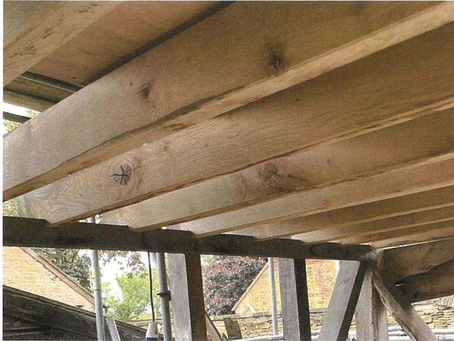
7. Underside of First Floor Structure
