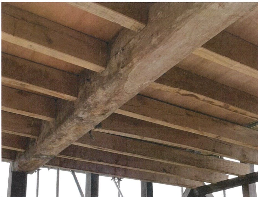
8. First Floor Spine Beam
