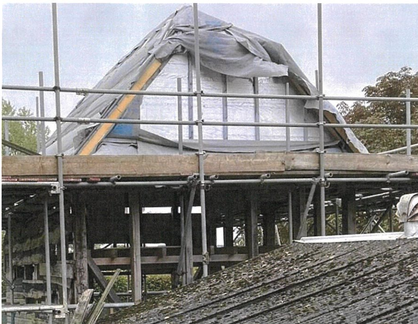
2. West Elevation Showing Gable End
