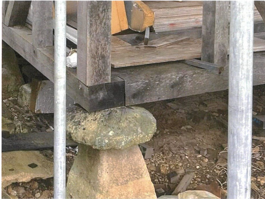
3. Typical Base & Corner Post Bearing
