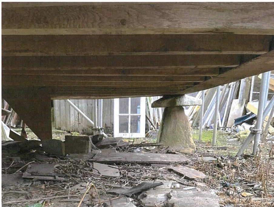
4. View on Underside of Base Framing
