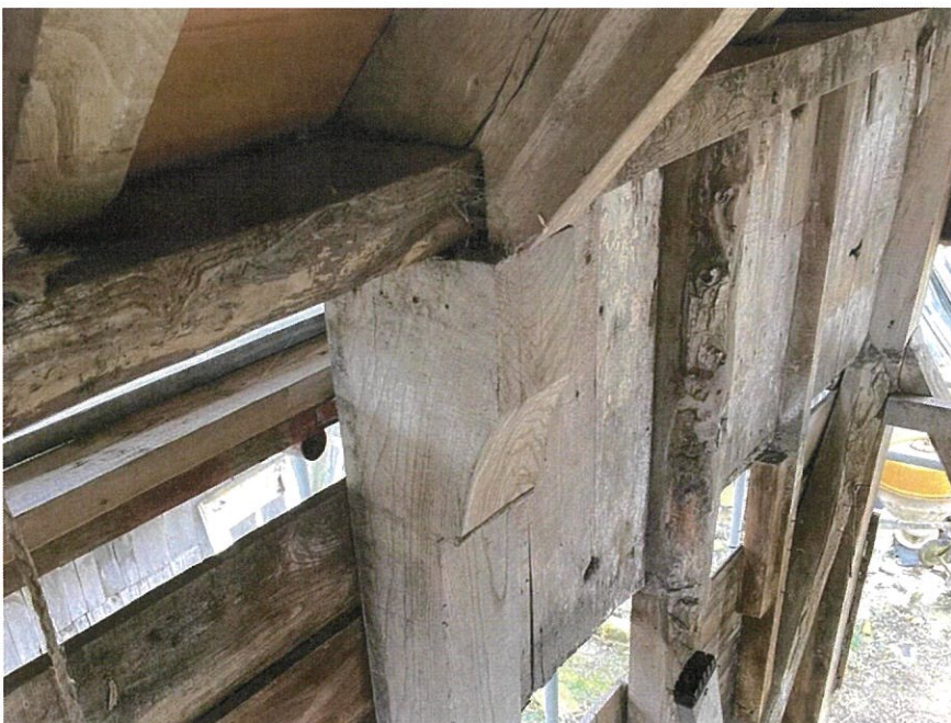
14. Principal Rafter Bearing Detail
