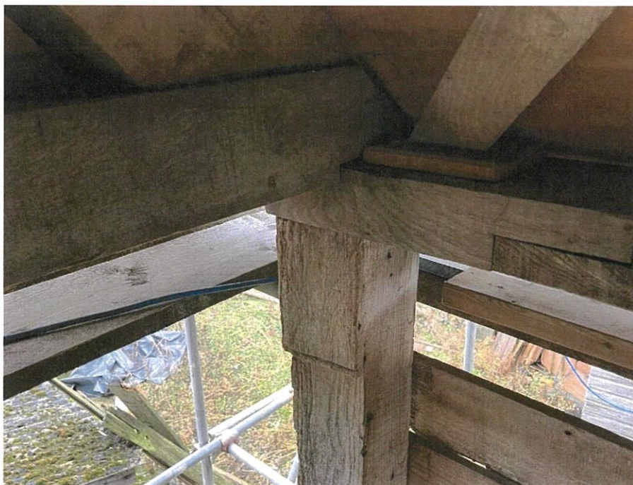
10. Typical Corner Post Head Arrangement
