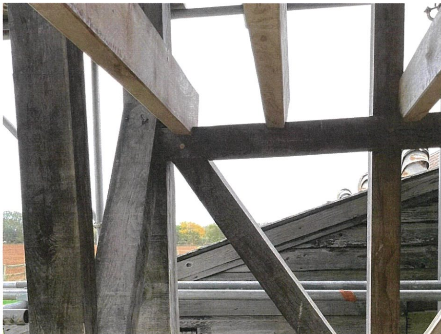
6. First Floor Joists End Bearings
