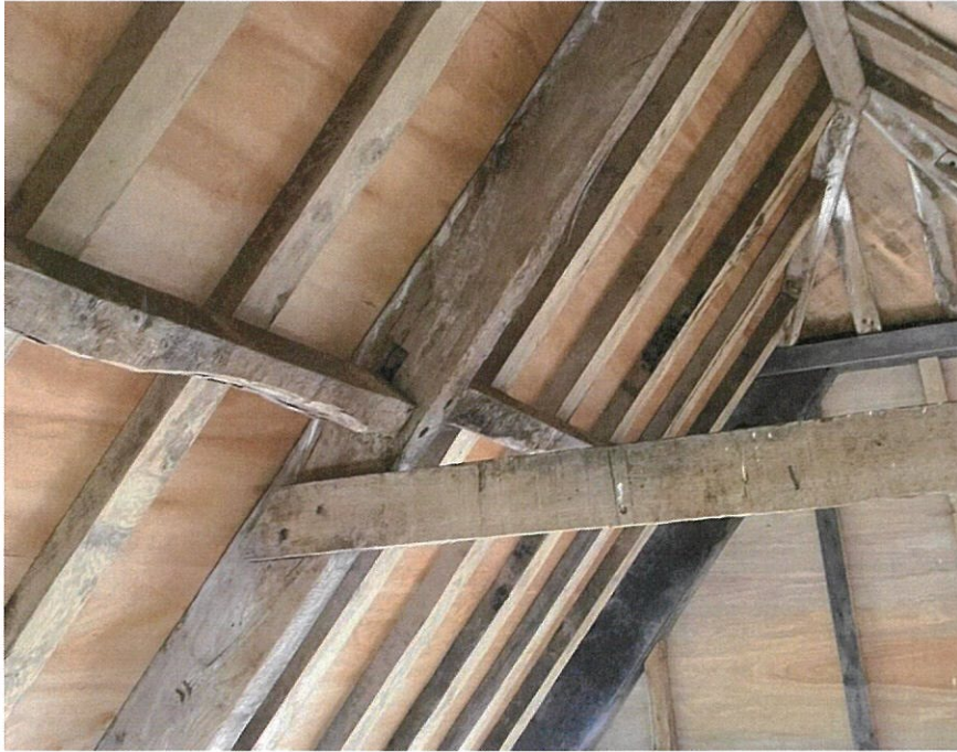
13. Roof Truss, Collar & Purlin Arrangement
