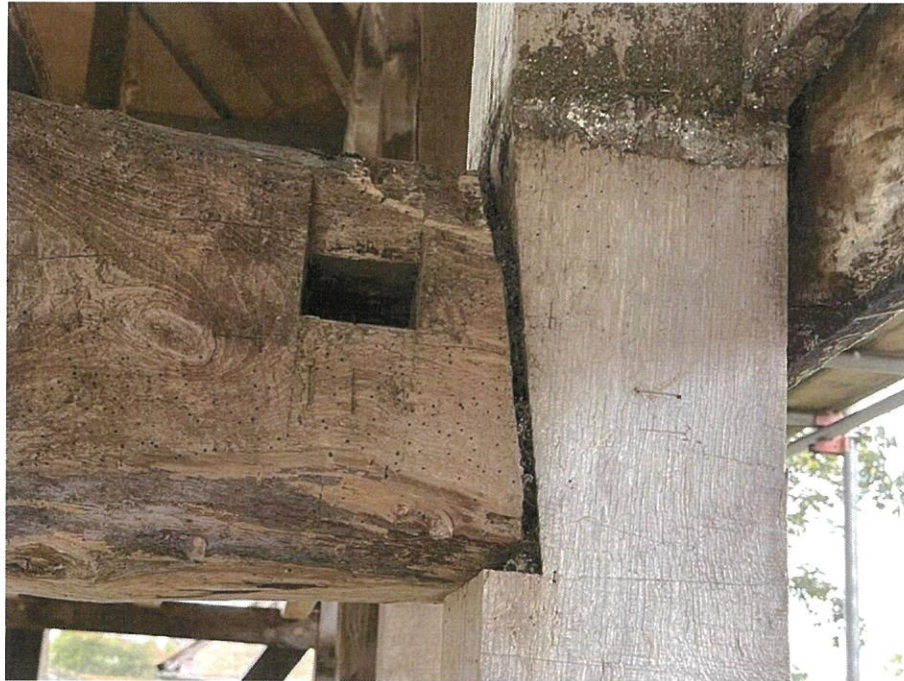
9. Spine Beam Shoulder & Typical Notching
