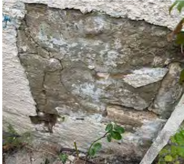
Area of stripped paint to eastern elevation revealing cementitious render beneath.
