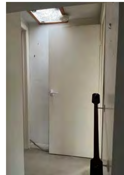
Internal view of first floor Landing | 2025
