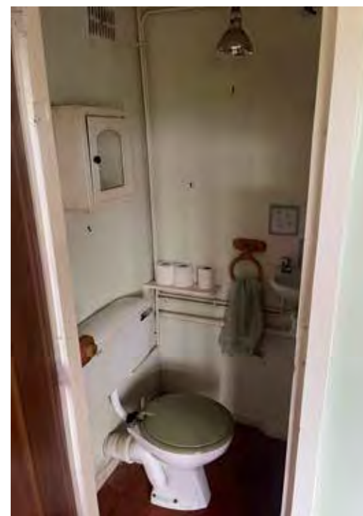
Internal view of Ground Floor WC | 2025
