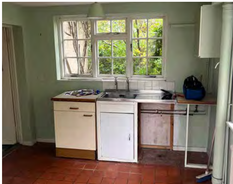
Internal view of Entrance Hall / Utility | 2025
