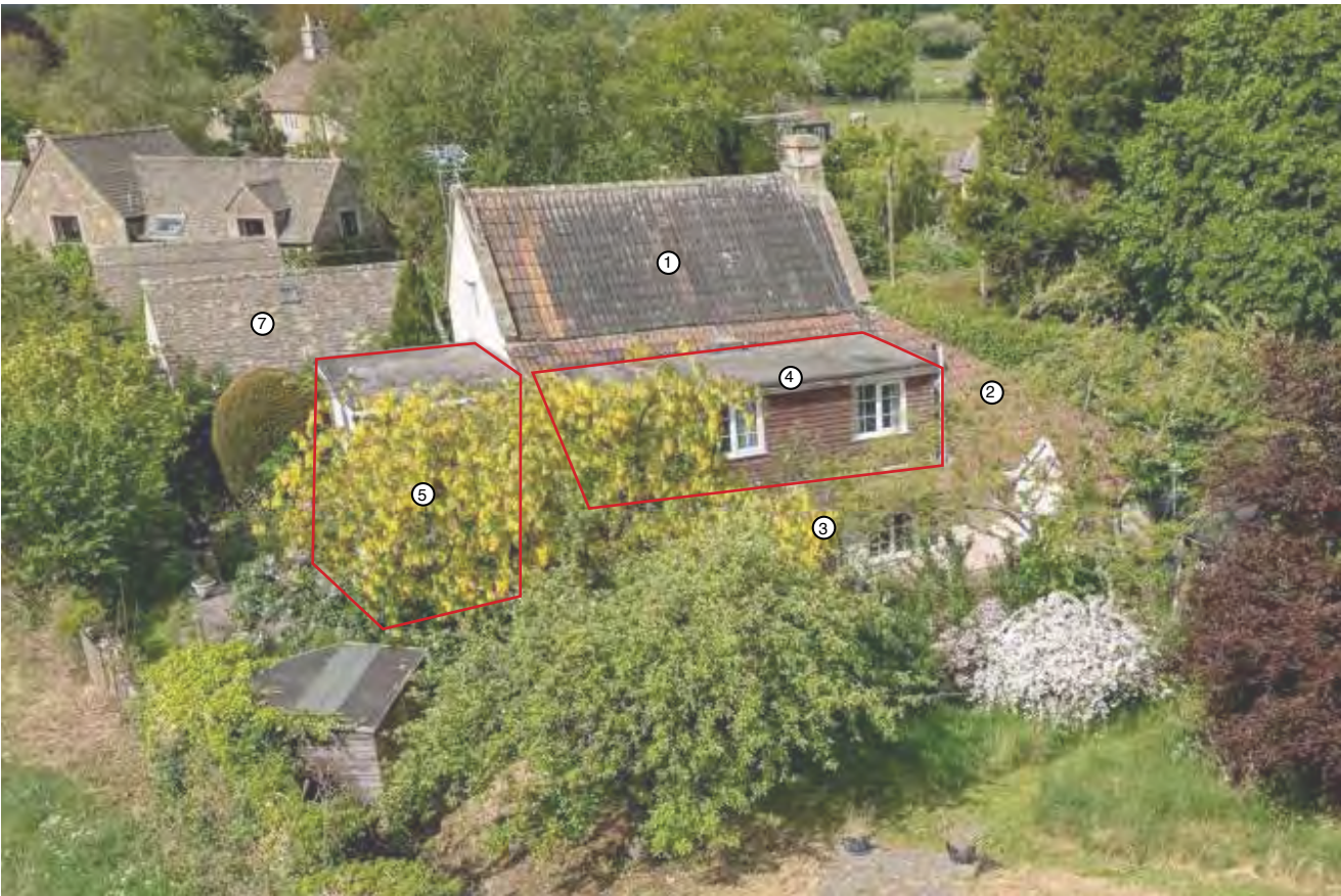
Aerial View - East
