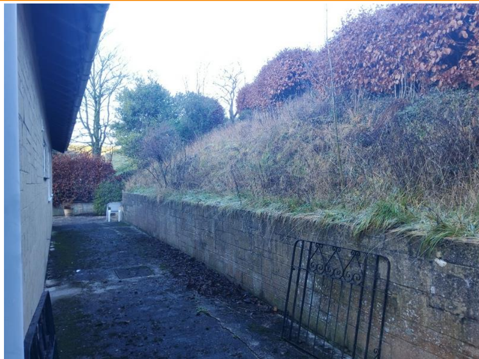
RHS of property located on raised ground.
