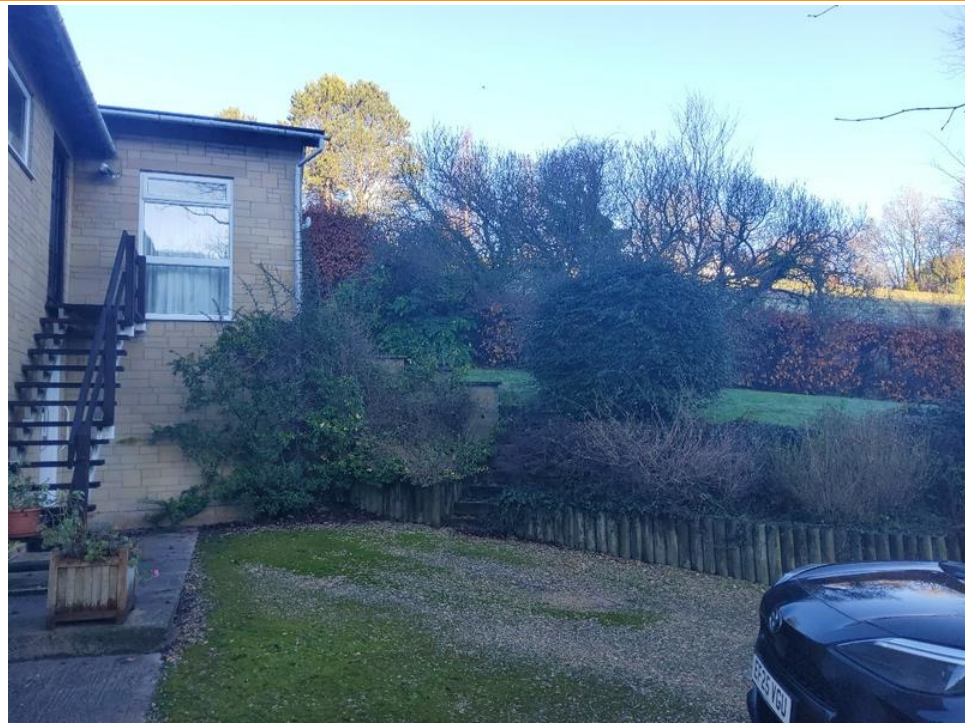
RHS of property located on raised ground.
