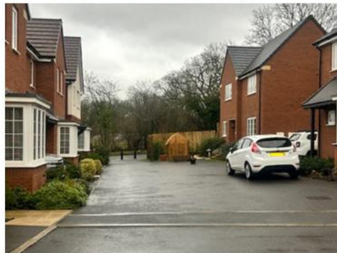
Below: 3 photos from east of the application site:
