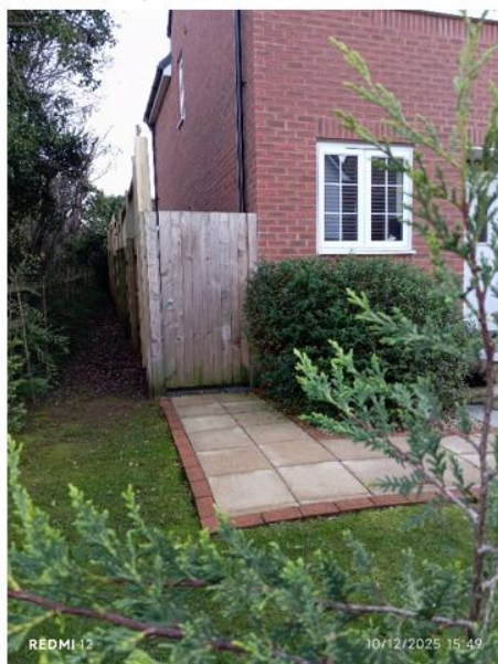
View of fence on eastern boundary from footpath in front of No.8
