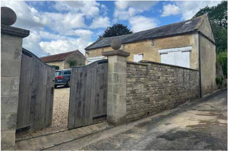
Entrance to the former farmyard from the road. The walls and gates were constructed in the late twentieth century. In the background is the nineteenth-century stable and coach house.
