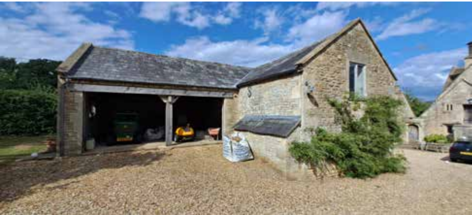
The modern cowshed to the rear of the stables and coach house, now in domestic use.
