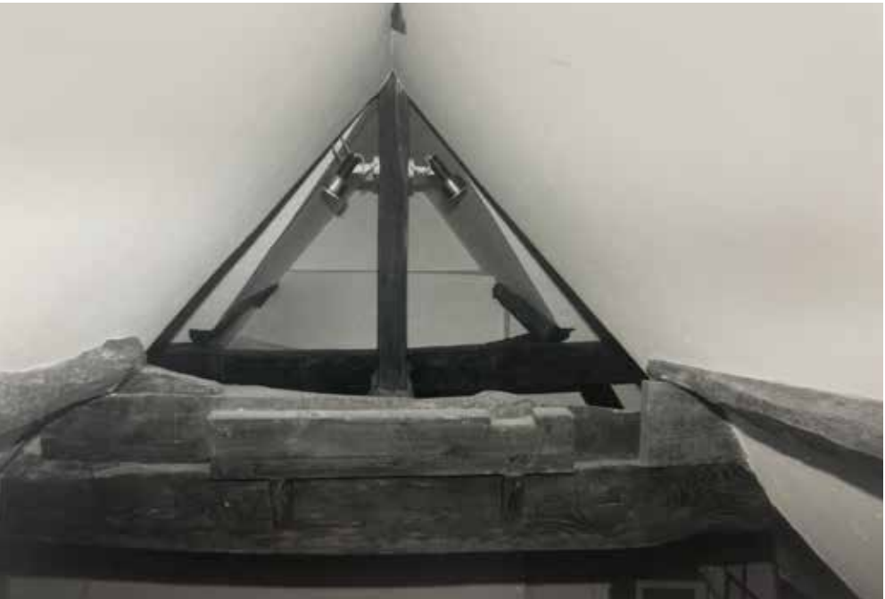
Extended collar trusses within the roof.
