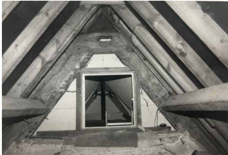
View of the roof space from the south-east.
