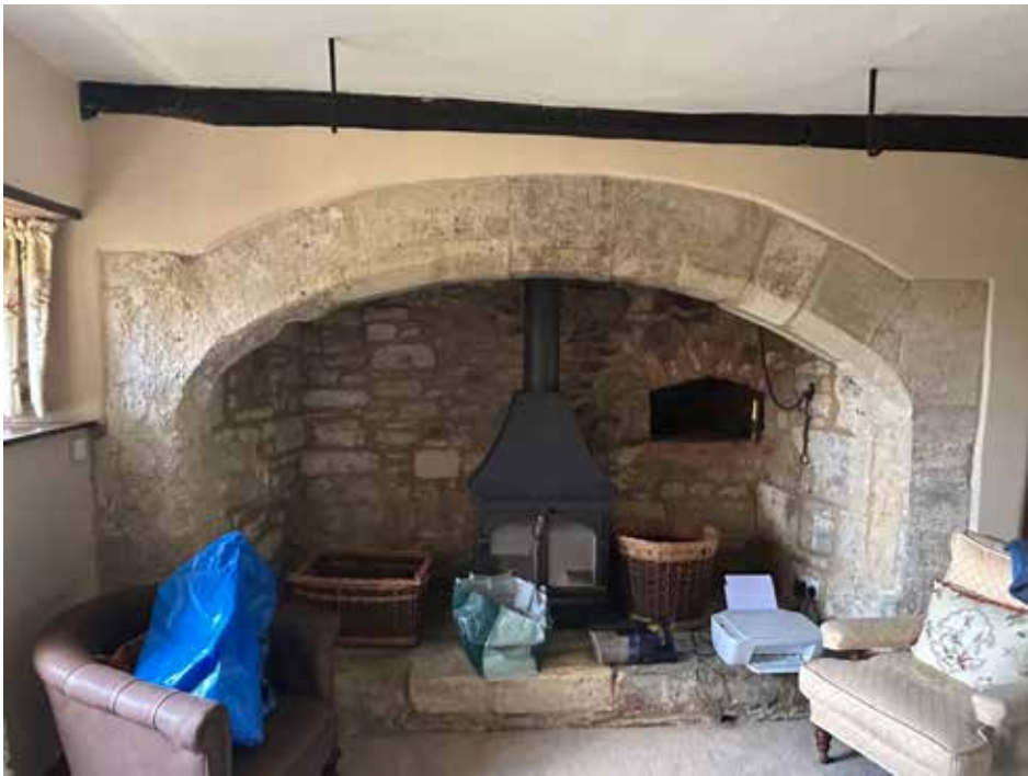
The segmental arched fireplace in the old Kitchen of the house to the west of the existing dining room.
