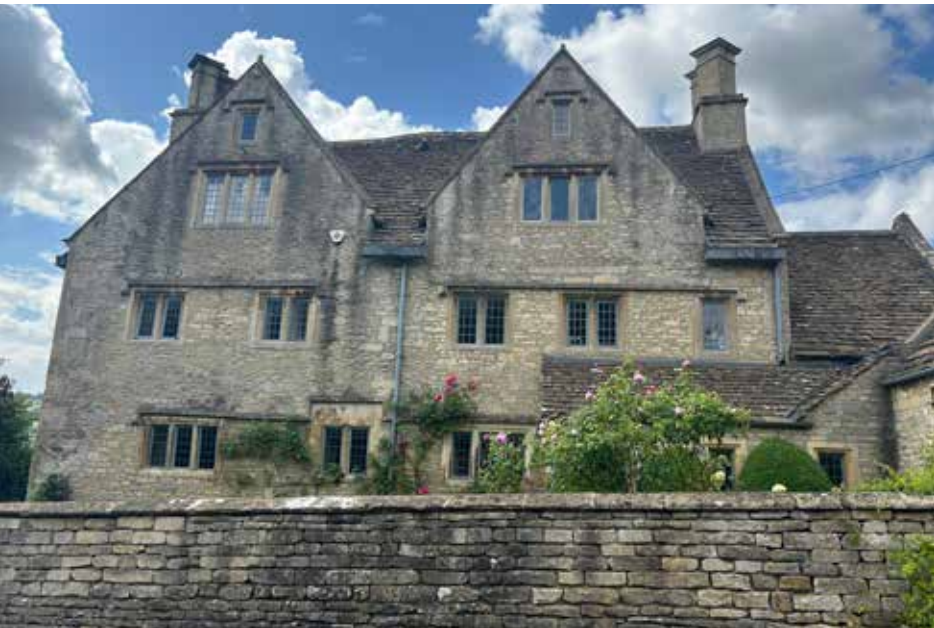
The north-eastern elevation, facing towards the road, thought to be the earliest phase of the building. The north-western elevation faces onto the entrance drive. Adjacent to the access gates is the former outbuilding (now the kitchen). This is attached to the main house by a twentieth-century entrance door and lobby. Adjoining this, at the end of the main house, is a one-and-a-half-storey former agricultural building. The main elevation to the south-west
