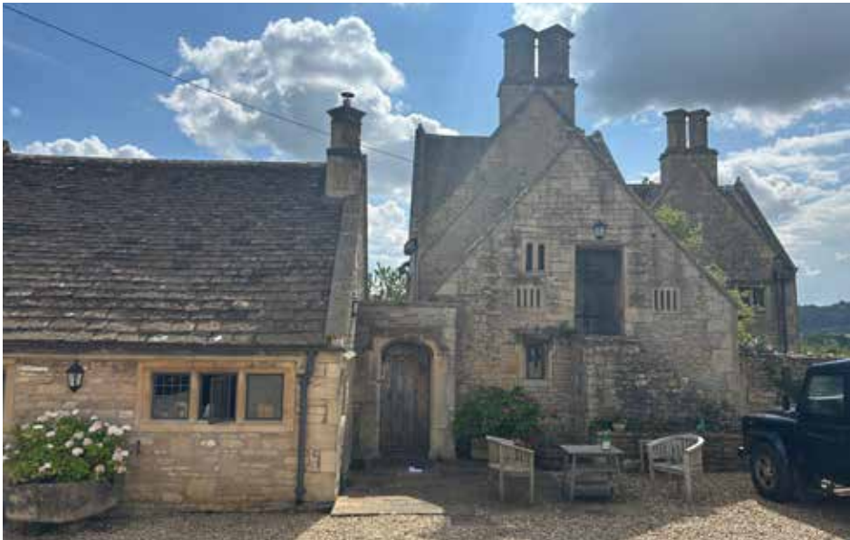
Modern view of the western side of the house, with the doorway and lobby created by Morley to link the main house and the outbuilding to the north.
