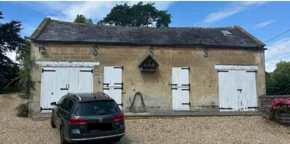
The south-eastern elevation of the nineteenth-century stable and coach house, adjacent to the boundary with the road. This building is now in domestic use.
