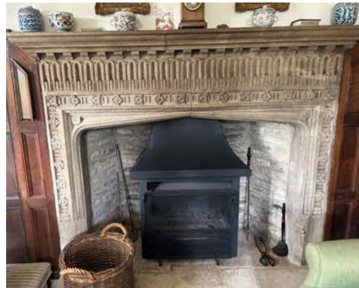
Left: The existing fire surround in the parlour. This is a modern replacement of the original that was recorded in the space in Herbert Hall's drawings of the early 20th century.
