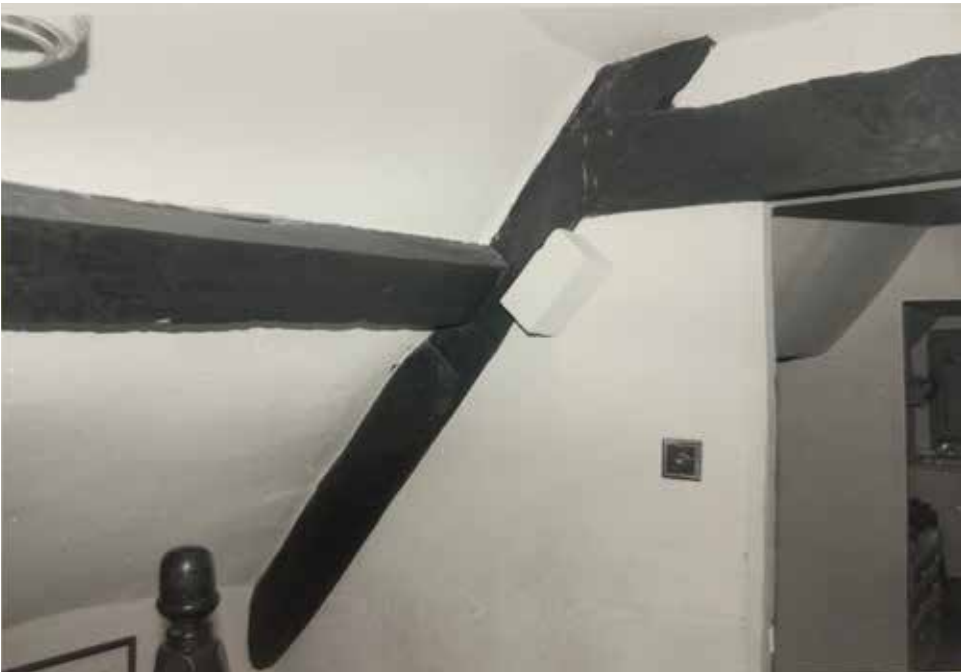
Internal view of the roof over the staircase.
