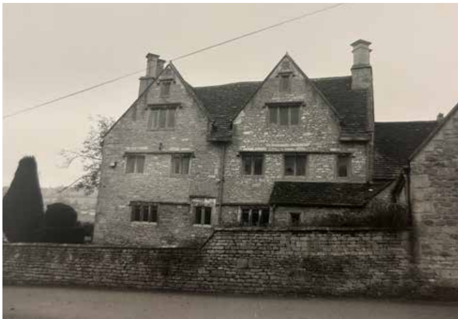
Additional view of the north-eastern elevation from the road.
