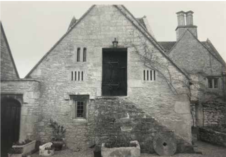
Additional view of the former agricultural building on the north-western elevation
