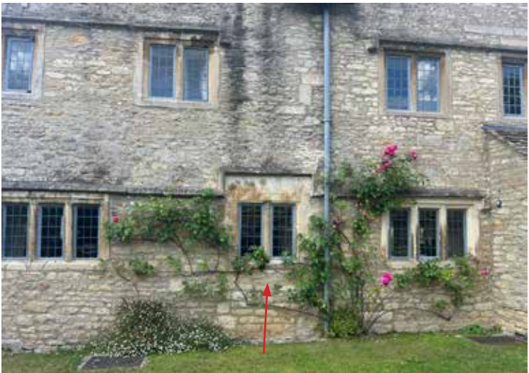
Left: Modern photo showing the blocked doorway on the north-eastern front, now a window to the hall.
