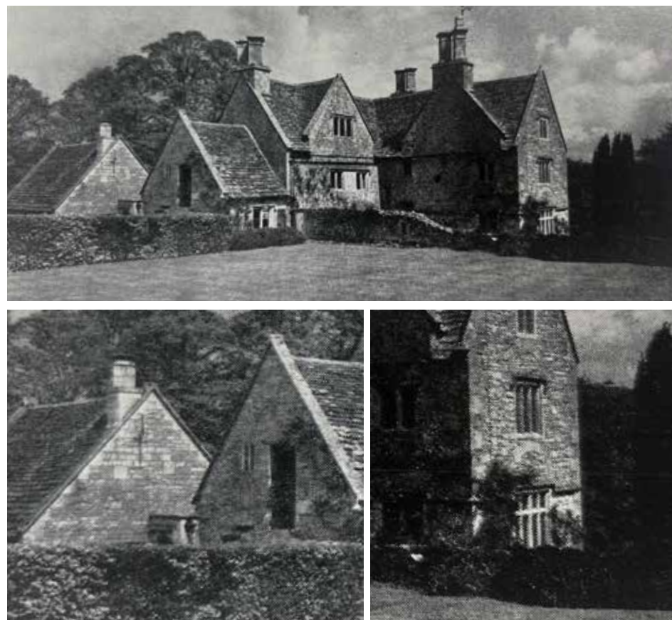
Photograph from the 1972 sales advert (top) showing some of the changes made by Robert Morley. The photo confirms that Morley created the lobby and new door between the outbuilding and main house (see inset detail, left). It also shows that the existing window had been installed into the parlour, replacing the one shown in Herbert Hall's drawing (see inset detail, right).
