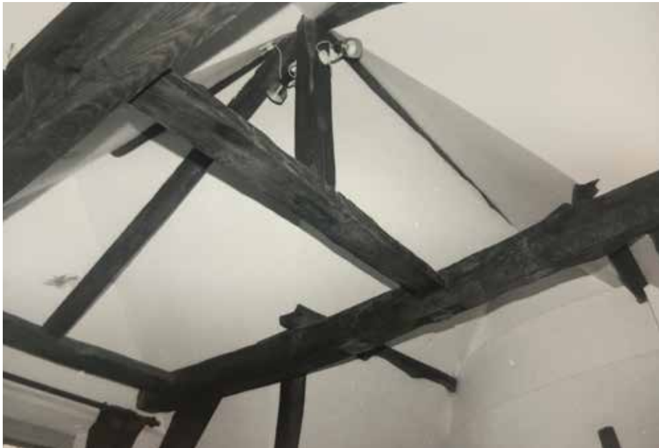
Extended collar trusses within the roof.
