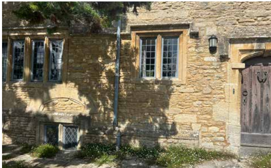
Detail of the south-eastern facade showing the plinth around the parlour wing that stops at the junction with the earlier range.
