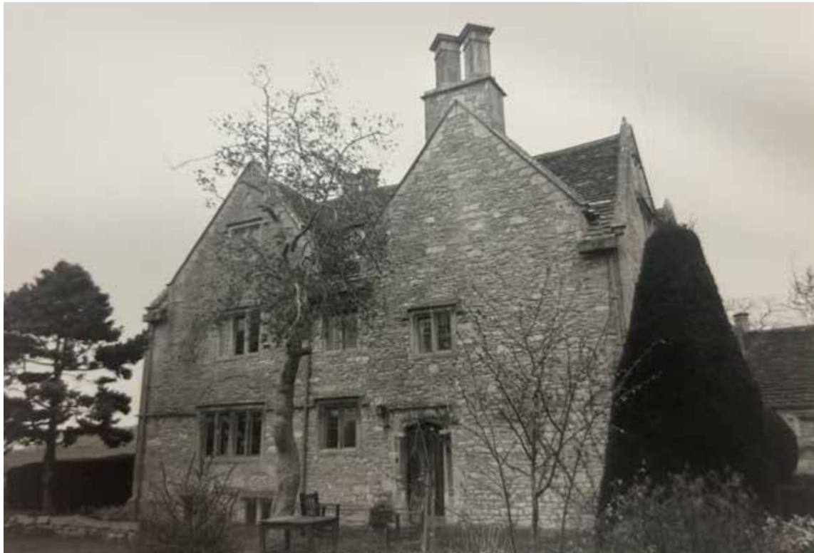
View of the south-eastern elevation from the garden.
