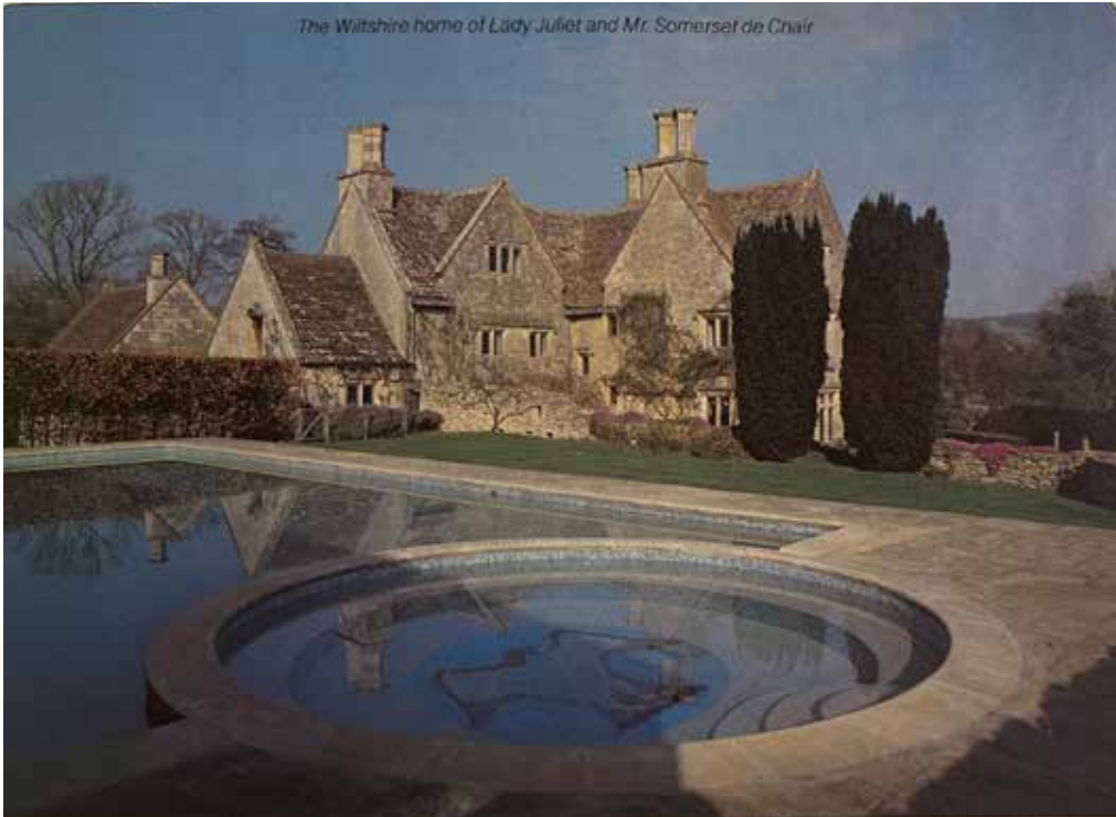
View across the gardens showing the swimming pool installed by Lady Juliet de Chair
