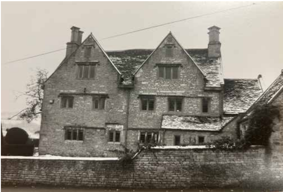
View of the north-eastern elevation from the road.
