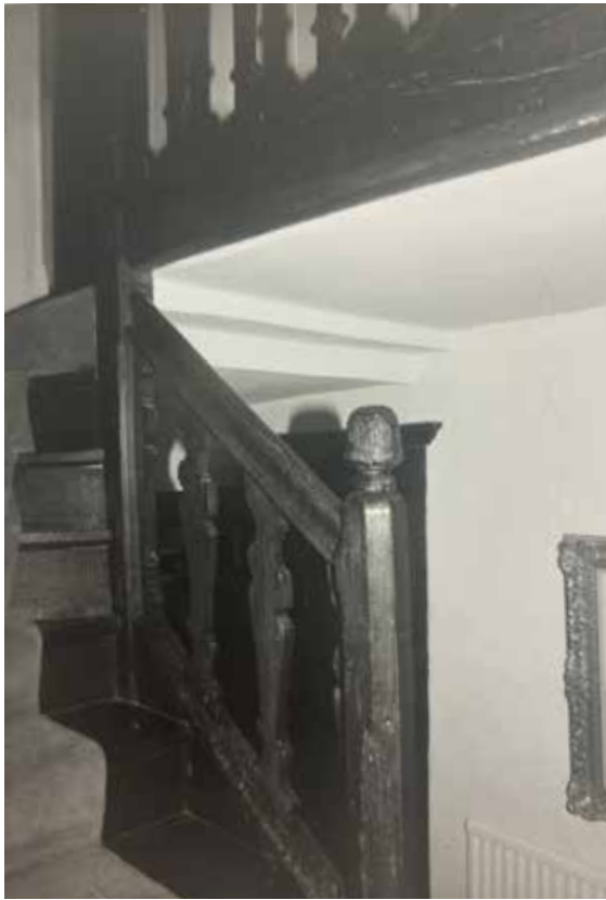
Interior detail of the staircase at first floor level.
