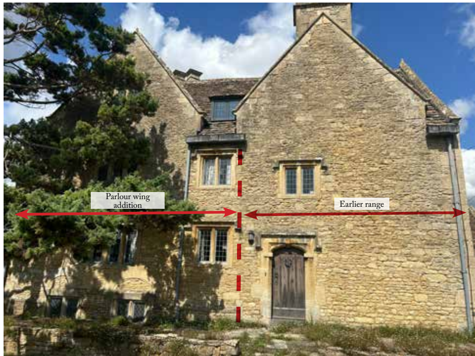
Modern photo of the south-eastern facade showing the end gable of the slightly earlier, north-eastern range to the right, and the parlour wing addition of c.1645 to the left.
