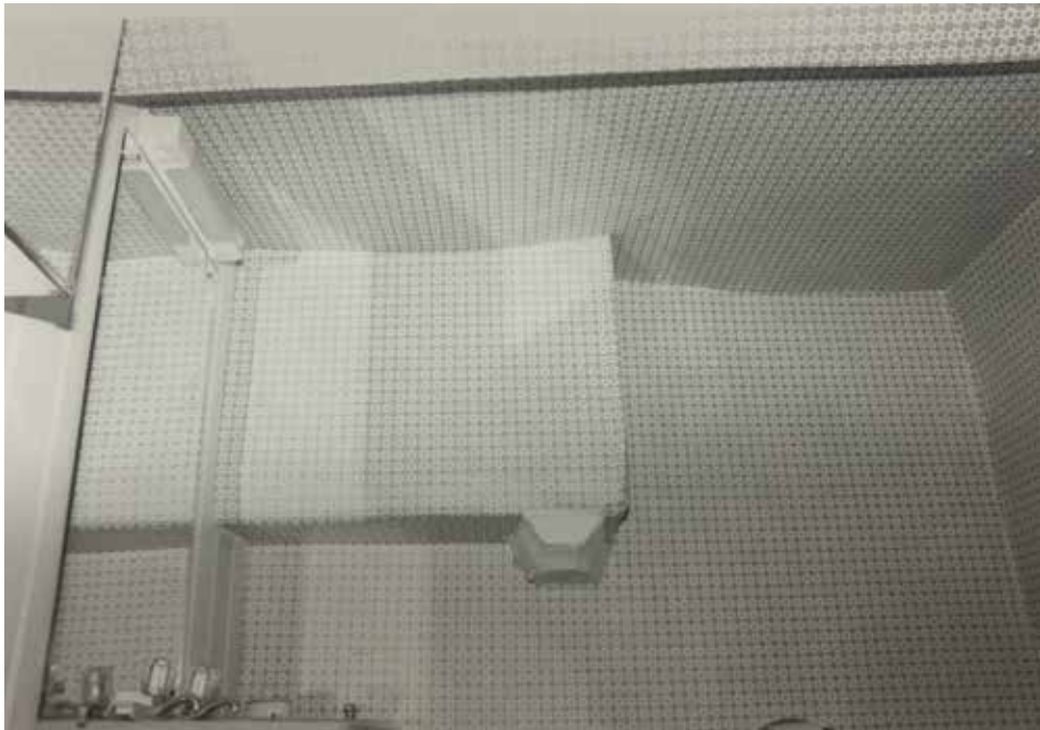
Internal view of the chimney stack at first floor level on the south-eastern wall.
