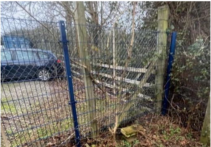
Existing fence around boundary of site
