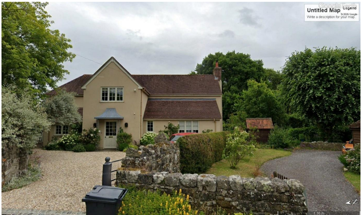
Fig.2 Front elevation to Church Hill
