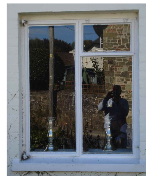
Window W2 (single glazed in metal casements)
