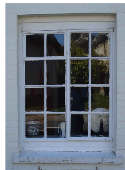
Window W1 (single glazed in metal casements with glazing bars)
