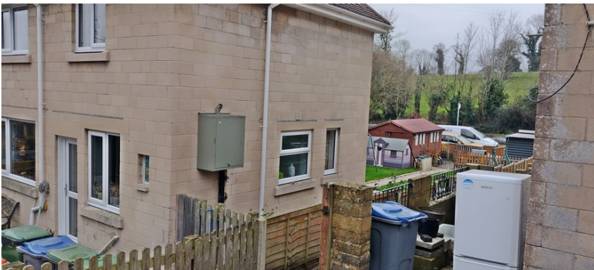
Side wall of 3, Snow Hill, from rear
