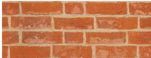
York Lindum hand made clay bricks laid in flemish garden wall bond with rubbed white cement pointing
