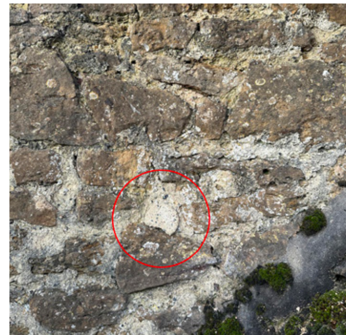
Proposed mortar sample held against existing
