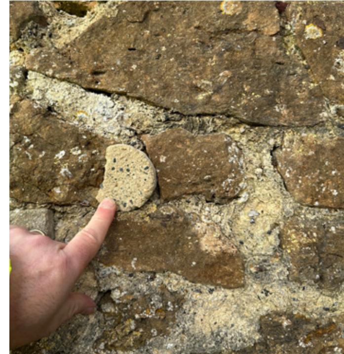
Proposed mortar sample held against existing
