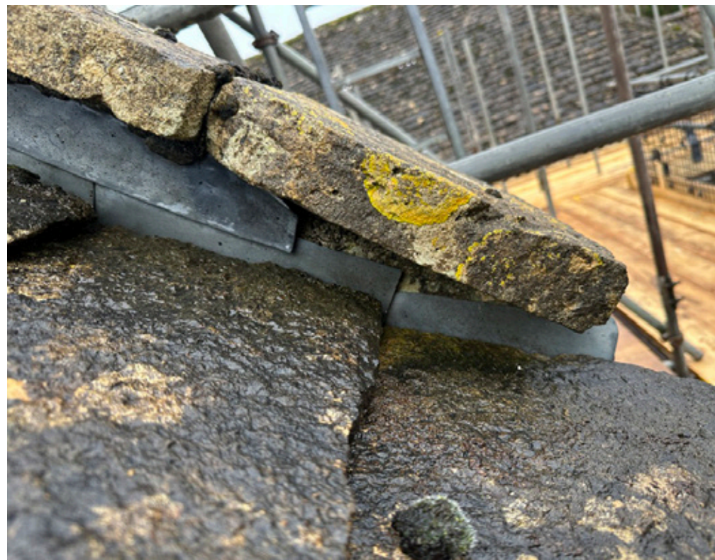
East gable - view from west
