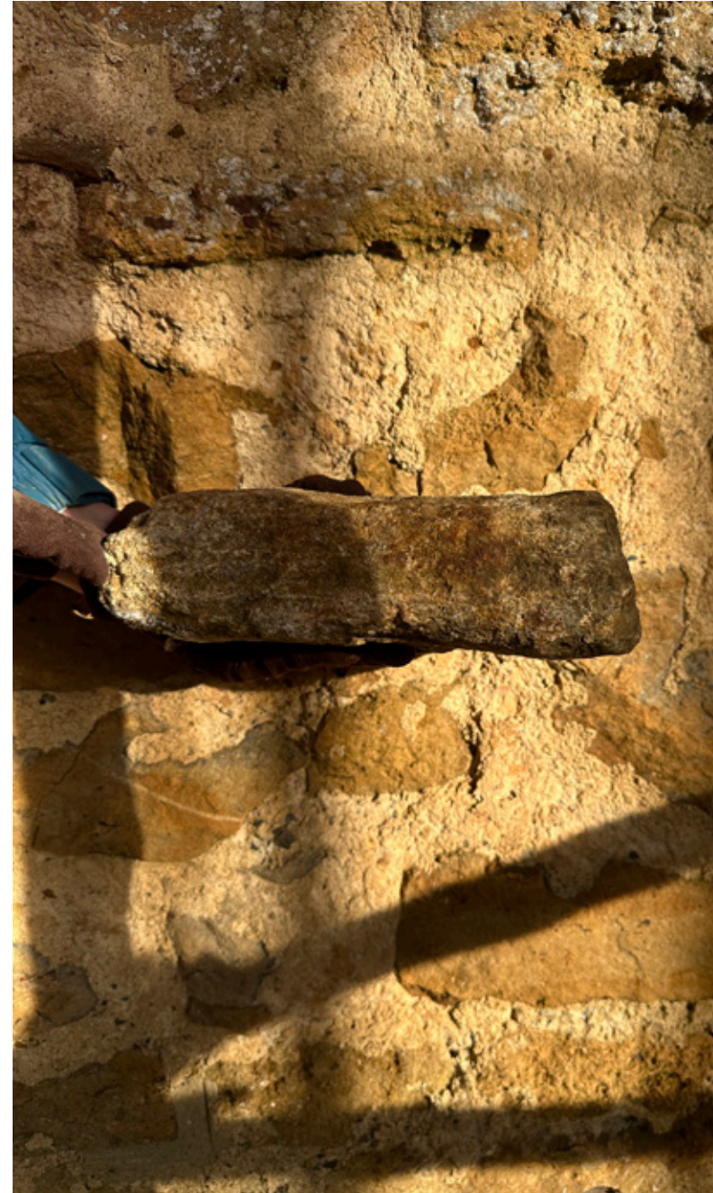
3. Samples held up to existing wall to demonstrate colour match
