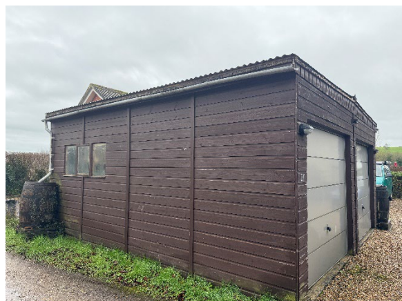
North elevation of B2 (Garage Building)
