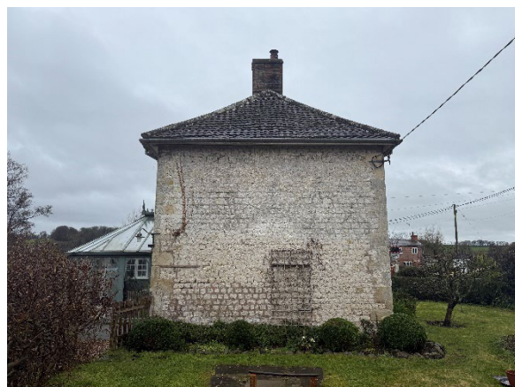
Northern elevation of B1, facing South
