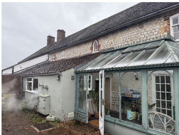
Rear of B1 – SE Elevation
