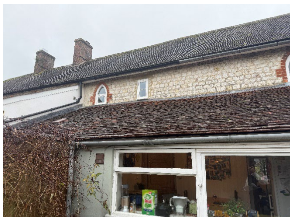
South-East Elevation of B1 facing West
