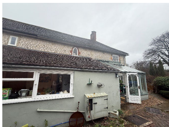
South-East Elevation of B1 facing East
