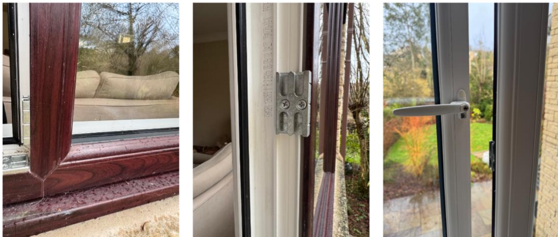
Figure 12 - Photos of materials from existing windows
