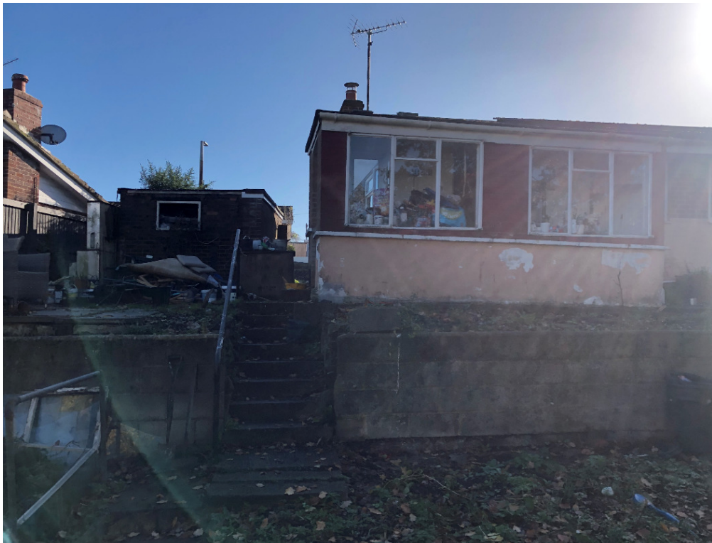
Image 4 –North Elevation (Rear) & Garage - As Existing
