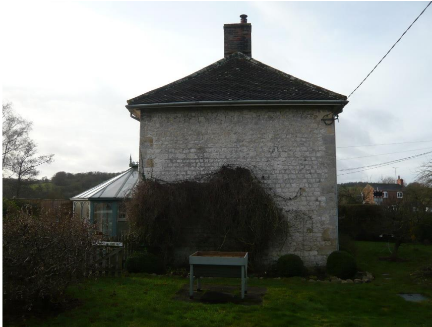
Fig.18 View from within the side garden of the cottage
