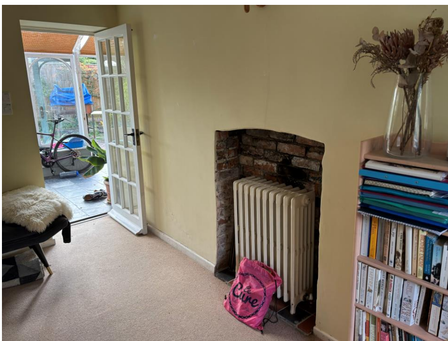
Fig.9 Dining Room with modern glazed doors into the conservatory. Note, back of the Living Room fireplace hollowed out to accommodate a radiator
