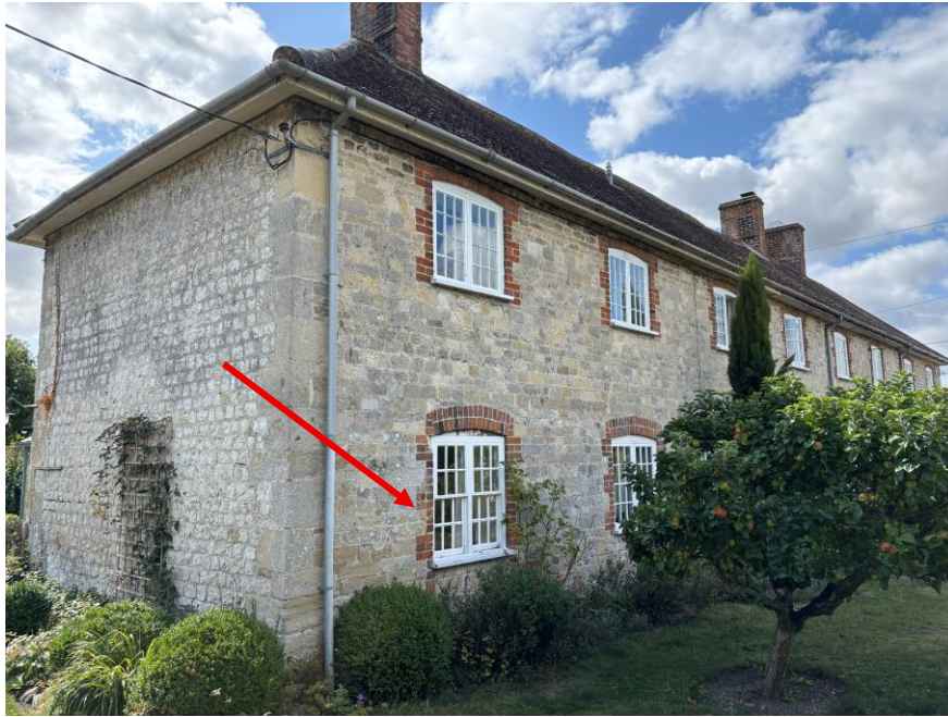
Fig.17 Northern end of the cottage – former door opening highlighted
