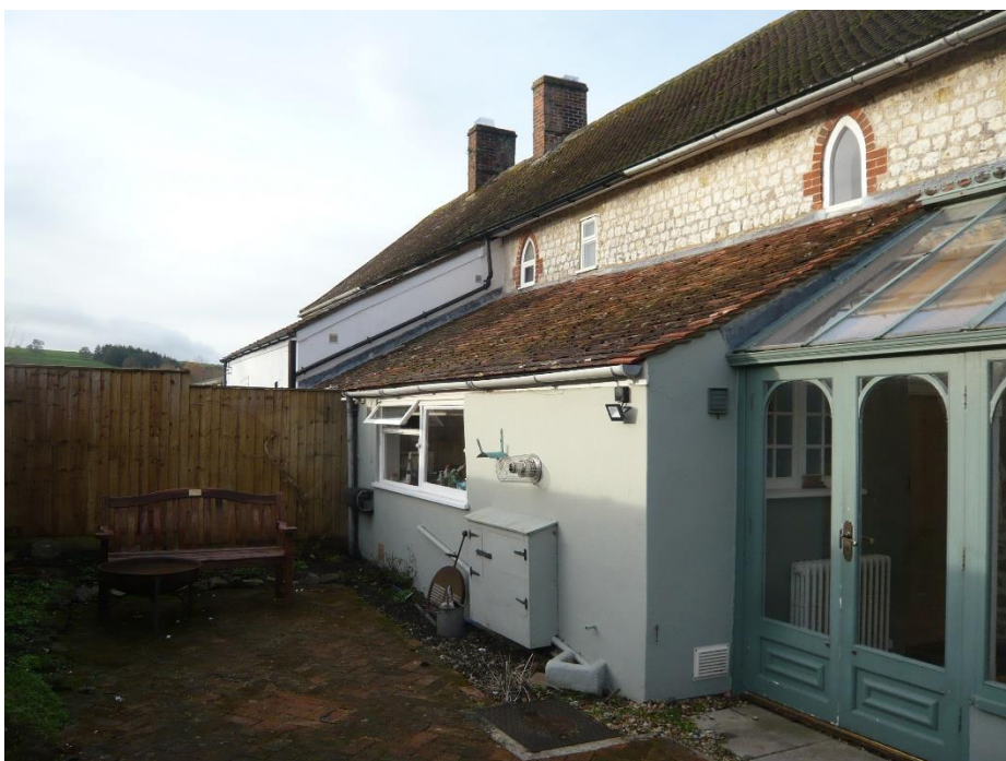
Fig.4 Backs of the cottages with various additions and lancet windows under the eaves
