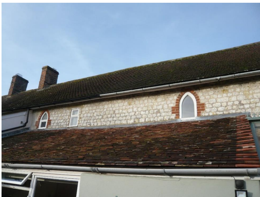
Fig.20 Lancet windows – the one on the right belongs to Corton Glebe Cottage
