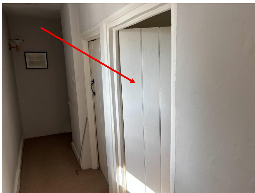
Fig.21 Door to the bedroom
