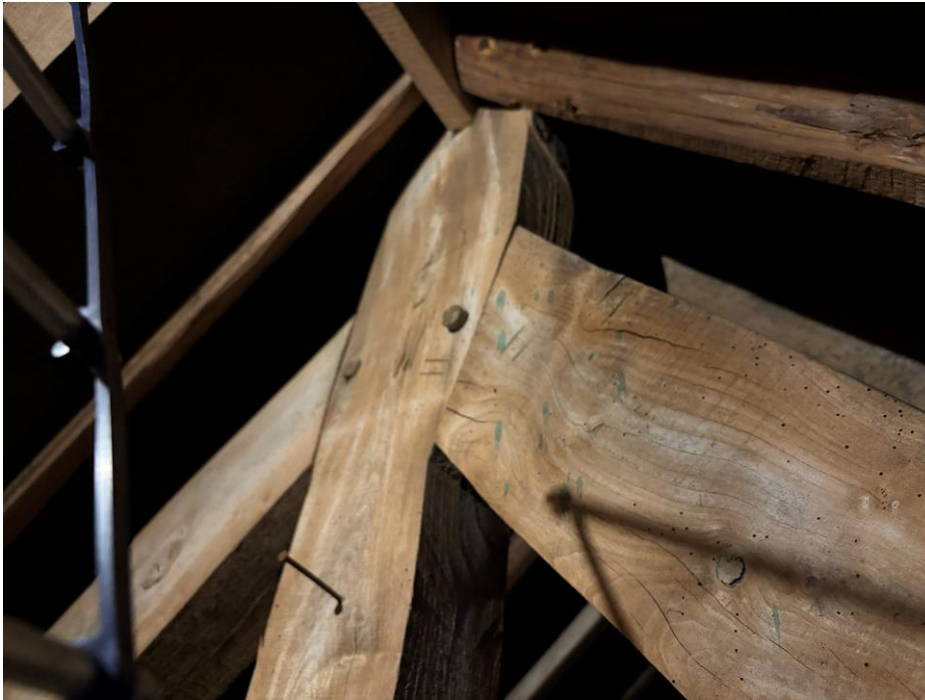
Fig.12 Apex of one of the king-post trusses in the attic
