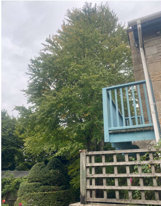
Katsura. Again this tree is far too big in its location next to the house. Fell
