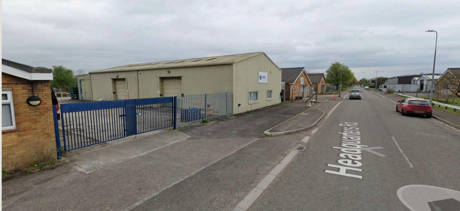
Fig 01: View North along headquarters Road
