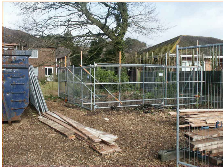
Image 1: Scaffold and Heras panels can provide standard protection that is fit for purpose.
