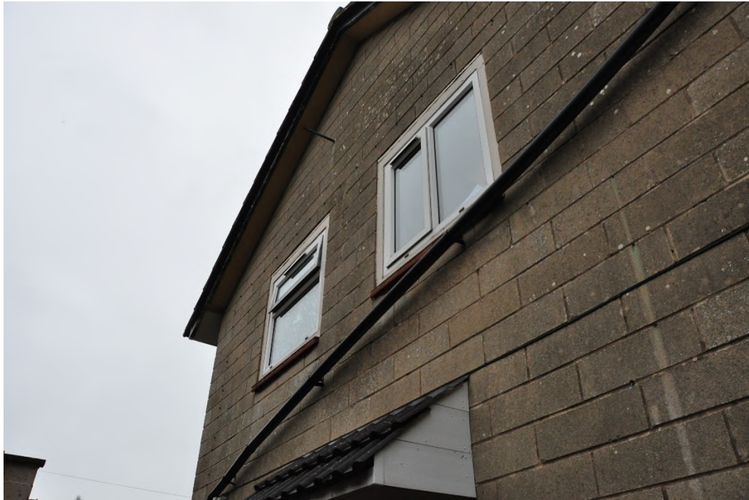
Plate 7 main house west side negligible potential for birds or bats
