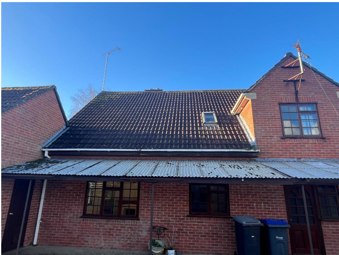
Figure 5. Southern elevations looking northwest
