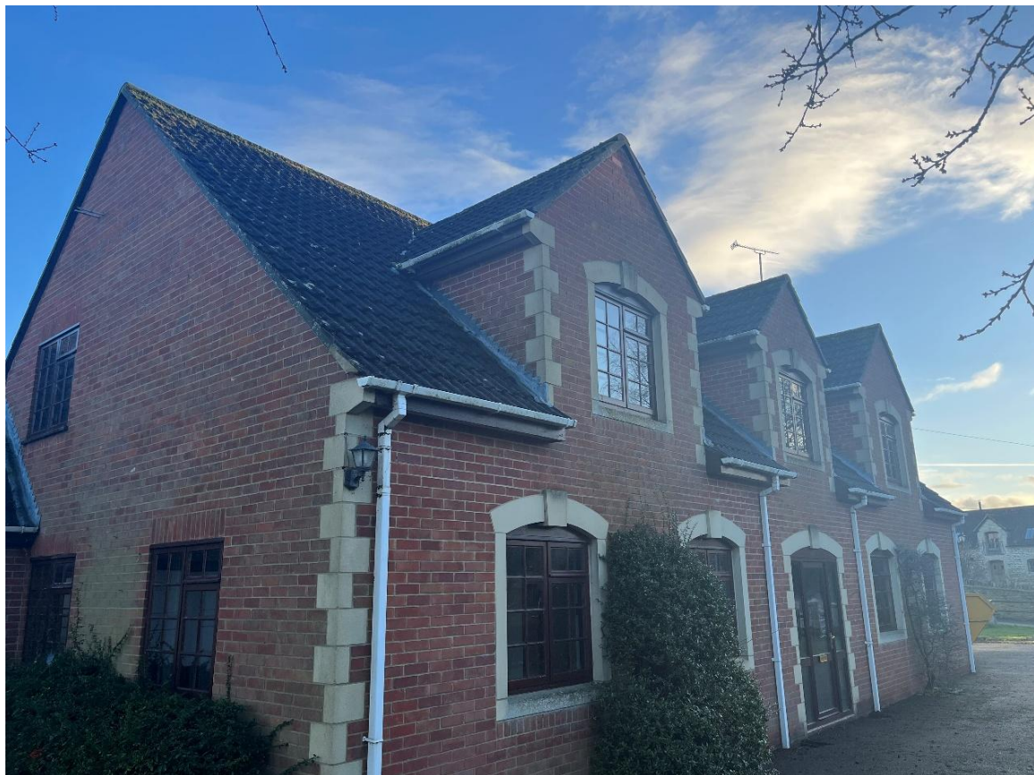
Figure 3. Eastern and northern elevations looking east
