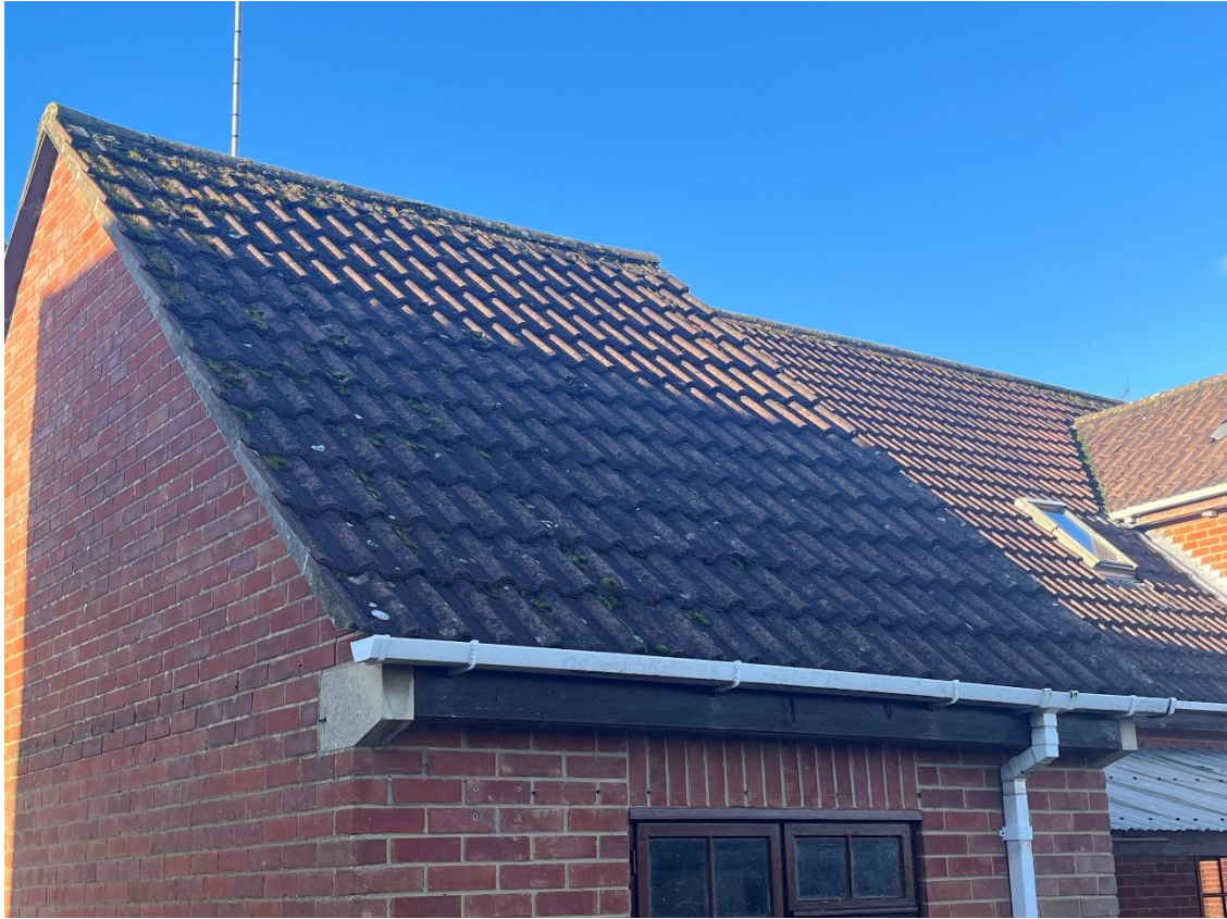
Figure 4. Western gable and western third of rear elevations looking north
