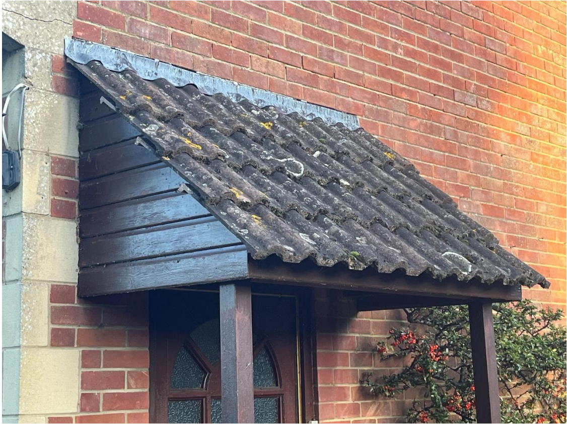
Figure 6. House west gable entrance porch area looking southeast
