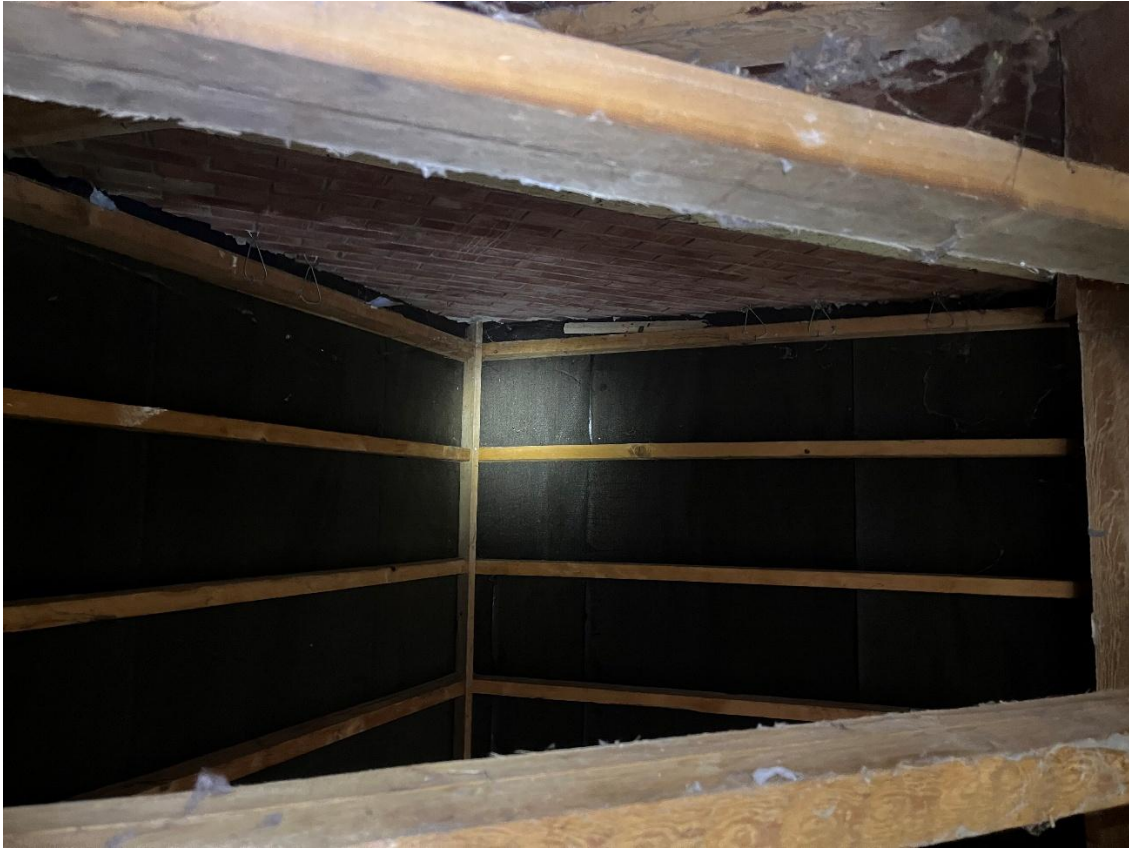
Figure 8. House loft below east gable.
