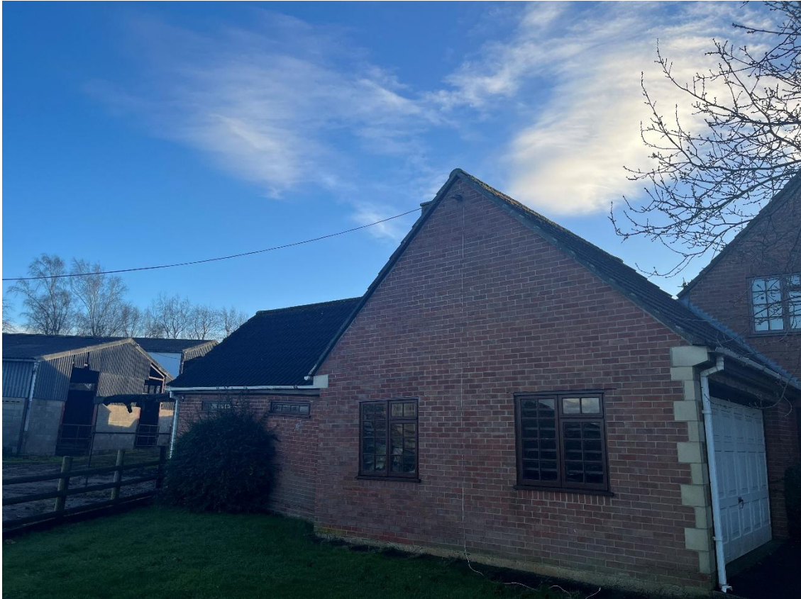
Figure 11. Garage east gable looking southwest
