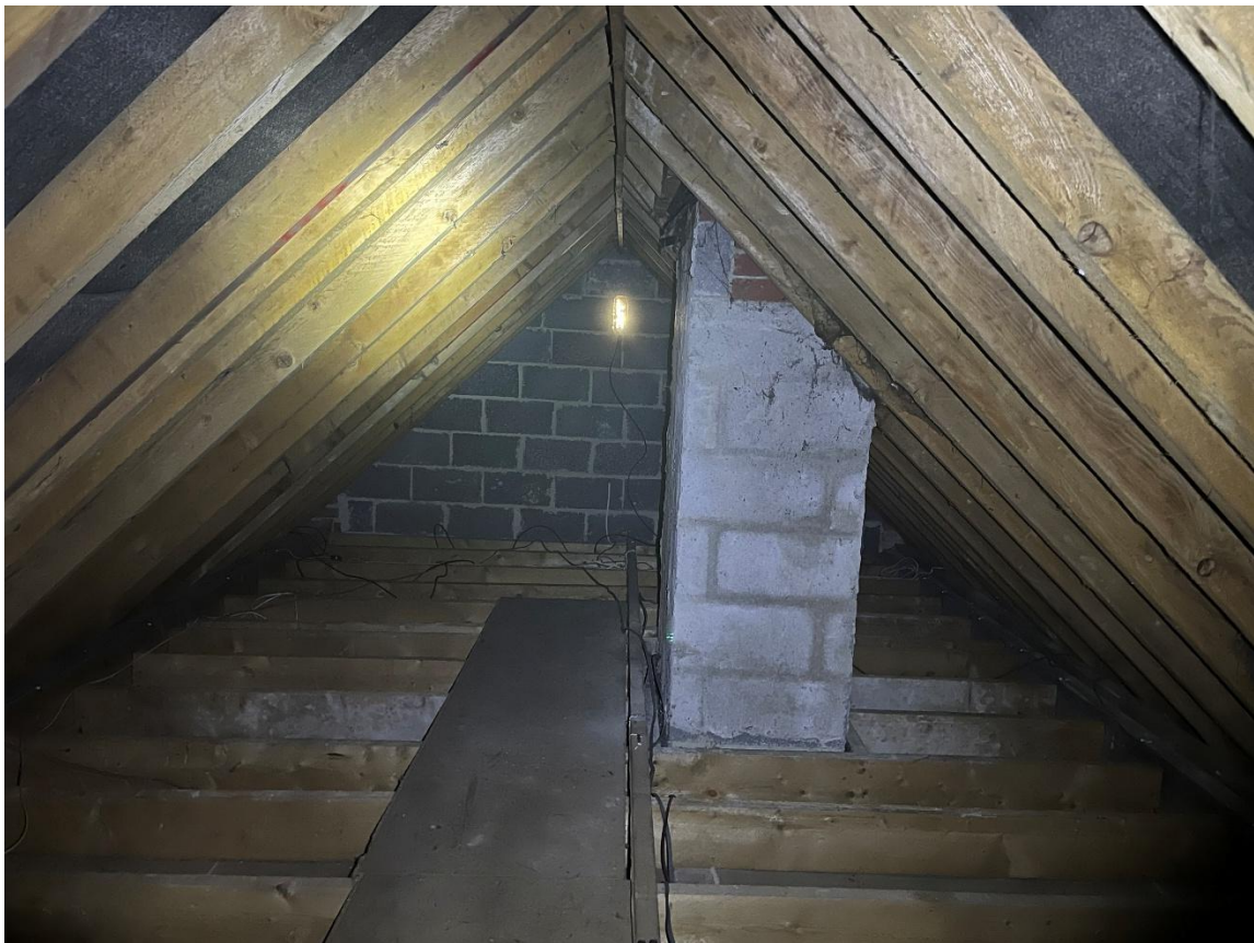
Figure 7. House loft looking southwest.
