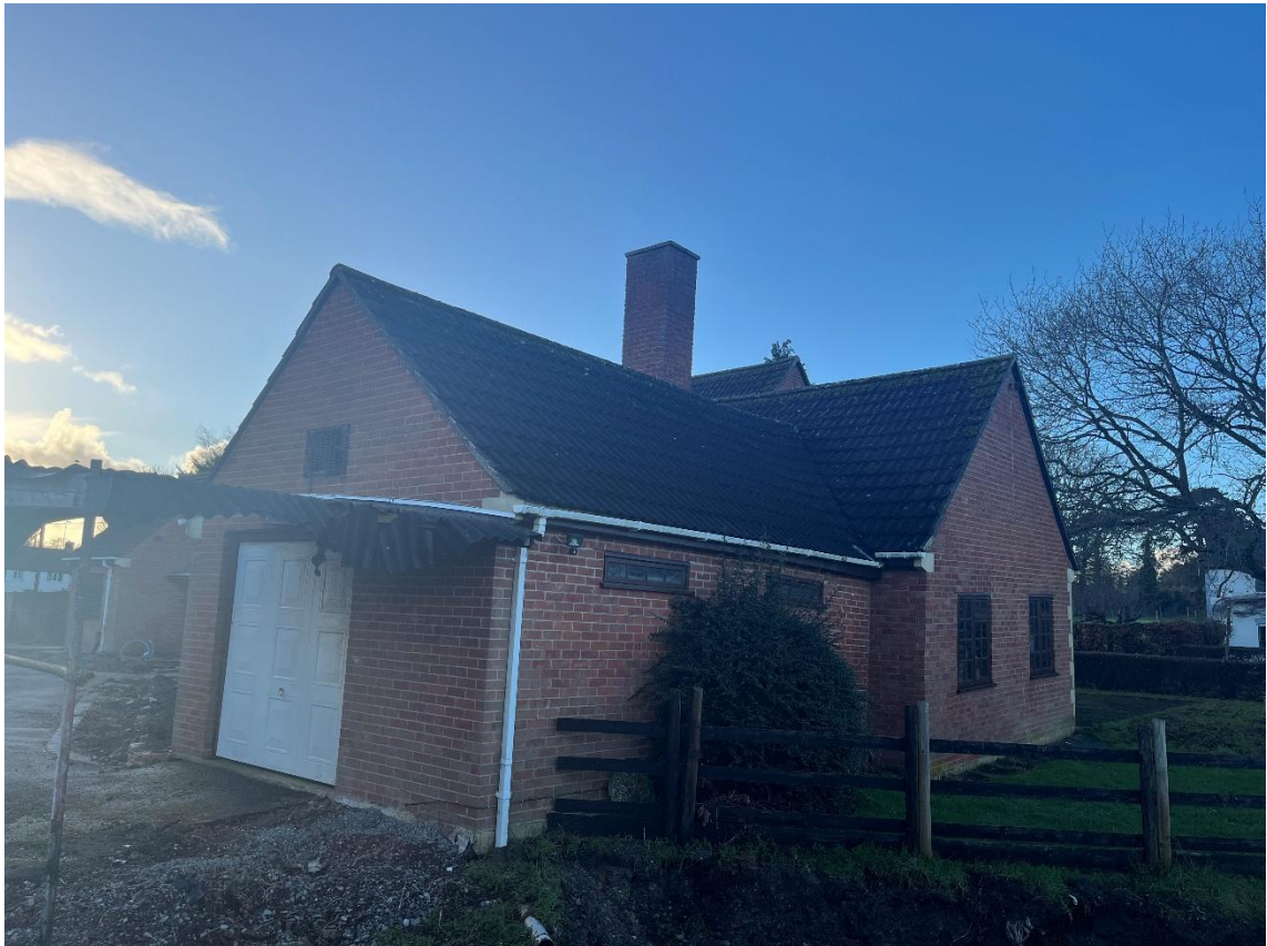
Figure 10. Garage looking northwest
