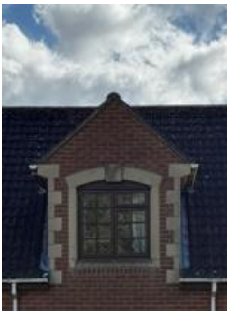
Figure 10 - Existing central front dormer
