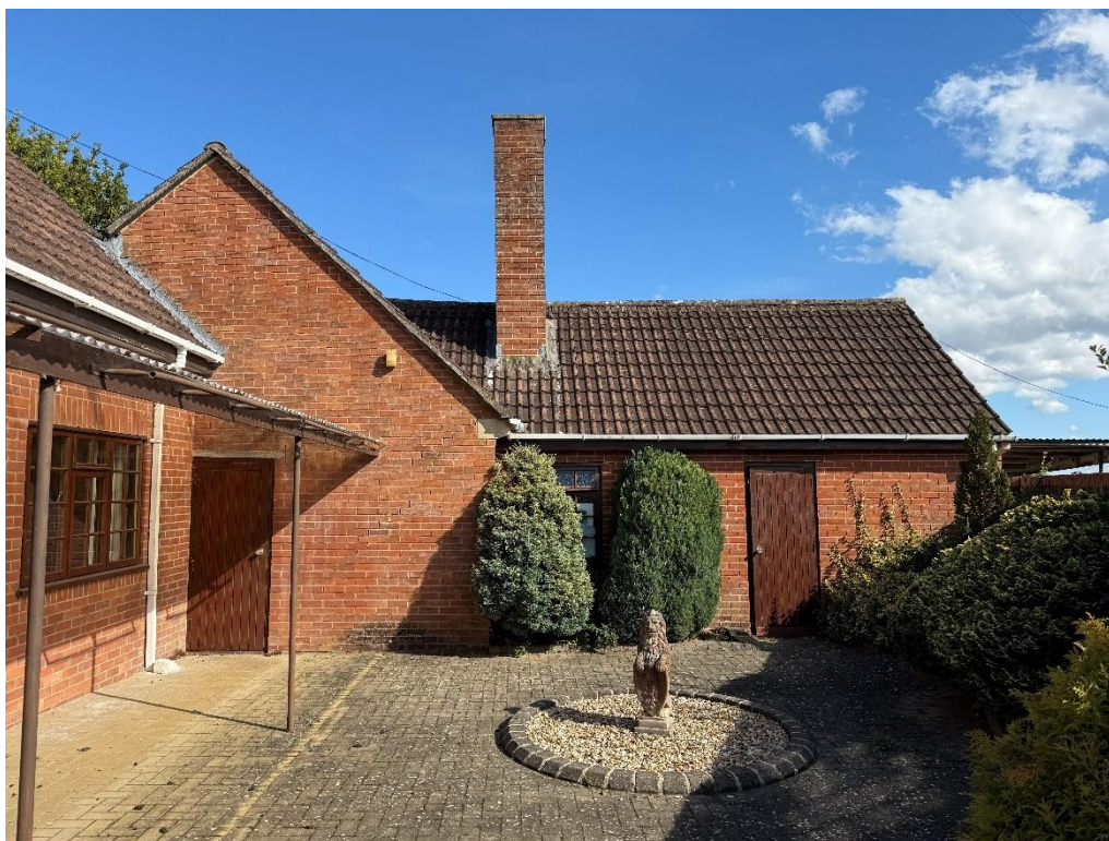
Figure 8 - Existing garages and chimney stack to be demolished
