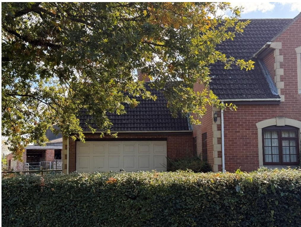
Figure 13 - View from Main Street, showing garages to be removed
