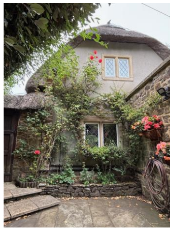
Kitchen window referred to rear south west
