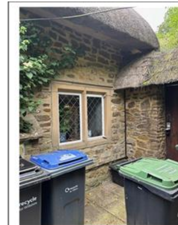
Side south east Kitchen window referred to
