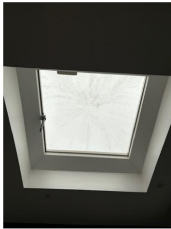
Bathroom rooflight internal view
