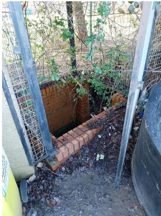
Image 3.1 – Access to Existing Concrete Headwall
