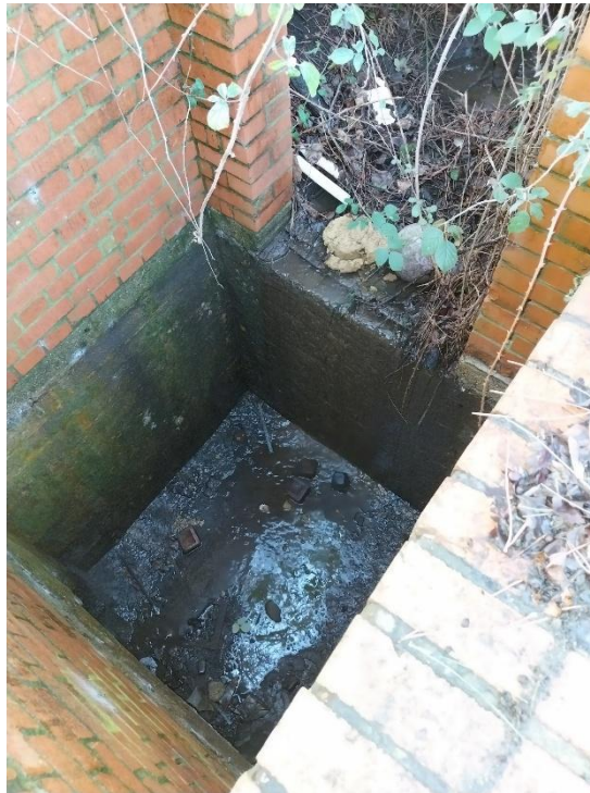
Image 3.2 –Existing Concrete Headwall
