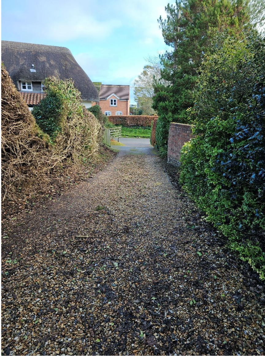
Figure 6 –Main vehicular access off the lane
