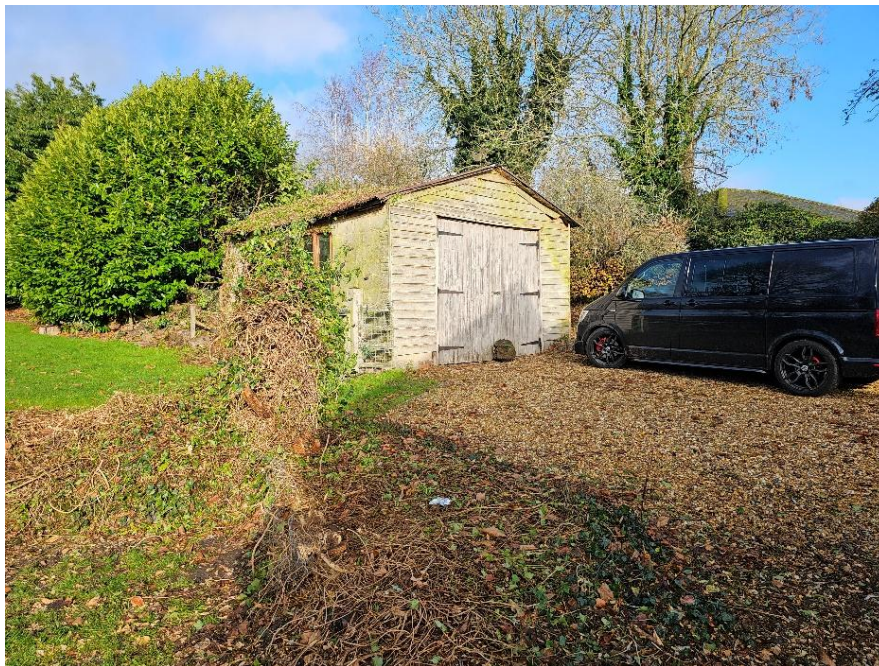
Figure 5 – Front (South) Elevation of the concrete block & timber garage outbuilding
