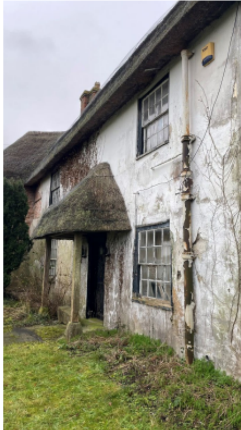
North Elevation windows 13-16
