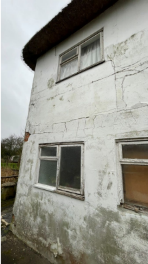
East elevation, Windows 8-10
