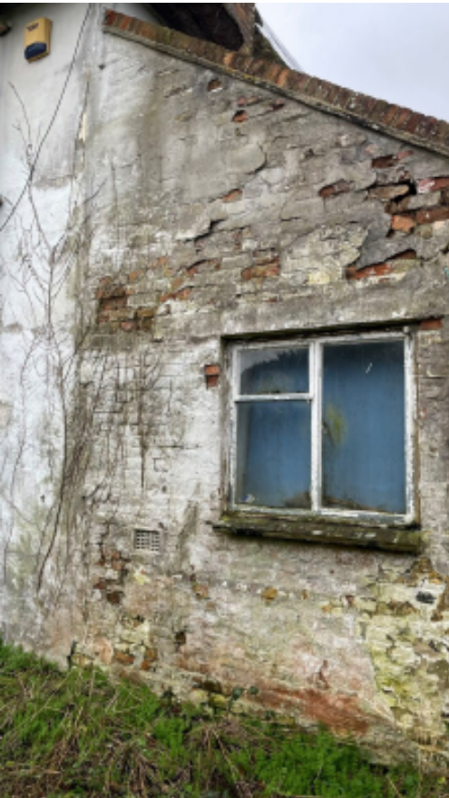
North Elevation window 17
