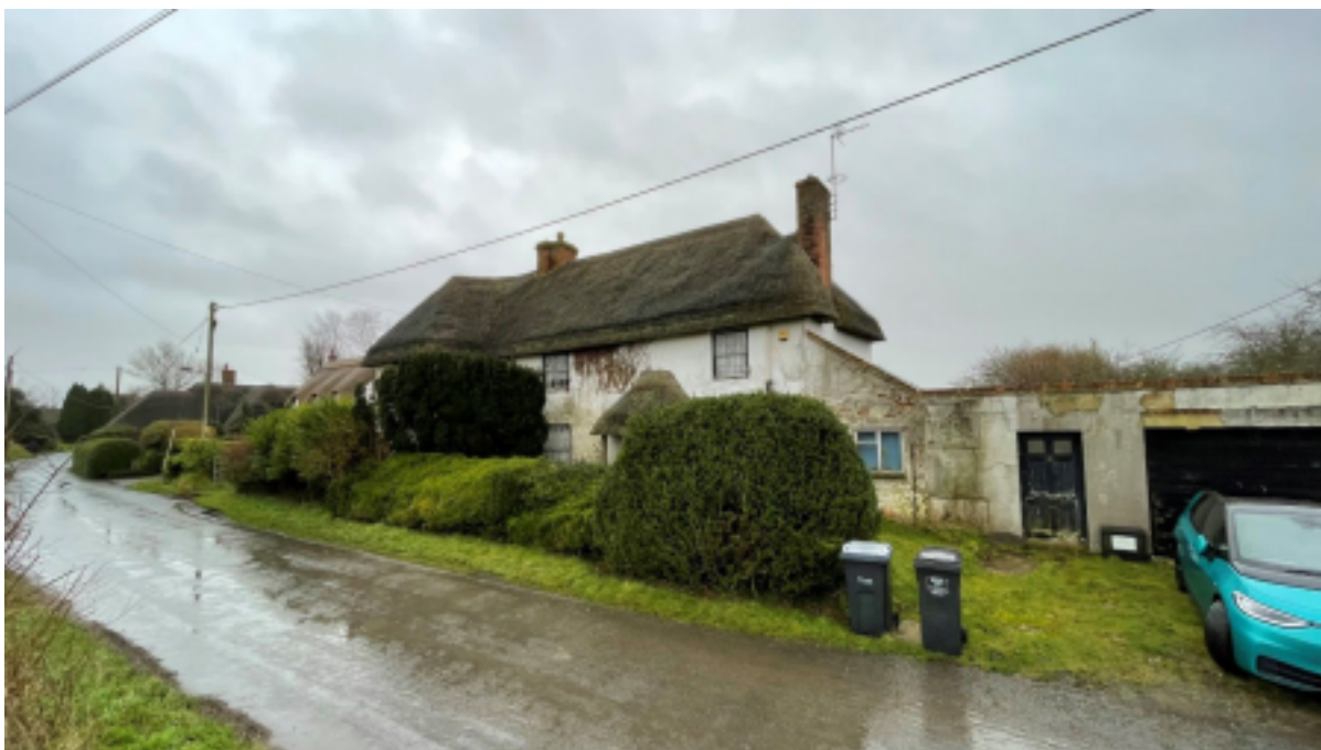
Yew Tree Farm from road to north
