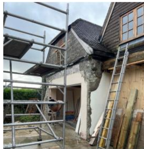
Demolition of link to form two dwellings
