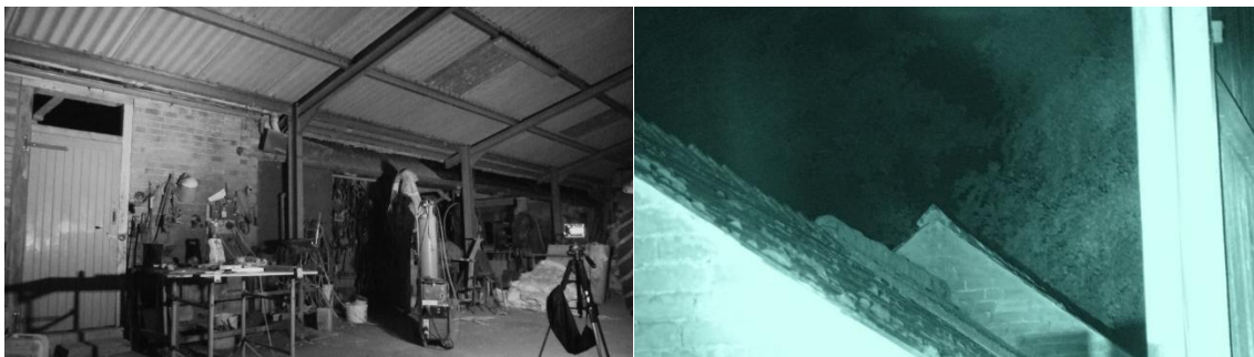
Figure 7 and 8: B6 viewpoint from inside B3 (left) and north (Right)
