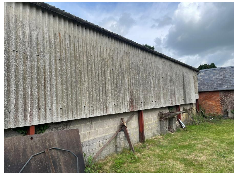
Plate 23: Barn 3's eastern elevation.
