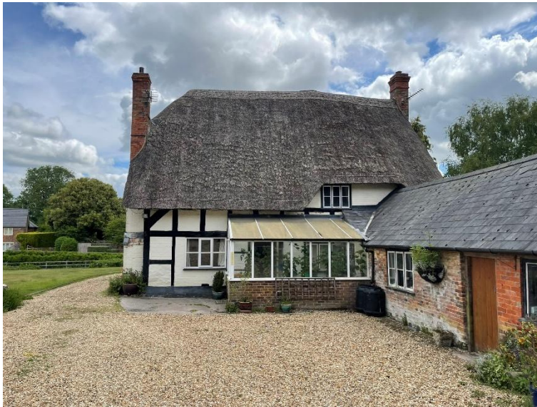
Plate 41: The farmhouse's western elevations.
