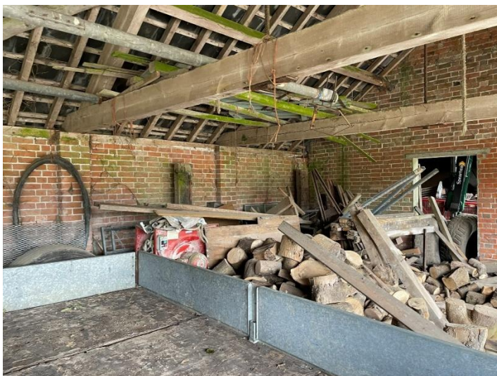
Plate 27: View towards the southern western internal elevation of the barn.
