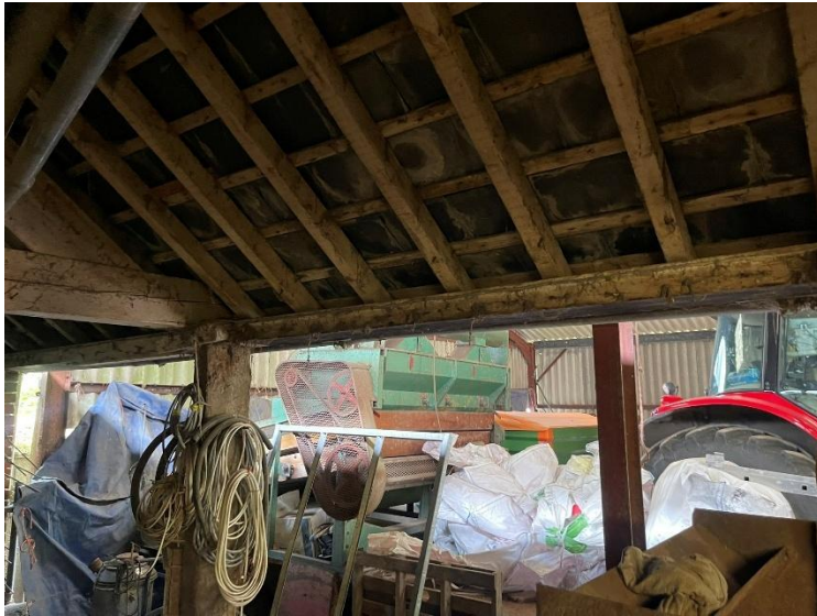
Plate 35: Barn 6's eastern elevation opening.
