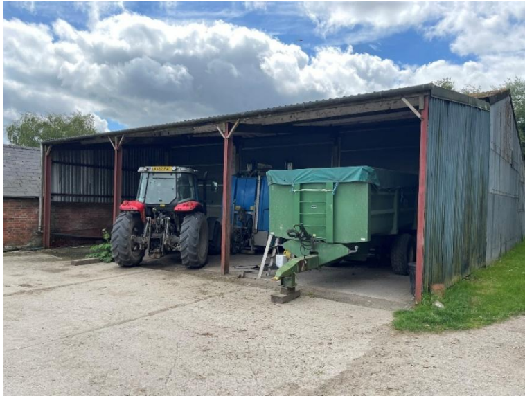
Plate 39: Barn 7's northern elevation.
