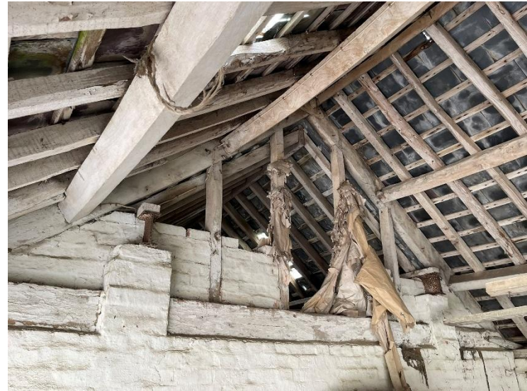
Plate 21: View of the wall opening and roof of Barn 2.
