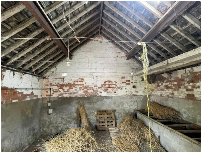
Plate 17: the eastern interior wall of Barn 1.
