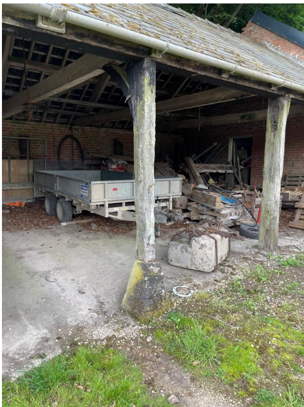
Plate 26: Barn 4, bracketed post supports.
