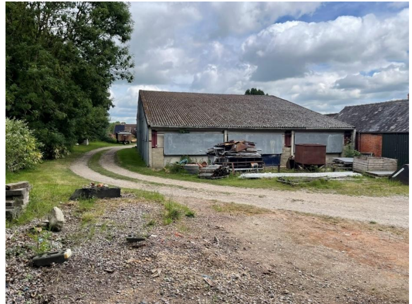
Plate 38: Barn 7's southern elevation.
