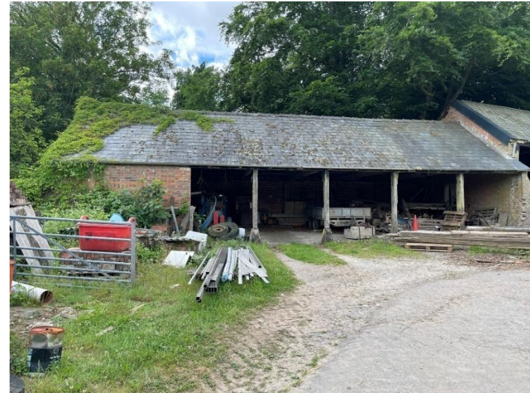
Plate 25: Barn 4's northern elevation.
