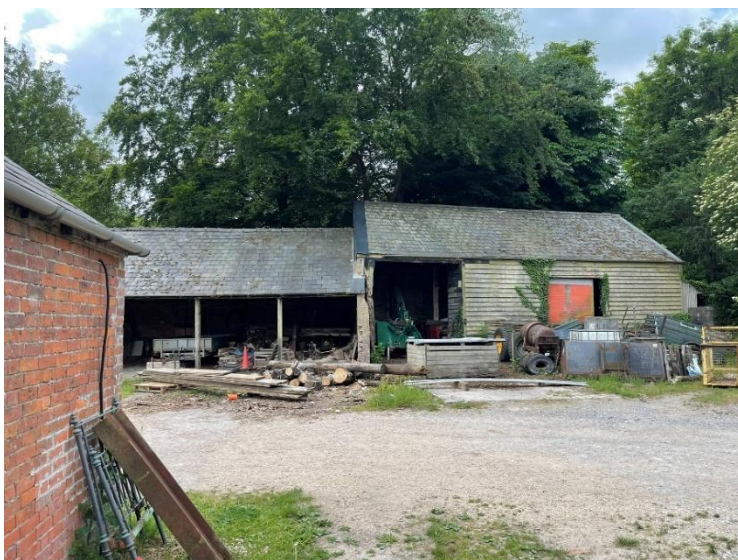
Plate 30: Barn 5's northern elevation.
