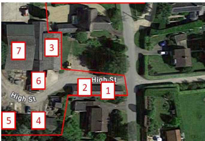
Plate 13: Site layout showing the location of Barn 1.
