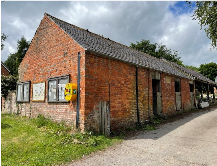
Plate 14: Barn 1, eastern and northern elevations as seen from the High Street.
