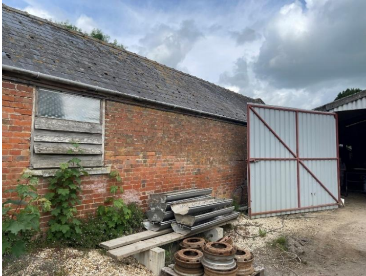
Plate 33: Barn 4's eastern elevation.
