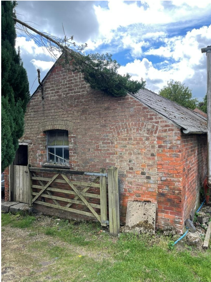
Plate 37: Barn 6's northern elevation, showing segmental arches and brickwork.
