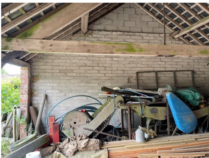
Plate 28: Modern brickwork of Barn 4's eastern wall.
