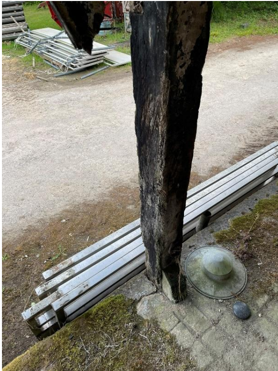
Plate 20: Barn 2, detail of post.
