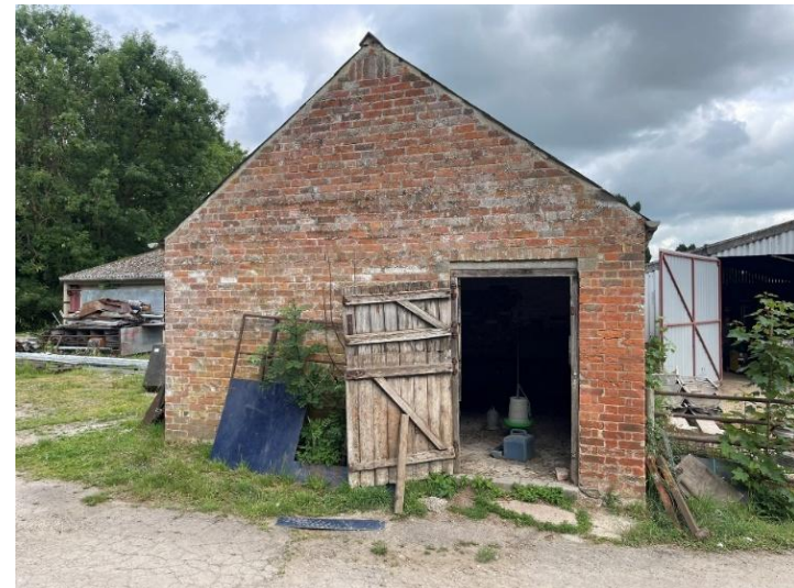
Plate 32: Barn 6's Southern Elevation.
