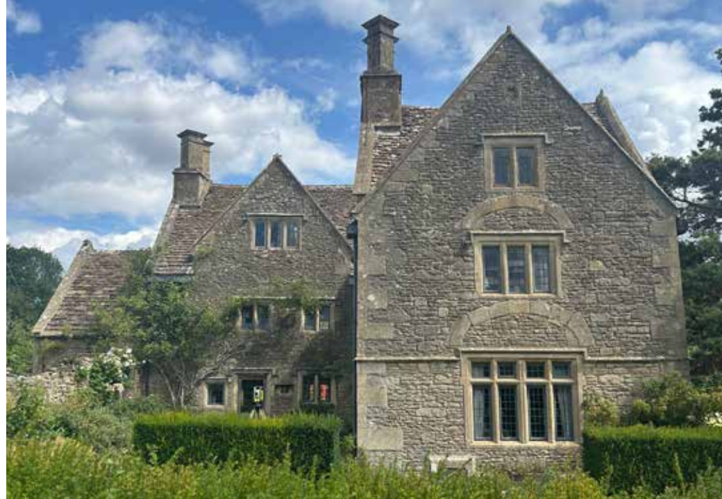
South-West elevation of the Main House
