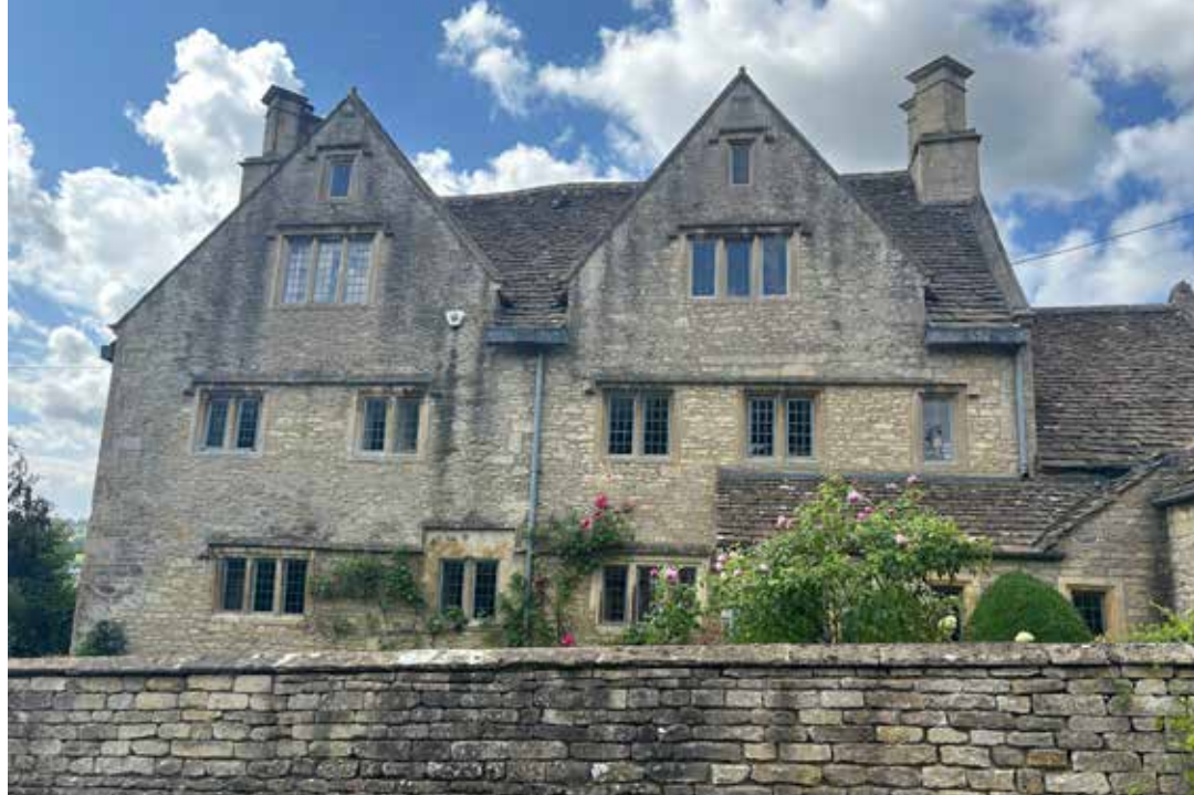
North-East Elevation of the Main House, facing the main road.
