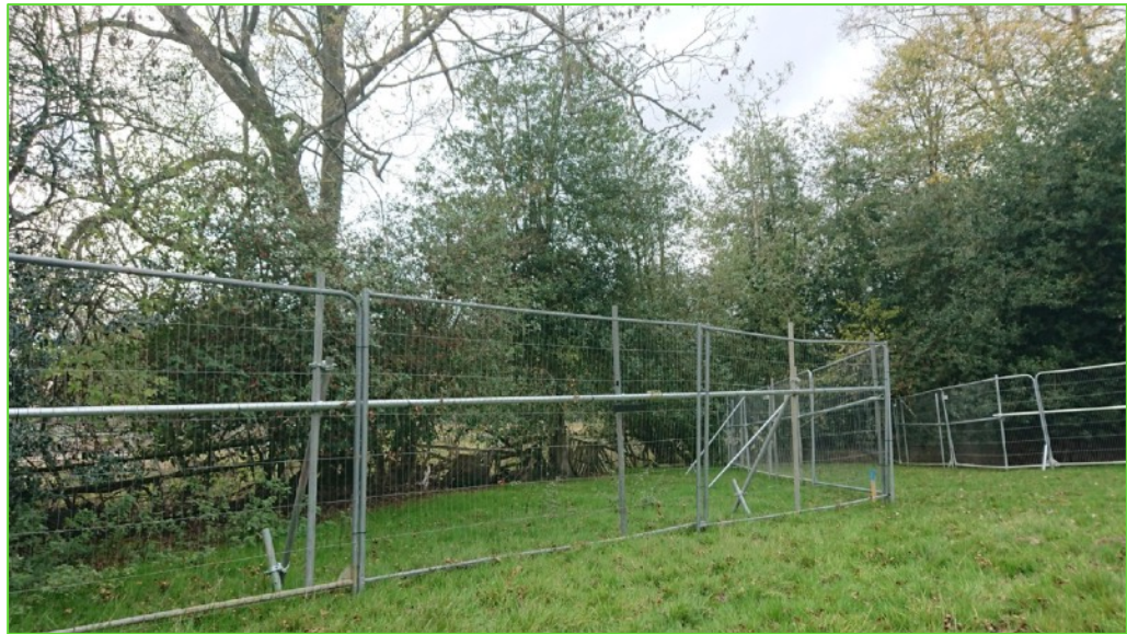
Typical tree protection barrier construction
