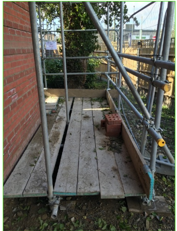
Scaffold ground protection
