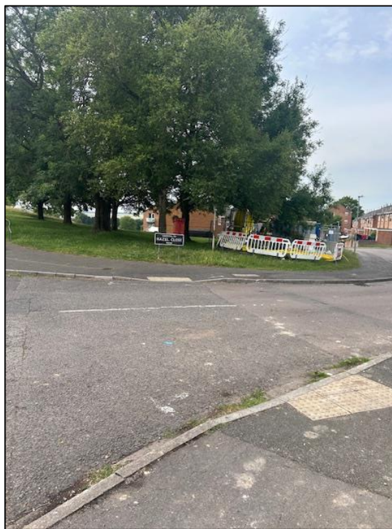
Photograph 4: Uncontrolled Crossing at Hazel Close
