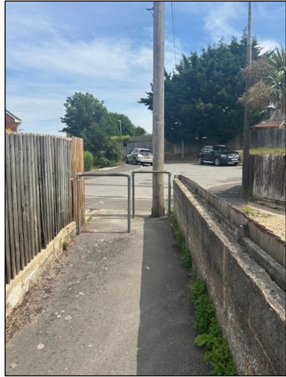
Photograph 11: Guard Railing at Cheshire Close – SALS37
