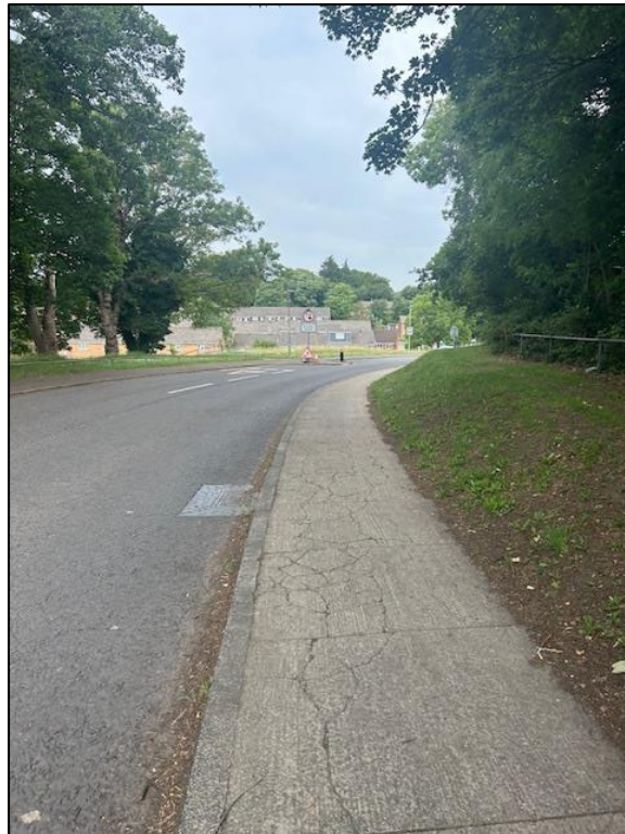
Photograph 3: Westwood Road Footway
