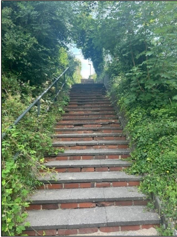
Photograph 10: Stairs at PRoW SALS37
