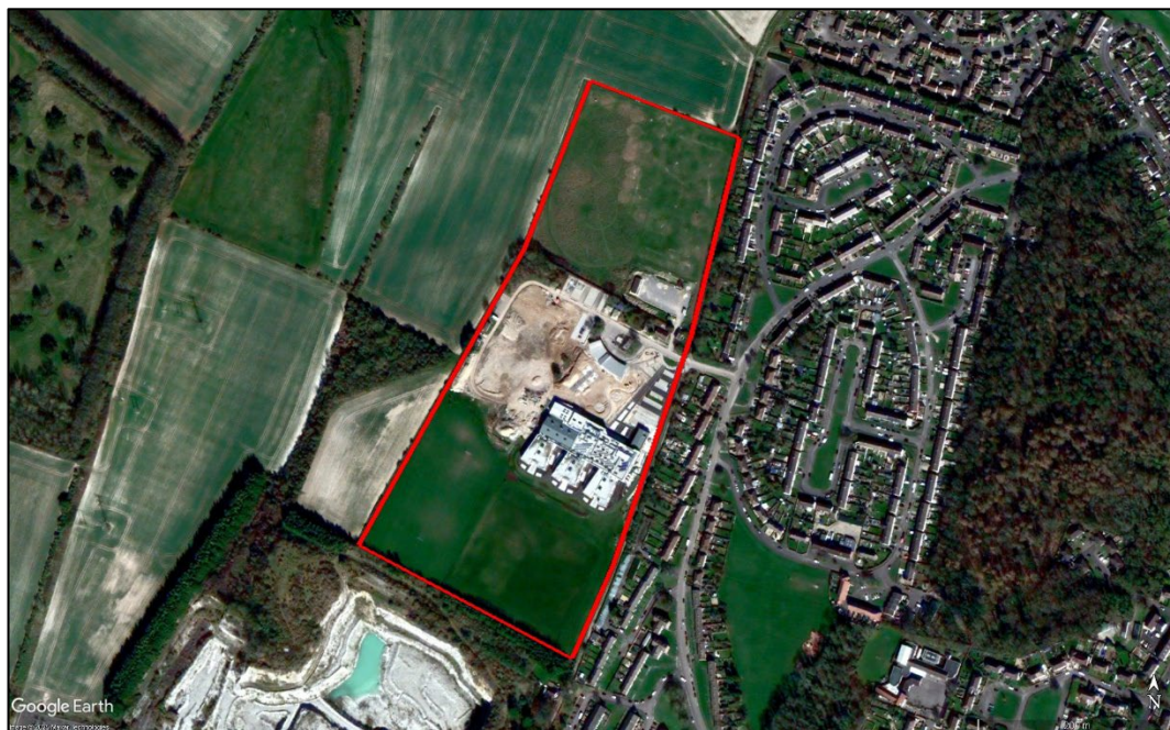
Fig. 8: Aerial image of the Site in 2014, showing the extent of the construction works
