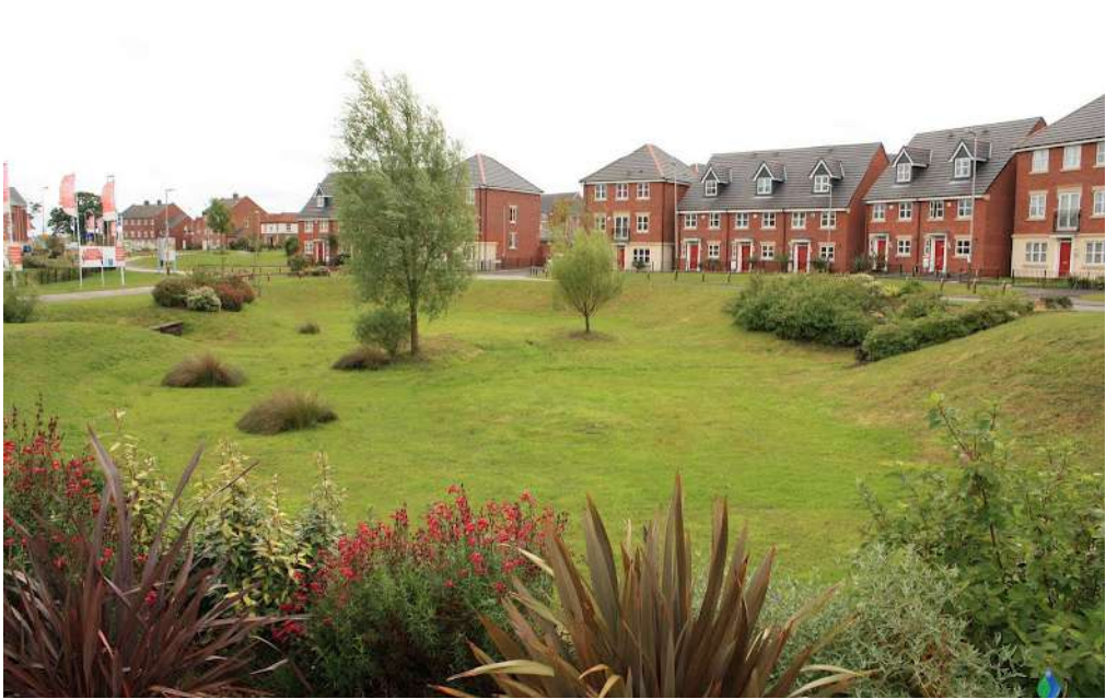
Dry Sustainable Drainage System storage basin
