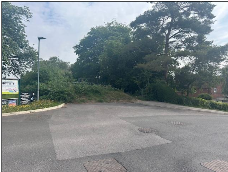
Photograph 1: Persimmon Homes Residential Development Future Access
