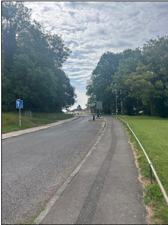
Photograph 4: Traffic Calming Build-out on Westwood Road
