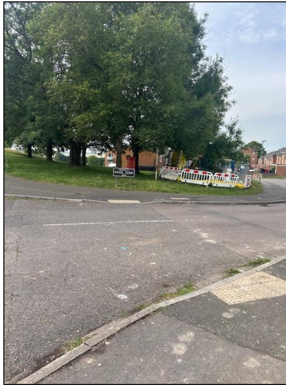
Photograph 3: Uncontrolled Crossing at Hazel Close
