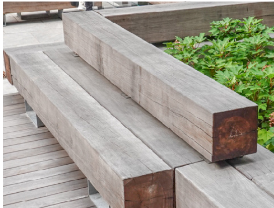
B1 - Two Level Stepped Sleeper Seating Description: Seating area around outdoor classroom space and used throughout courtyard. Colour/Finish: Upcycled Hardwood FSC
