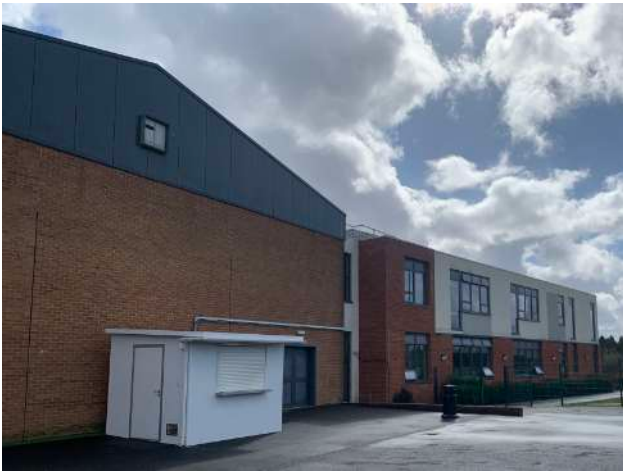
West elevation of the existing school and sports hall, highlighting a mix of both brown and red brick.
