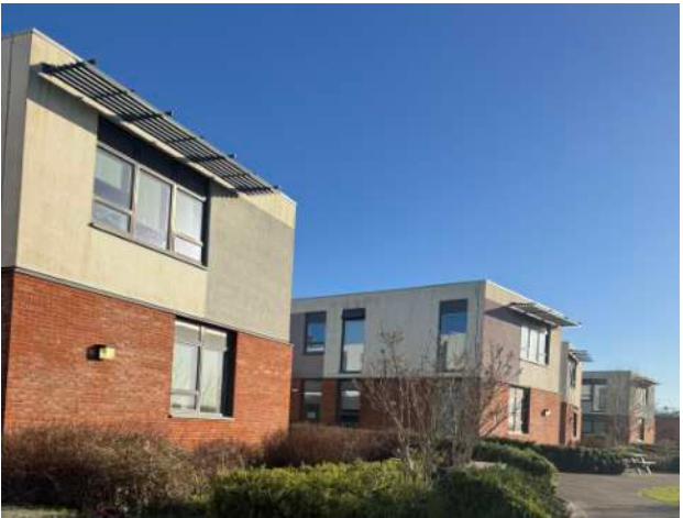
South elevation of the existing 'petals,' with a red facing brick at ground floor.
