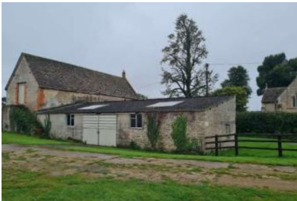
Figure 3: Image of Tithe Barn and Church from application site.
