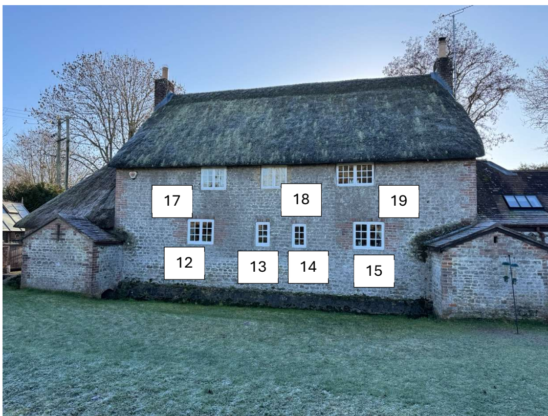
Rear (North) Elevation Left
