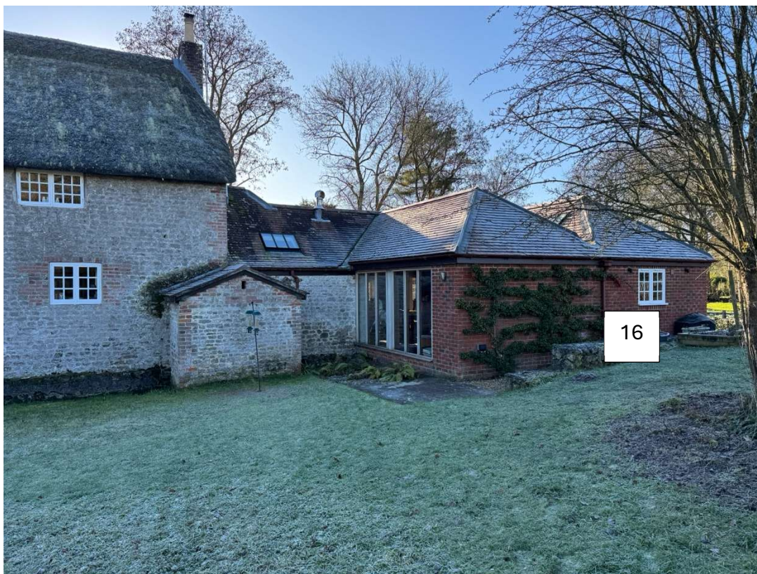
Rear (North) Elevation Right
