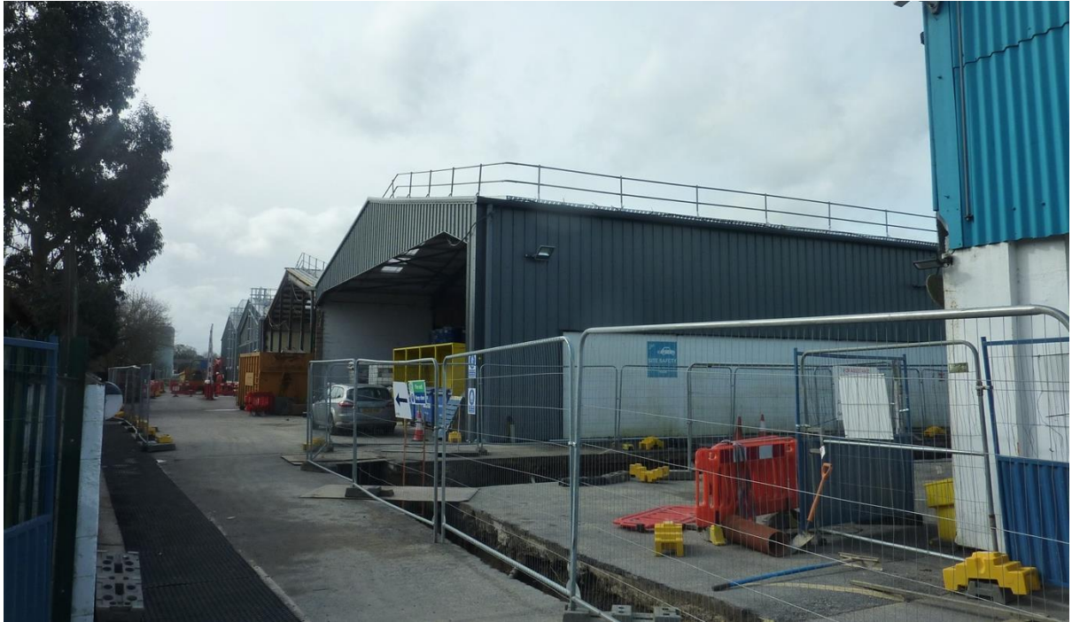
Figure 3 – Example of building with new Merlin Grey cladding
