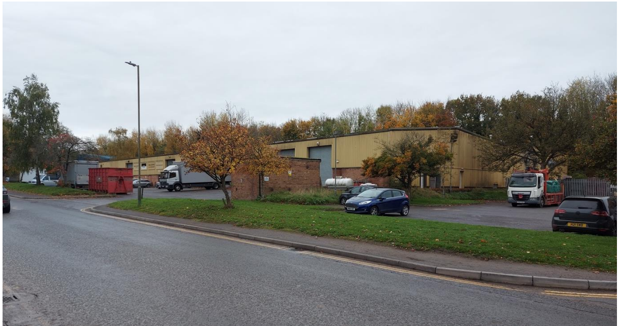
Figure 2 –Existing cladding on the application building
