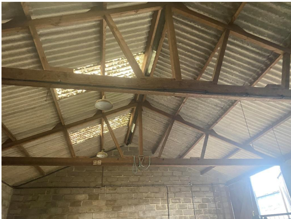
Plate 3: Interior view of main barn
