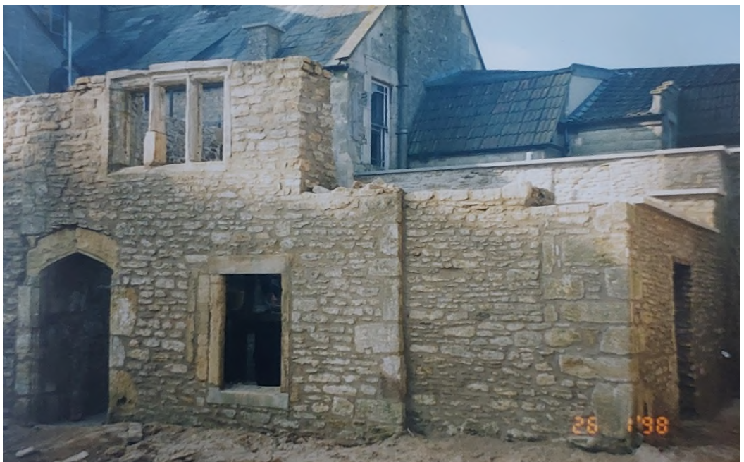
Figure 6 The front elevation of the former farmhouse during reconstruction in 1998.
