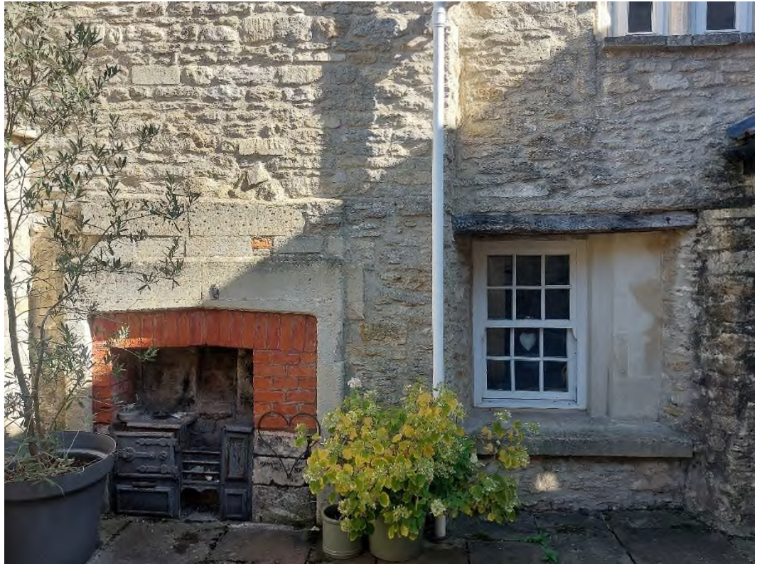
Figure 11 The west, formerly internal face of the northern part of the original front elevation which now faces into a small, enclosed yard area.
