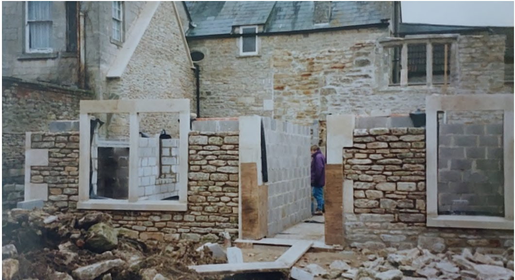
Figure 7 The new house set in front of the former front elevation of the farmhouse under construction in c.1998.
