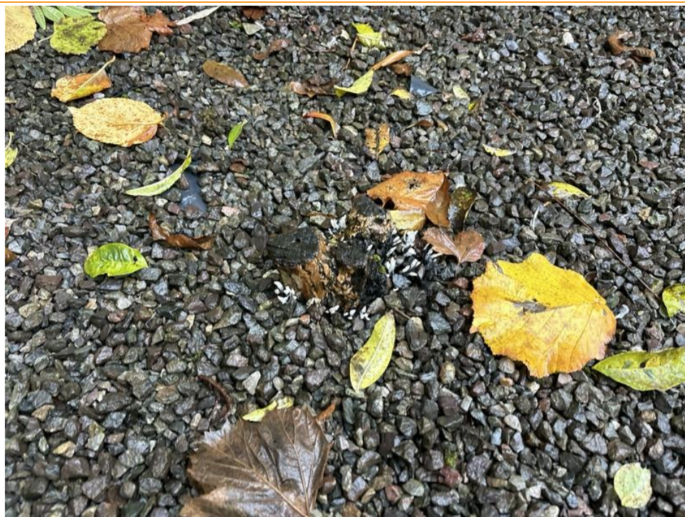
Small old, decayed stumps to front of property.
