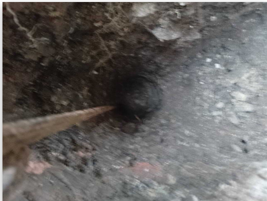
Fig 1.1: Trial Hole 1 Location
