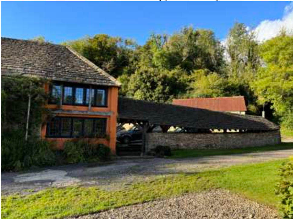
Image 1.8 – Oak framed structure and infill building [in lime render] built in 2017/8
