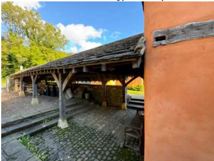
Image 1.9 – Oak framed structure and infill building [in lime render] built in 2017/8
