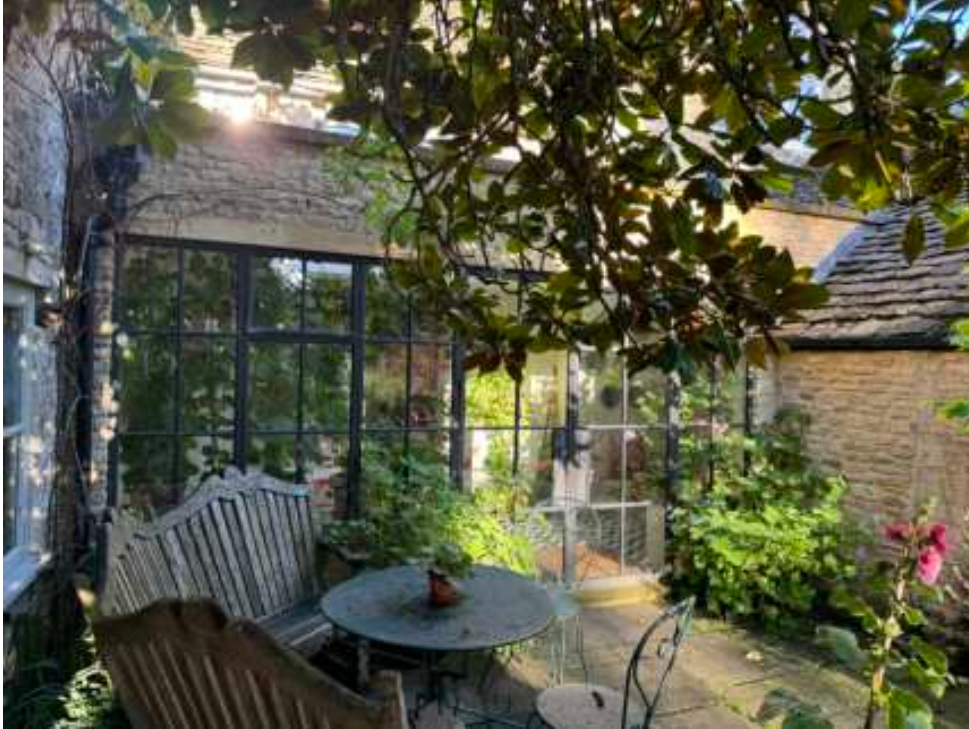
Image 1.8 – Oak framed structure and infill building [in lime render] built in 2017/8
