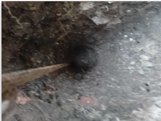
Fig 1.1: Trial Hole 1 Location
